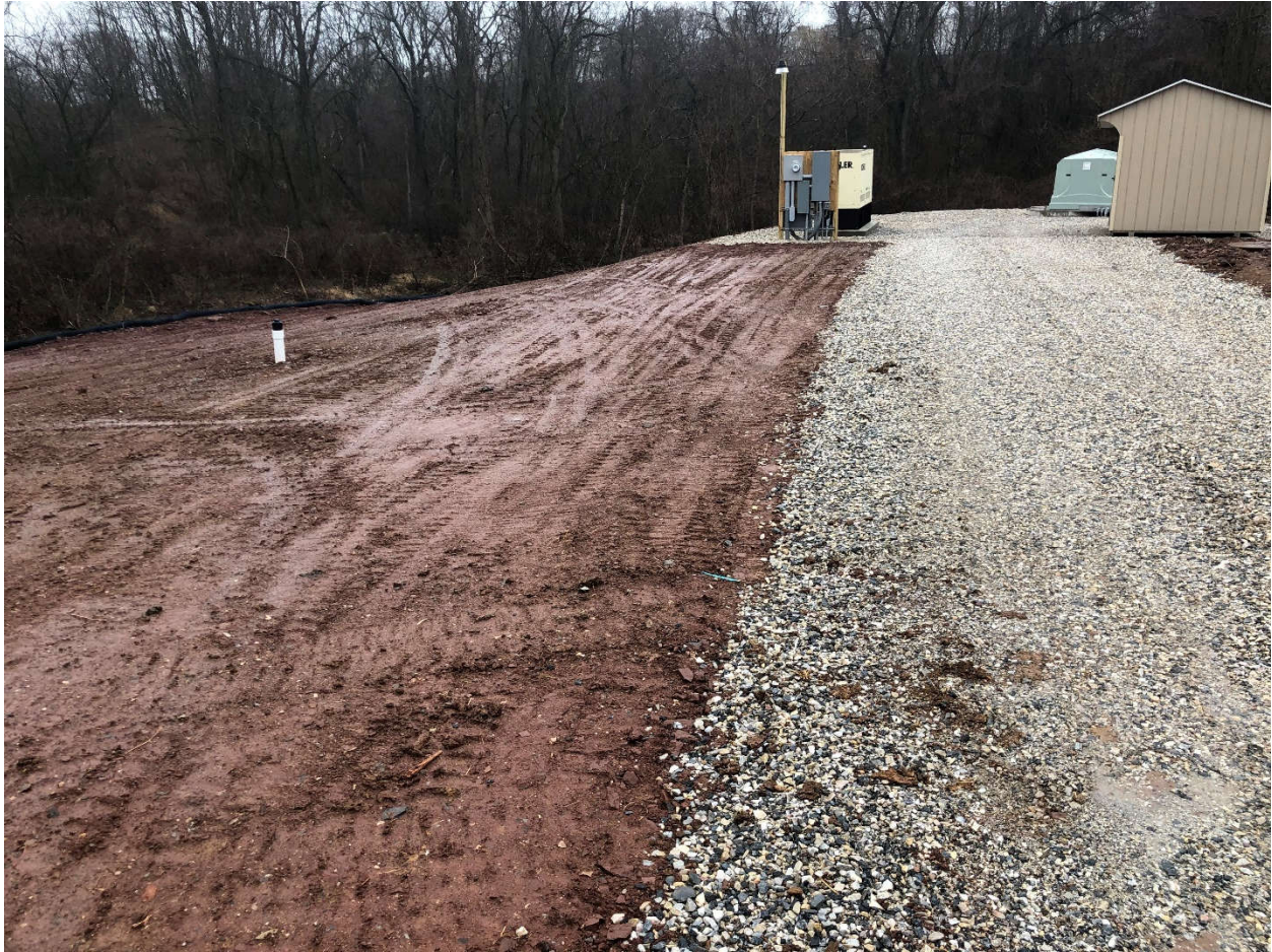
Location of Former Wastewater Treatment Facility (New Pumping Station and Generator Shown in Background) Date of Photo: February 10, 2020
