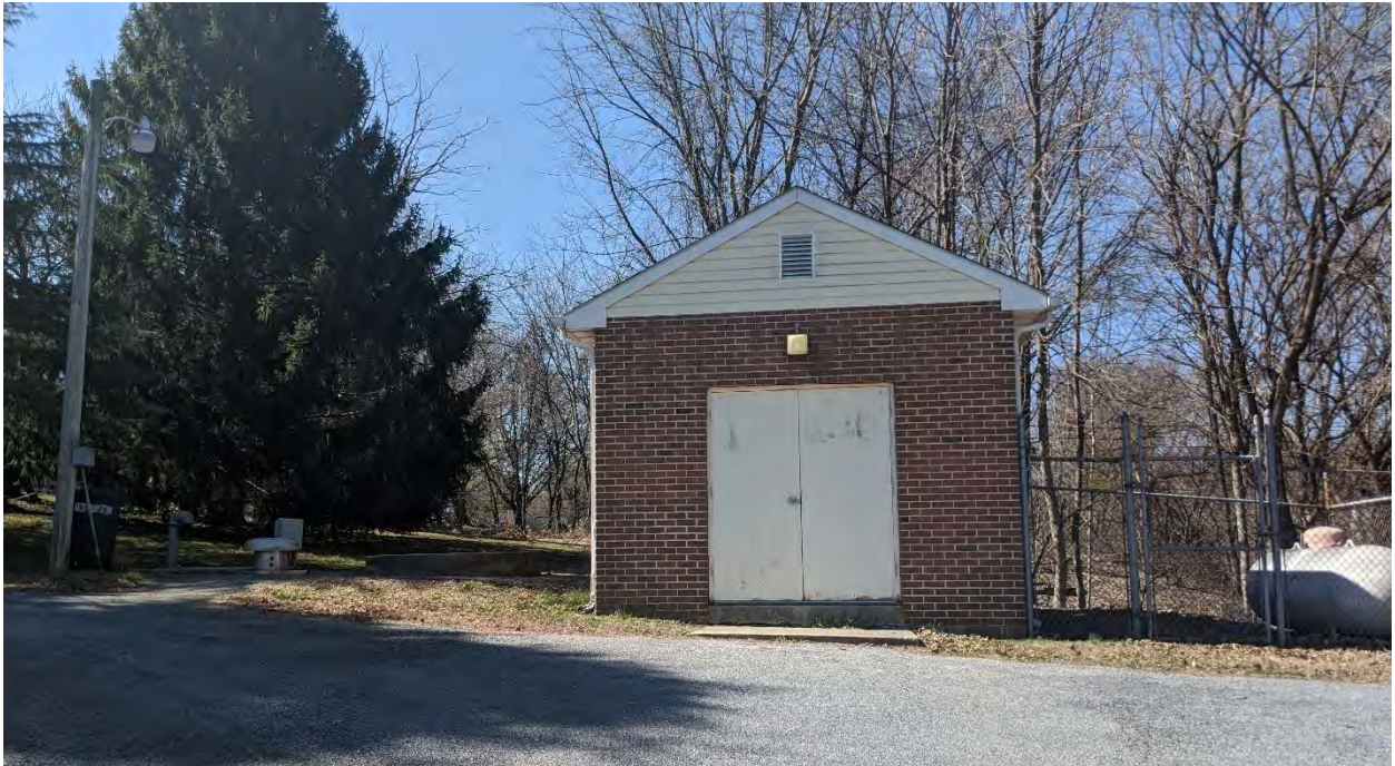
Country Ridge Pump Station
