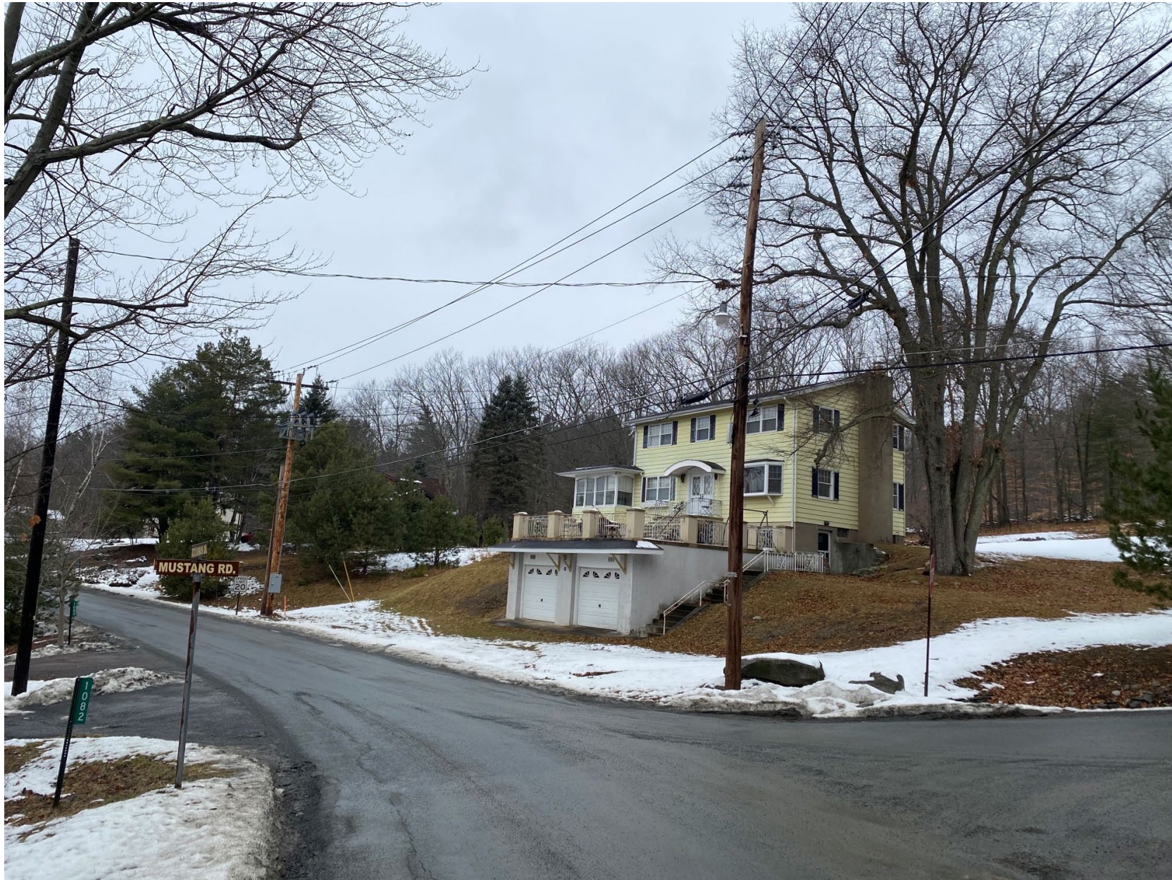
View of 1079 Aquarius Dr, taken from south of intersection of Aquarius Dr and Mustang Rd
