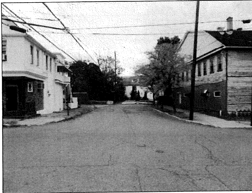
View of the near advance intersection. Note the missing advance "Bridge Closed" signs.
