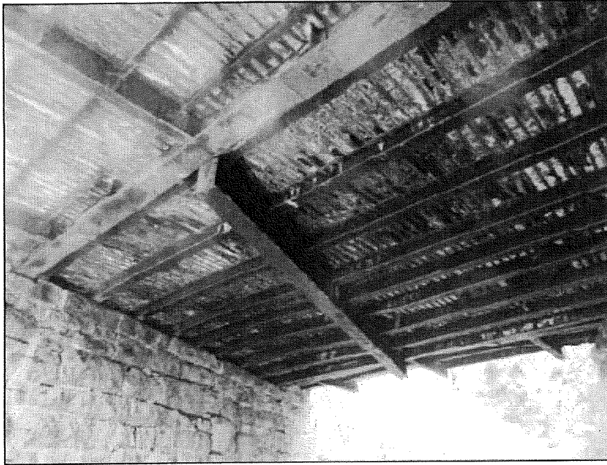
View of the left floorbeam and girder connection.
