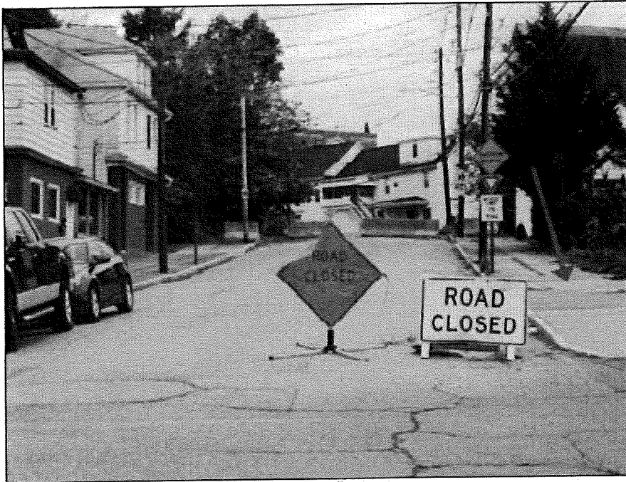
View of the far advance intersection. Note the missing advance "Bridge Closed" signs.
