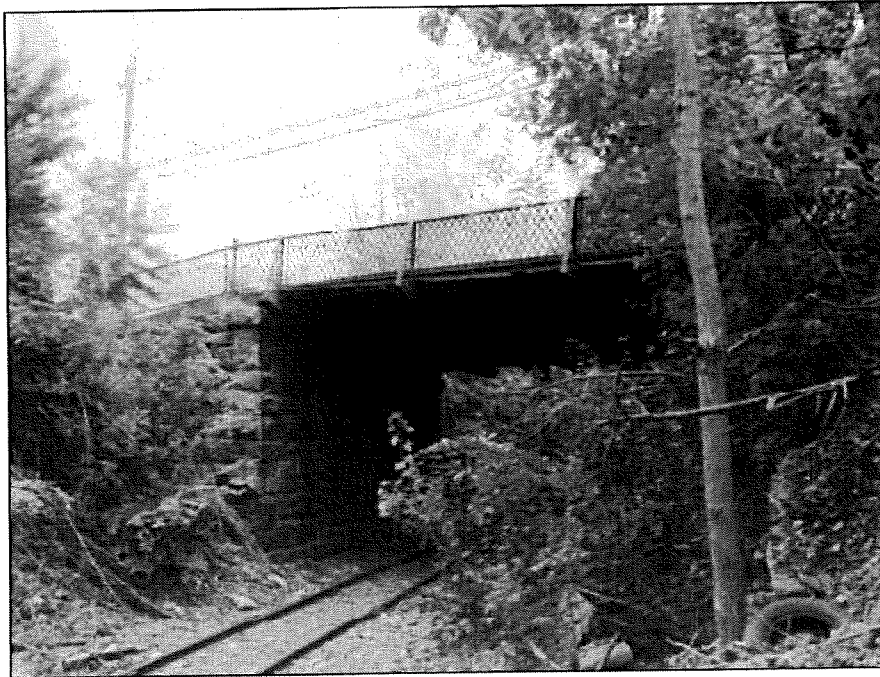
Elevation view, looking from the left.
