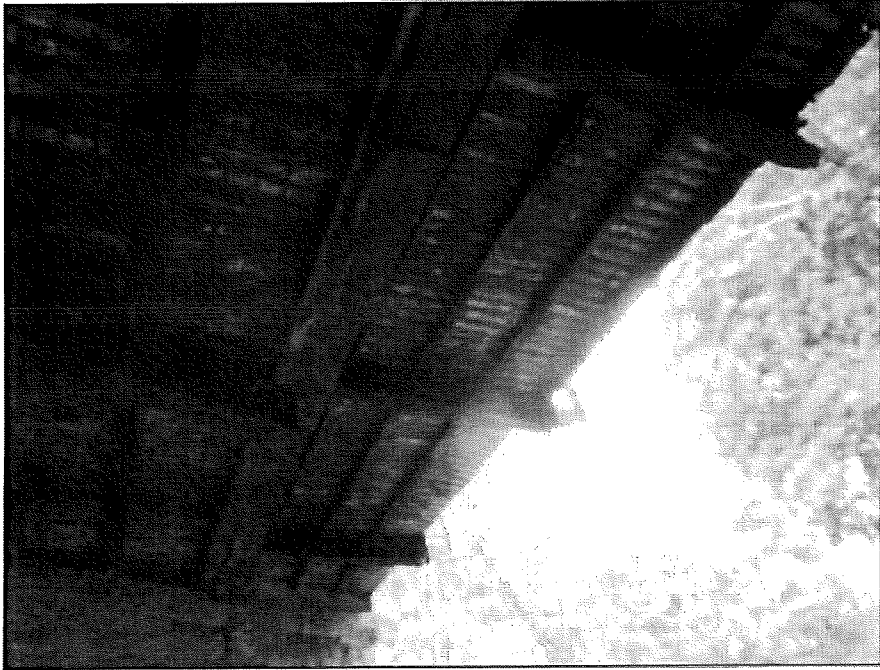
View of the underside of the right sidewalk.
