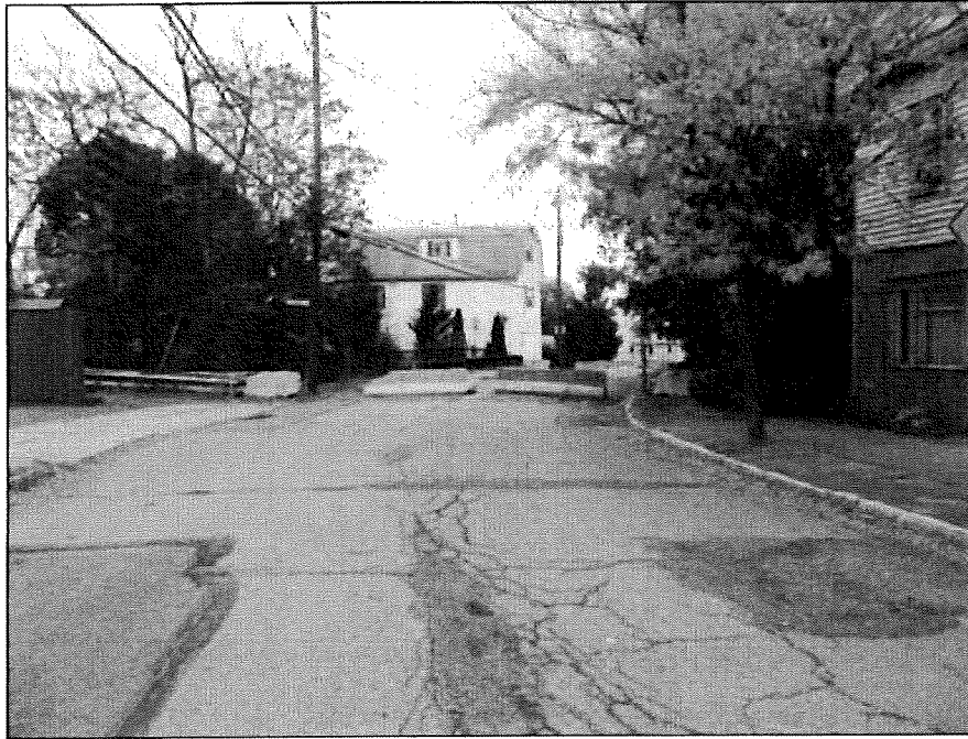
The approach roadway, looking from the near side. Note the missing "Bridge Closed" sign.
