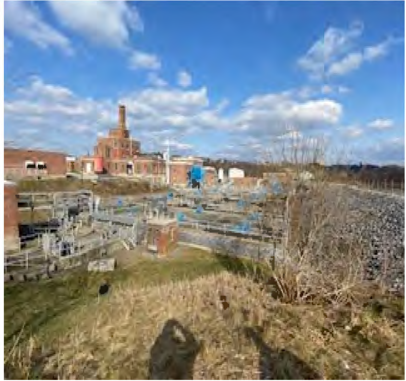
A/O Tanks (RNR System)
