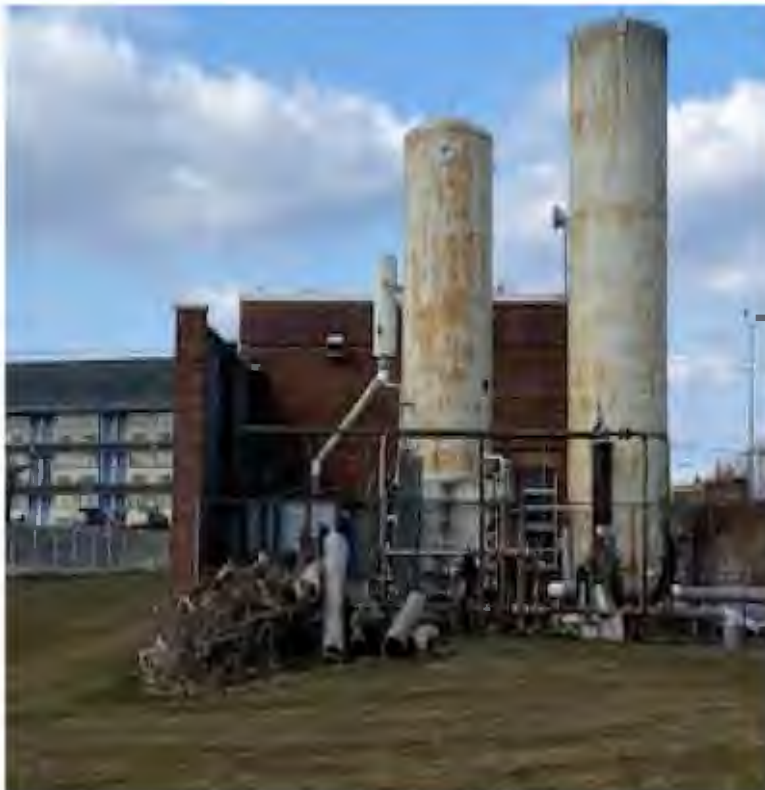
Old Compressor Building
