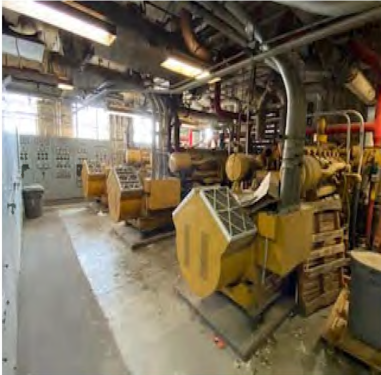
CAT Engines (Out of service)
