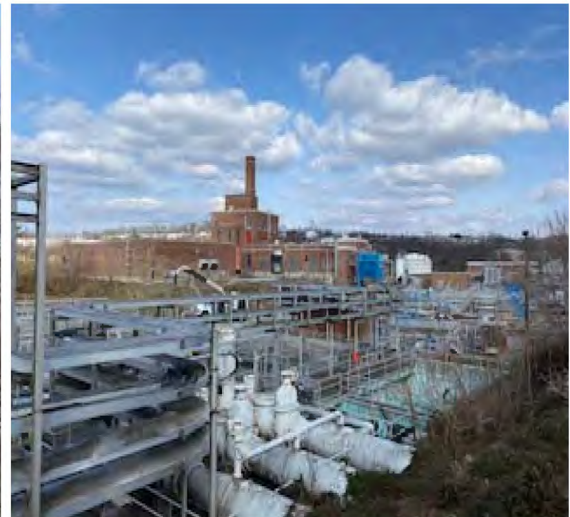
Complex/Control Room and Training in background.
