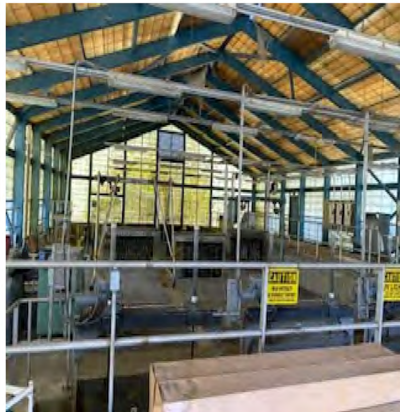
Ultra-Violet Disinfection Building
