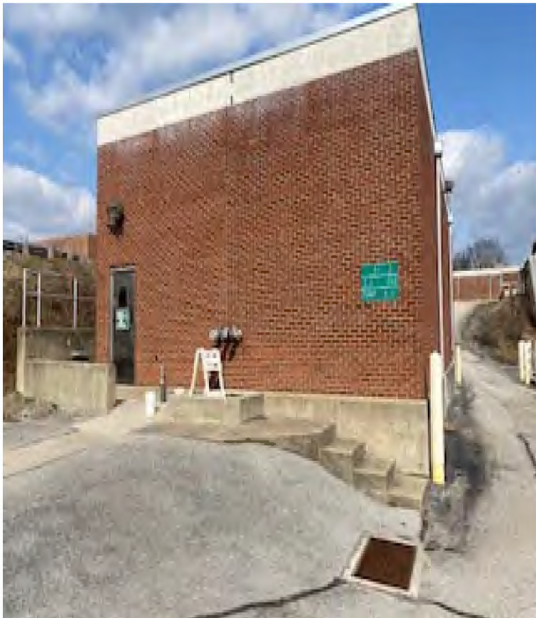
Sludge Pump Building
