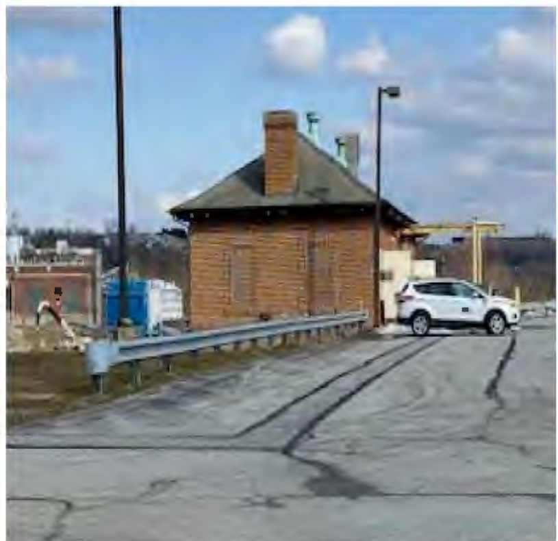
Primary Sludge Pumping Station
