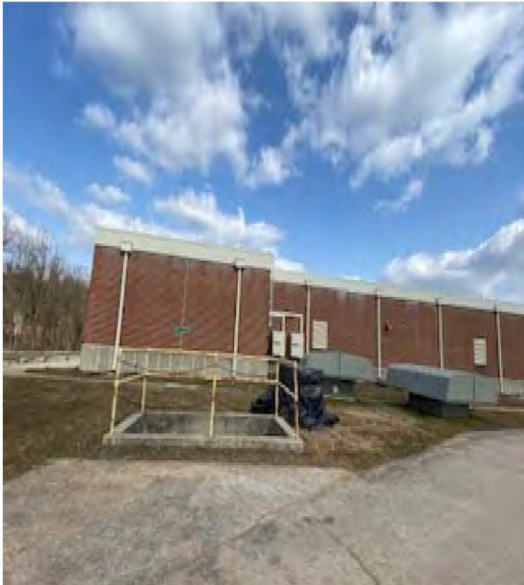
Filter Building (Diamond Filters)
