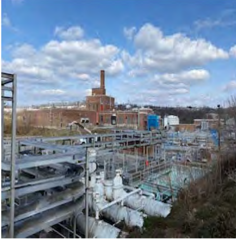
Storm Water out flow and A/O Tanks are in the foreground.
