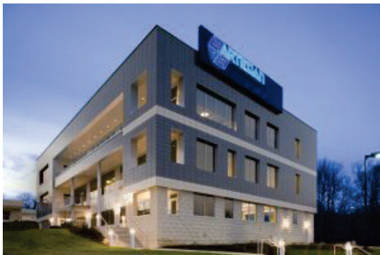
Artesian Water Co. has acquired the Frankford municipal water system in a $3.6 million deal. | PHOTO COURTESY OF ARTESIAN
