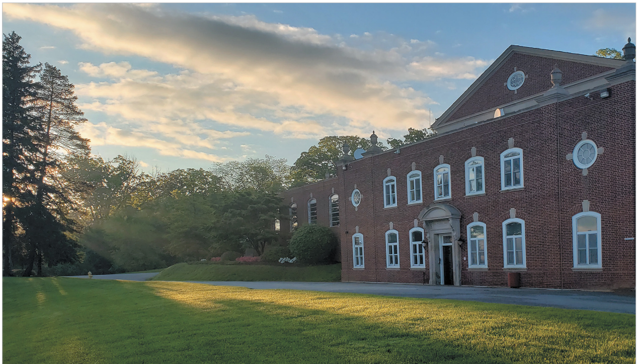
Our Filter Plant, located in Reservoir Park, was built in 1930 in order to meet the water needs of the growing community. This facility was initially built with a capacity of 15 million gallons per day, but has since expanded to 40 million gallons per day. This facility is still in service today, and purifies and distributes water to our customers every single day.
