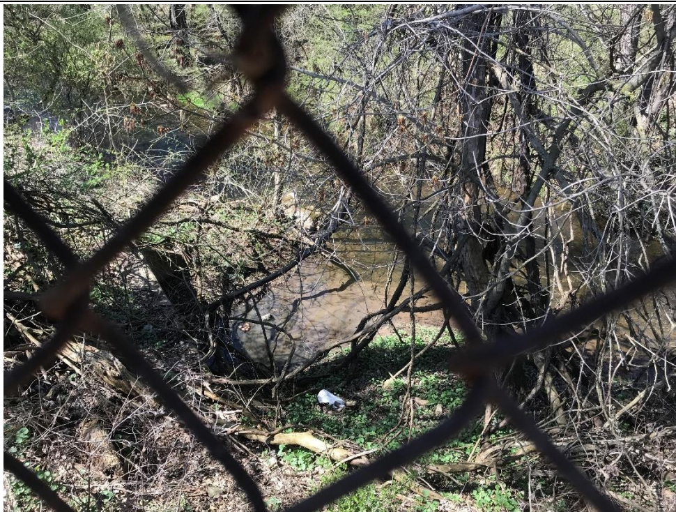
Photo 3. Outfall 006 where discharge of wastewater occurred. Sewage odor present. Photo taken by Ashley Chong.
