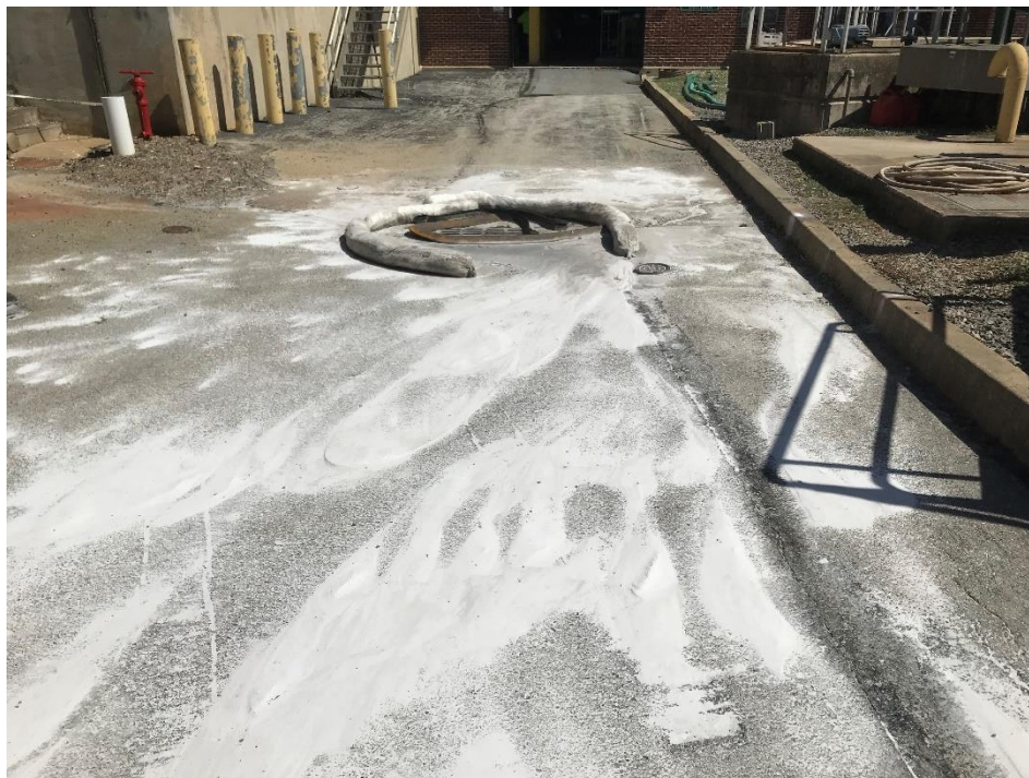
Photo 8. Catch basin which wastewater had entered next to Digester #1. Photo taken by Ashley Chong.
