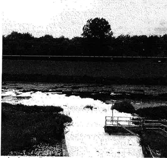
Photo taken by Austen Randecker - Outfall 002 effluent cascade on 08/14/2019
