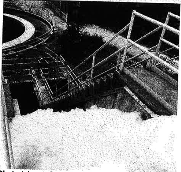
Photo taken by Austen Randecker – Train 2 screw pumps with foaming 08/14/2019
