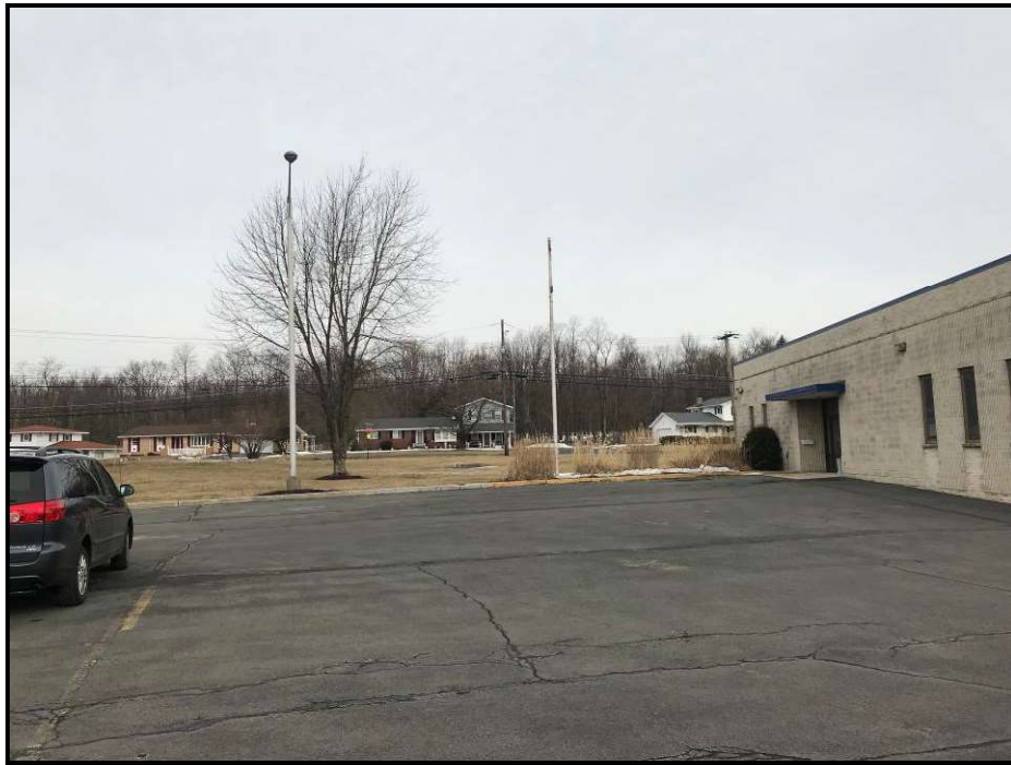
Flagpole and pole mounted lighting
