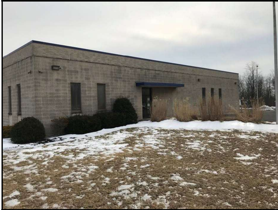
North side of the office building
