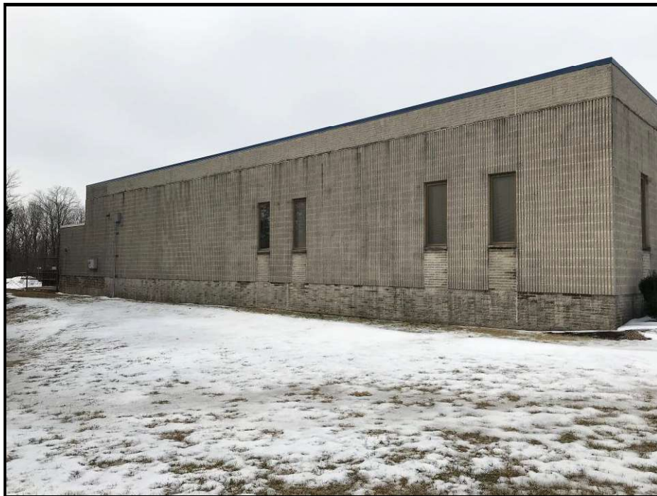
East side of the office building
