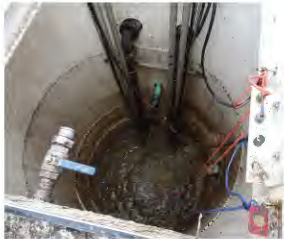
Figure 4 – Pump Station Wetwell
