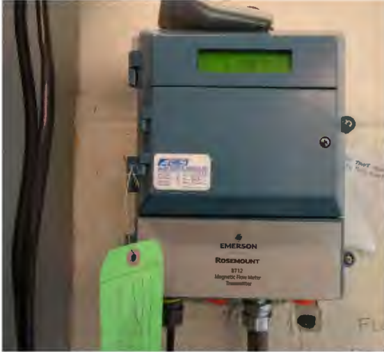
Figure 9 – Flowmeter readout
