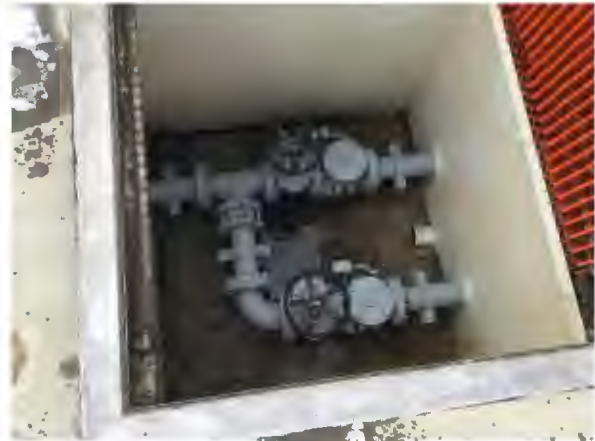
Figure 6 – Valve Chamber
