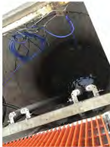
Figure 2 – Pump Station Wetwell
