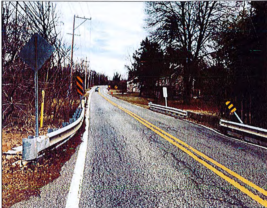
Photograph 1. View of Swedesford Road facing east
