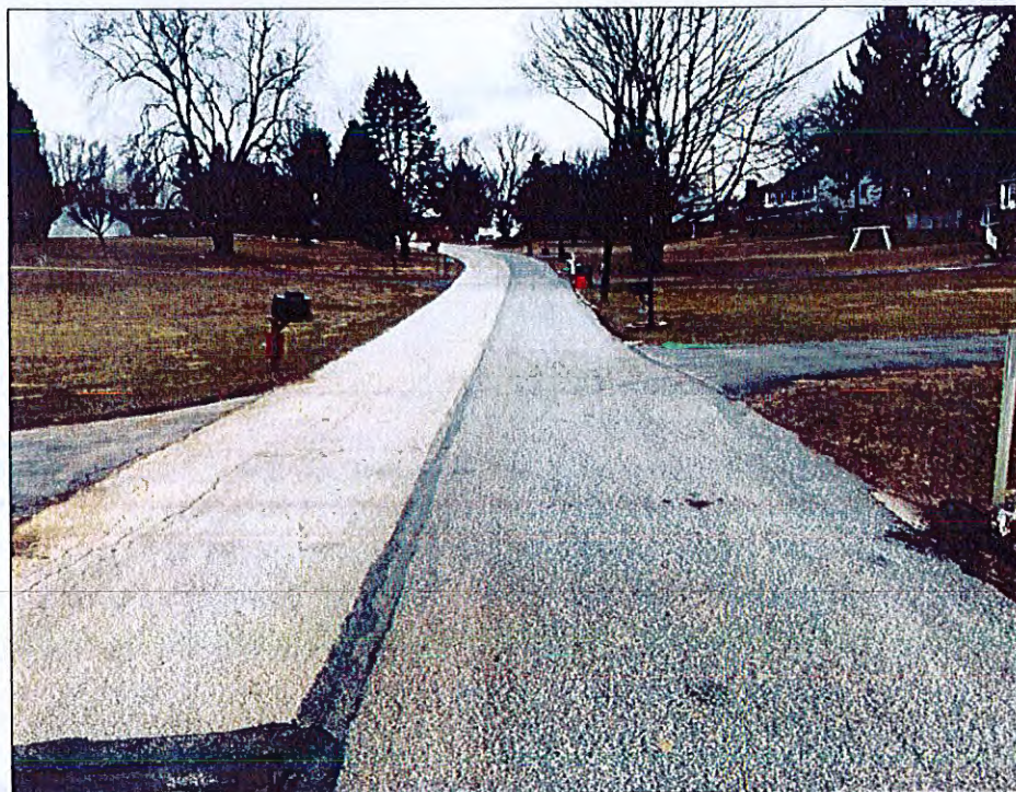
Photograph 4. View of Elk Drive facing west.
