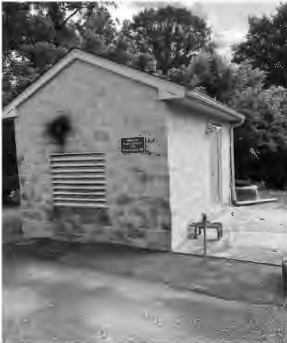
Hillbrook Circle Pump Station - P.S. 11
