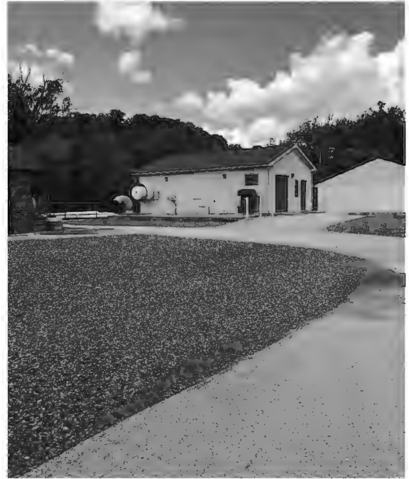
Mill Lane Pump Station - P.S. 2
