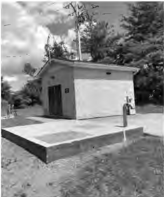
Wilburdale Pump Station - P.S. 3
