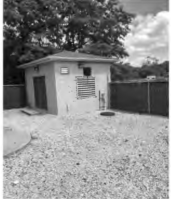
Lee Boulevard Pump Station - P.S. 4
