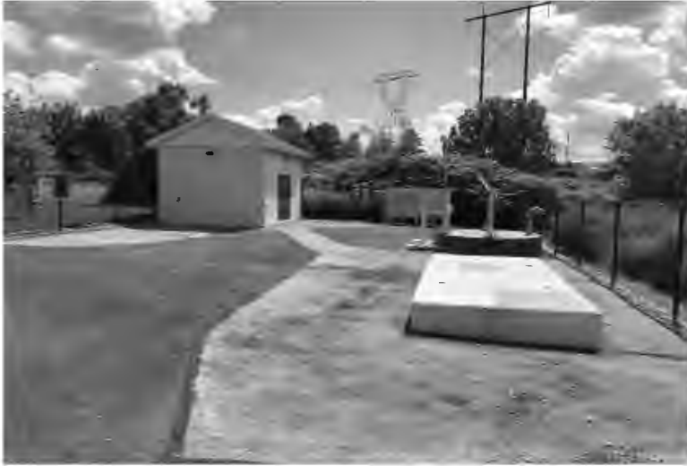
Planebrook Road Pump Station - P.S. 14
