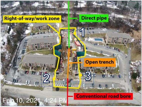
To bring the pipeline across Glen Riddle Road onto the Property, SPLP is using conventional boring, a technique typically used for road crossings, in which pits are excavated at either side of the road, a boring machine is lowered into the pit at one end and bores underneath the road to the other side, and then pipe is installed. That area of work, which is depicted in red on the photograph, is already completed.
