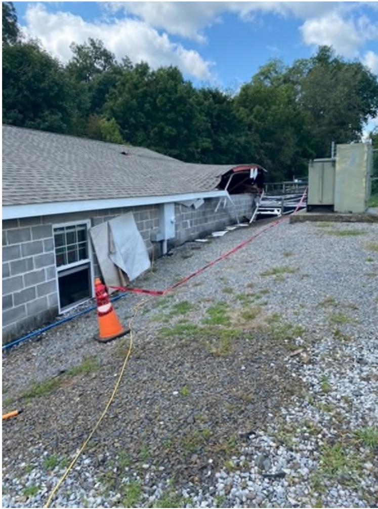
**CONTROL BUILDING ROOF DAMAGE DUE TO THE FLOATING OF THE RAPID SAND FILTER TANK / ULTRAVIOLET DISINFECTION SYSTEM IN ABOUT HALF OF THE BUILDING.**
