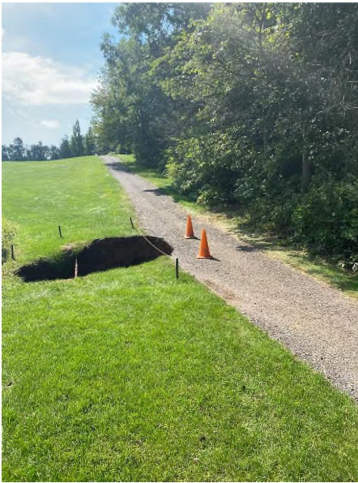
**SINKHOLE LOCATION ON GOLF COURSE PROPERTY OVER TOP OF CULVERT. NHSC PROPERTY LINE AT WOODS/FENCE LINE TO THE RIGHT. EARTH WASHED INTO THE COLLAPSED CULVERT SUBSTANTIALY BLOCKING IT.**
