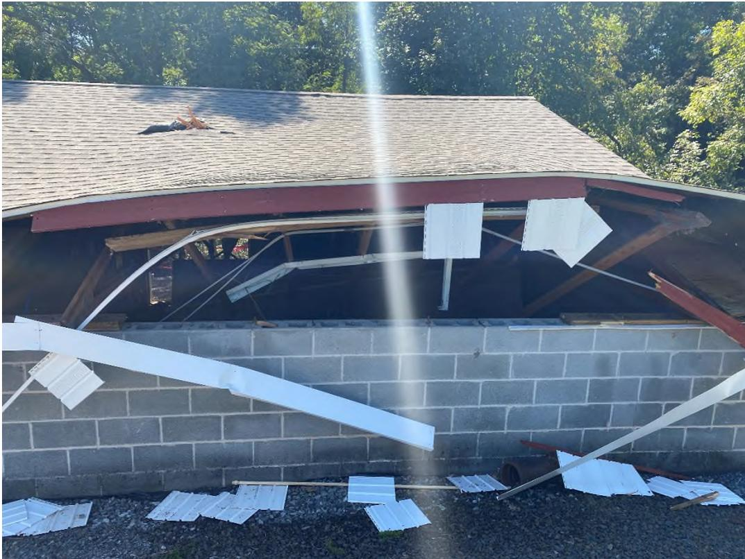
**RAISED UP ROOF TRUSSES AND ROOF RESULTANT FROM TANK FLOATING IN THE CONTROL BUILDING.**
