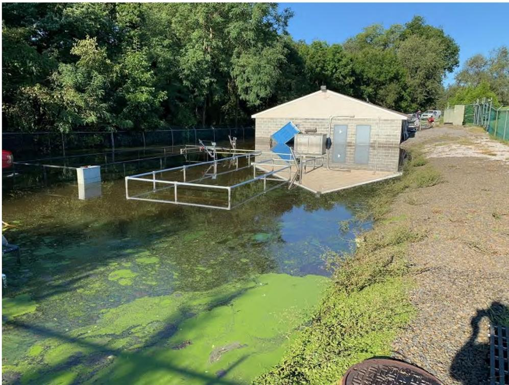
**SUBMERGED WASTEWATER TREATMENT PLANT VIEW FROM EAST SIDE OF PLANT LOOKING WEST. RAILINGS ON EQ AND SLUDGE HOLDING TANKS CAN BE SEEN. GENERATOR IS TO THE LEFT OF CONTROL BUILDING DOOR.**
