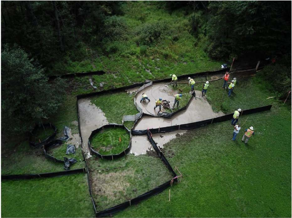
Photo by Austin Richardson, EI with Tetra Tech on August 25, 2018
