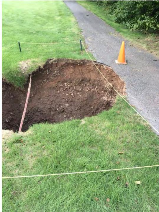
Figure 1- photo taken by Kevin Buss, shows sink hole at the site of the culvert failure.
