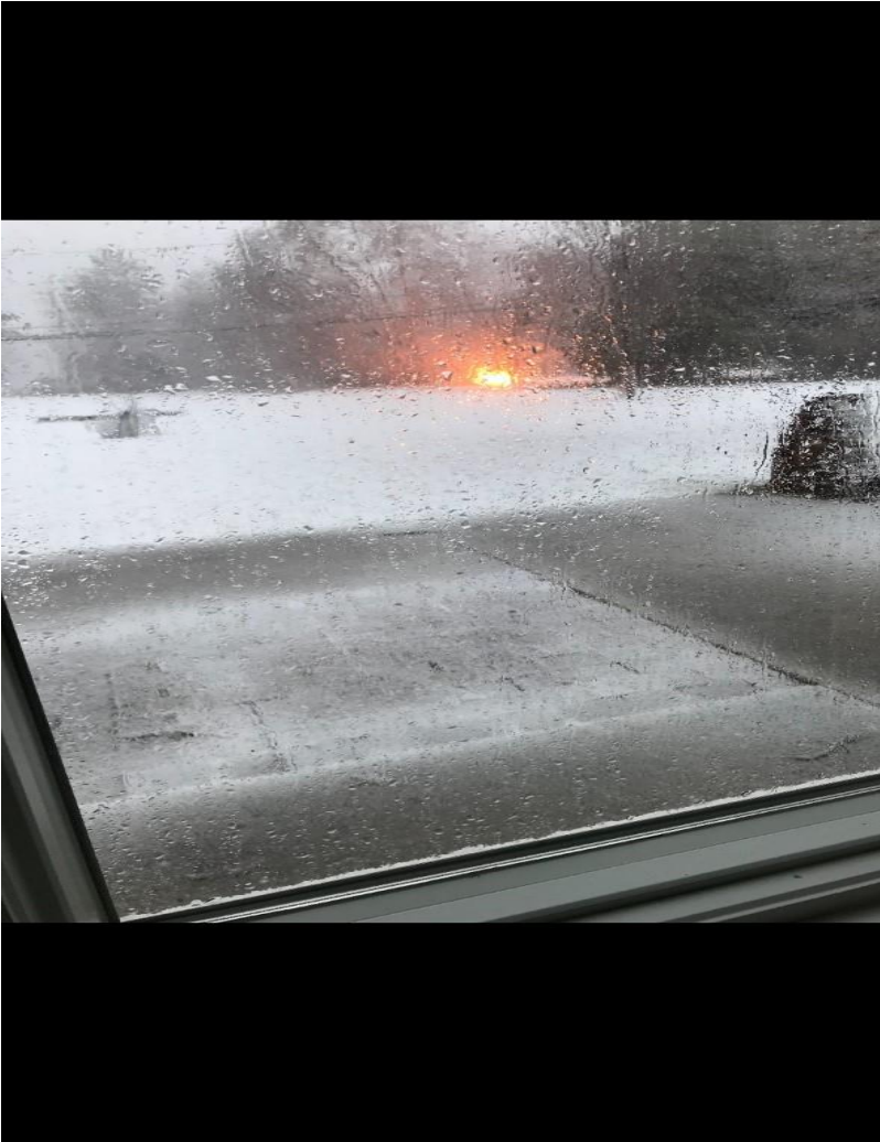
Exhibit 3 Electrical Fire in Backyard
