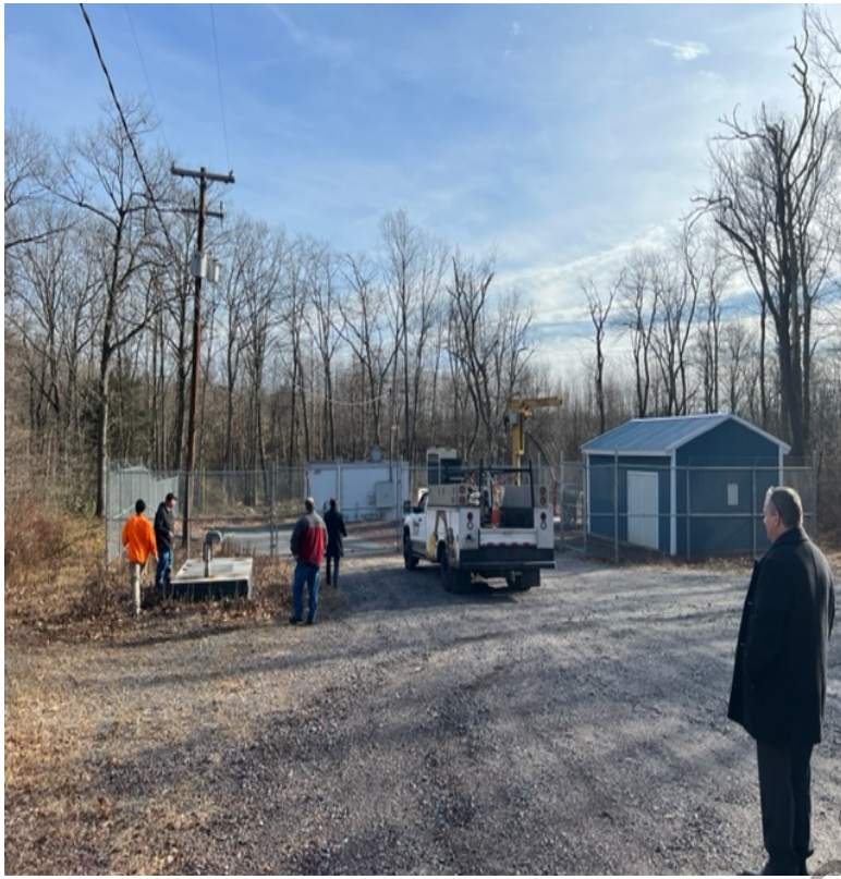
Woodside pump station
