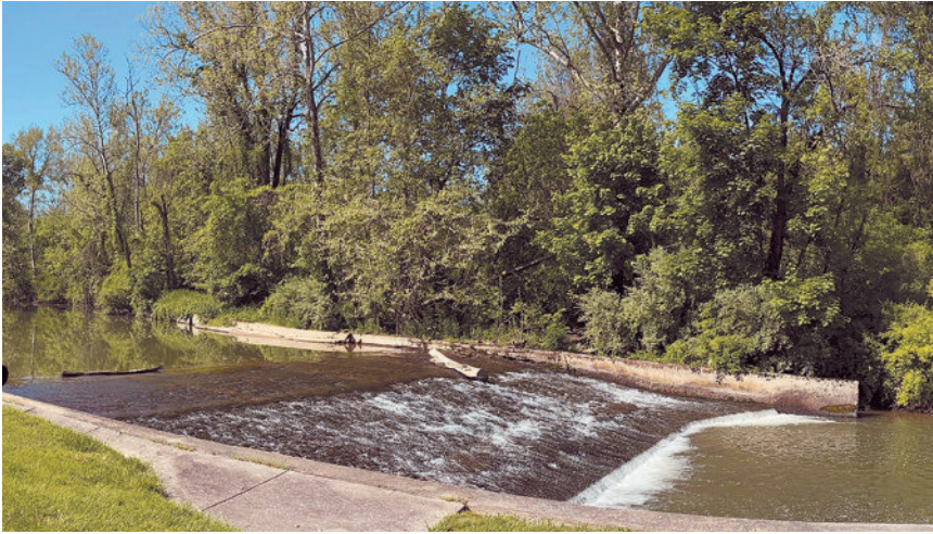
The South Branch of the Codorus Creek runs behind Brillhart Pumping Station, which has been transferring water to our Filter Plant for over 125 years.
