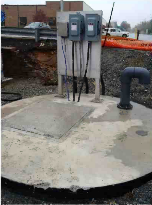
Figure 1 – Wet Well Exterior
