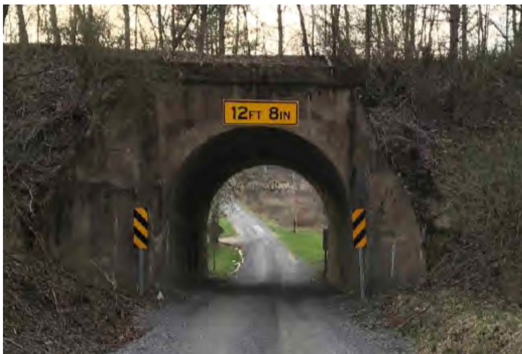
East Bellport Road wing walls westbound
