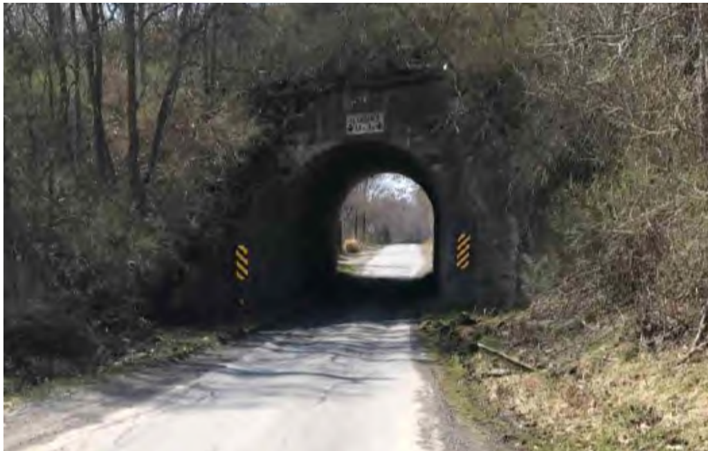
Ramsaytown Road wing walls westbound
