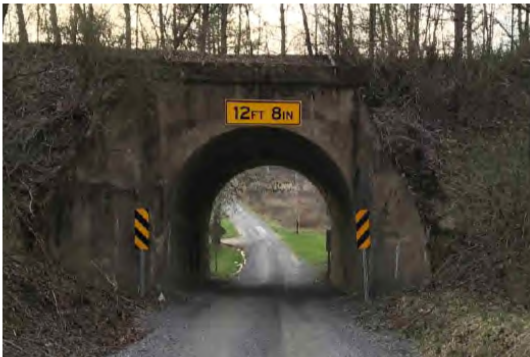
East Bellport Road wing walls westbound
