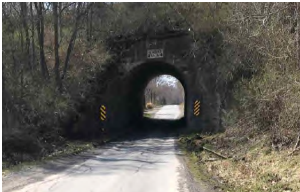
Ramsaytown Road wing walls westbound
