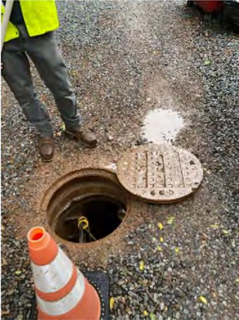
6-27-22 - Manhole to which the ultraviolet disinfection system effluent discharge pipe is connected. Note the adjacent puddle in this low spot. TSS may be introduced at this location. Plastic manhole insert to be installed to prevent introduction of TSS at this location.
