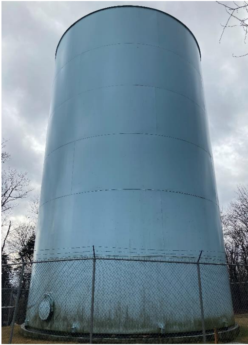
Figure 1 – Tank looking South
