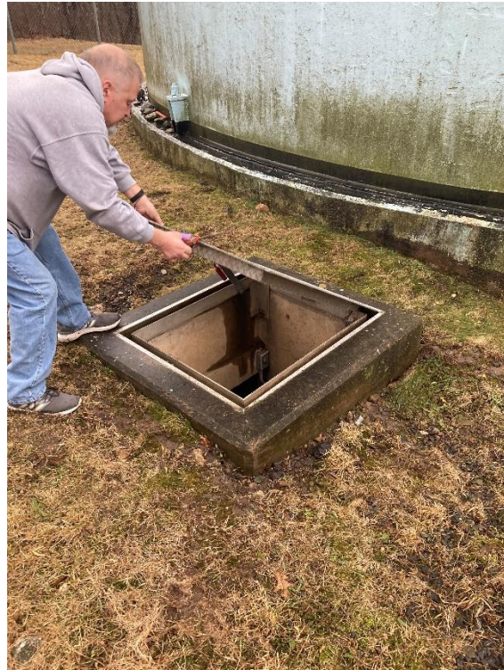
Figure 2 – Valve Vault
