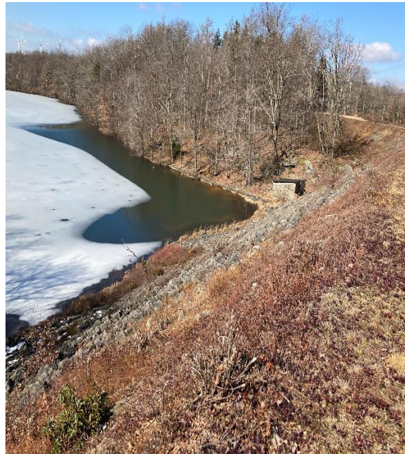
Figure 4 – Raven Run Dam No 3 – Downstream Slope and Crest
