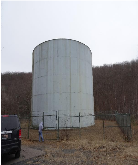
Figure 1 – Tank Looking East
