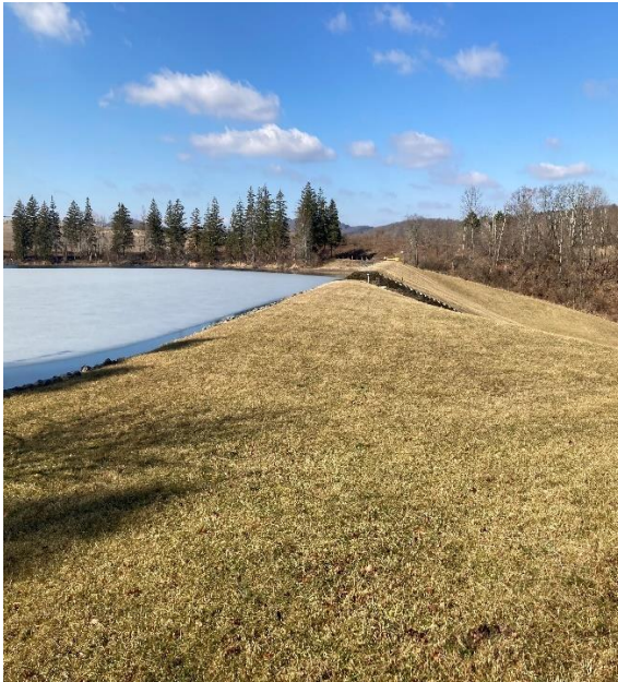
Figure 1 – Ringtown Dam No 5 –Downstream slope of Embankment
