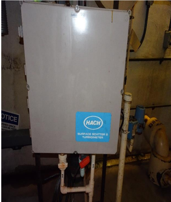
Figure 21 – Turbidity Meter
