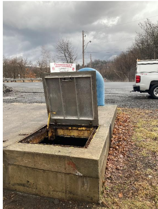
Figure 2 – Vault Entrance Hatch
