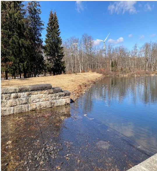
Figure 3 – Raven Run Dam No 3 – Spillway, Slope and Crest
