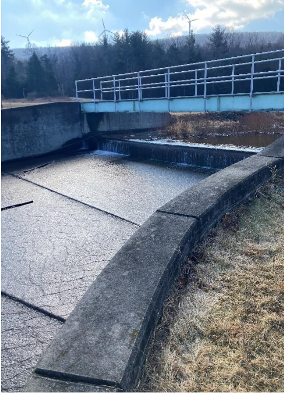
Figure 1 – Ringtown Dam No 6 – Concrete Spillway
