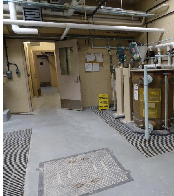
Figure 10 – Magnifloc Dosing Station
