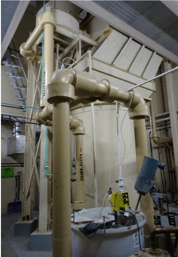
Figure 13 – Plate Separator
