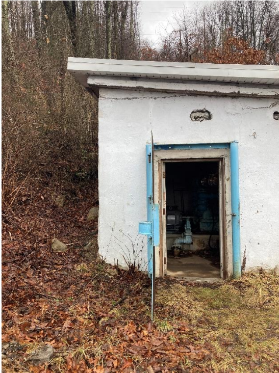
Figure 1 – Front of Building
