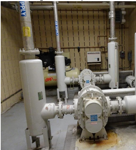
Figure 13 – Plate Separator
