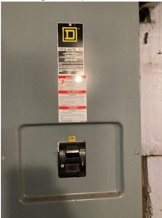
Figure 7 – Power Disconnect
