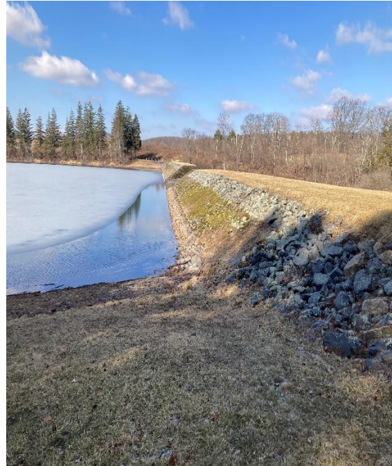
Figure 2 – Ringtown Dam No 5 –Upstream slope of Embankment
