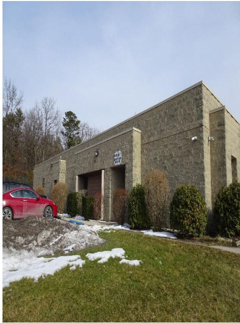
Figure 1 – Front of Treatment Building
