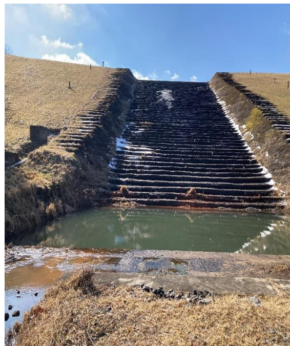
Figure 4 – Ringtown Dam No 5 –Roller Compacted Concrete Spillway
