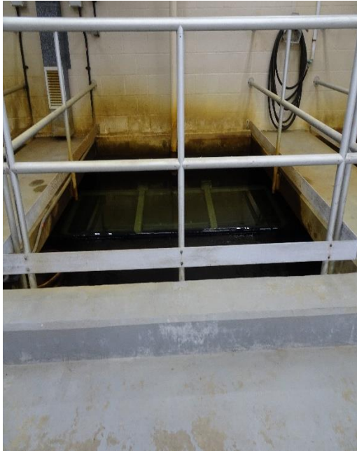
Figure 25 – Sand Filter
