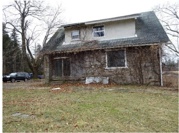
Figure 5 – Caretaker House Rear
