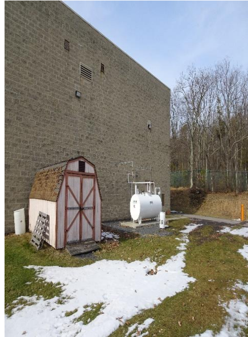
Figure 30 – Rear of Treatment Building
