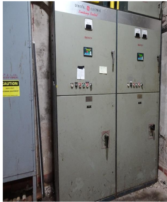
Figure 2 – Motor Starters
