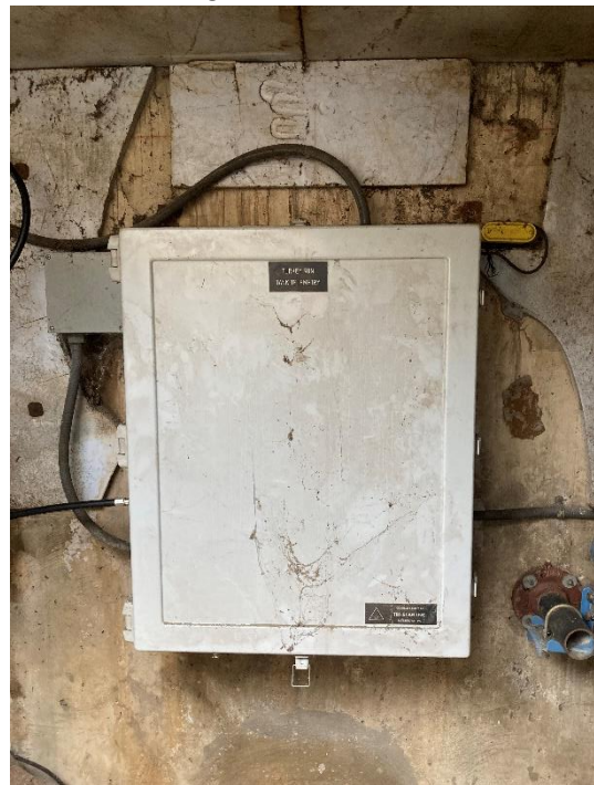
Figure 4 – Telemetry Box
