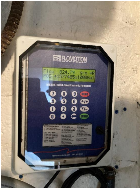
Figure 7 – Flow Reader
