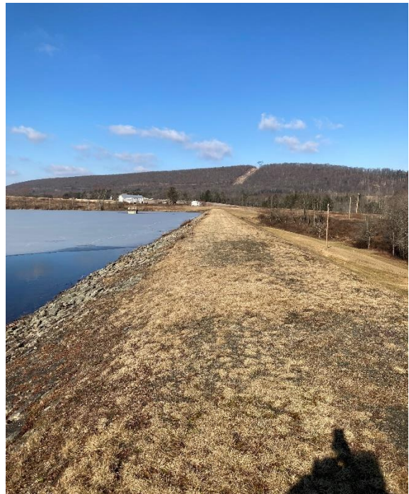
Figure 4 – Ringtown Dam No 6 – Embankment Crest and Crest Line
