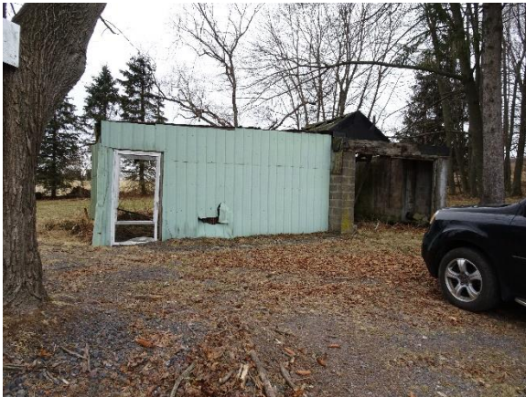
Figure 7 – Caretaker House Garage
