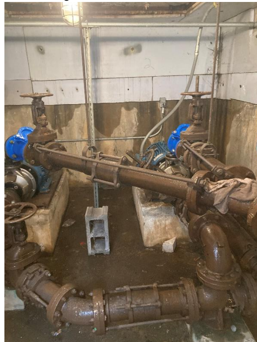
Figure 8 – Discharge Piping
