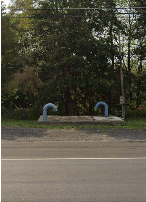
Figure 1 – Pump Station looking West
