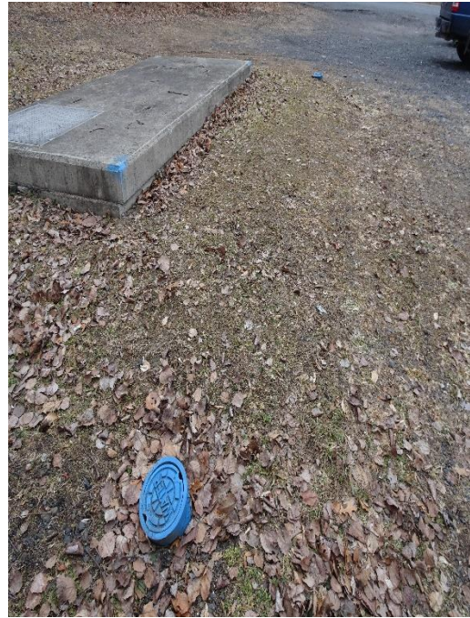
Figure 2 – Vault 2 looking East
