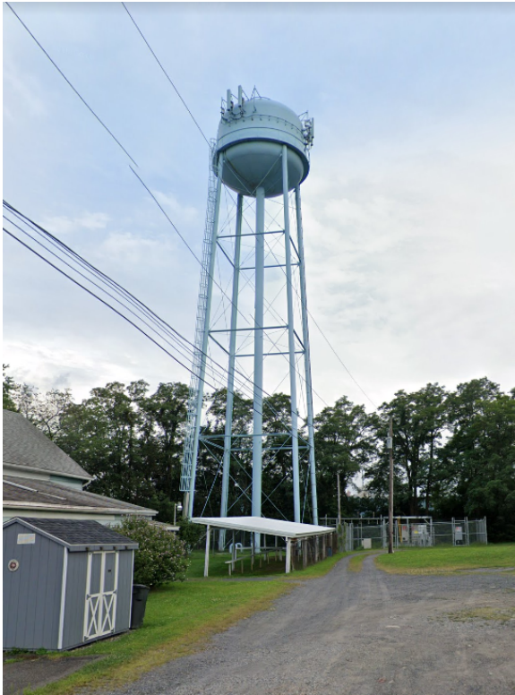
Figure 1 – Tank from Furnace Street
