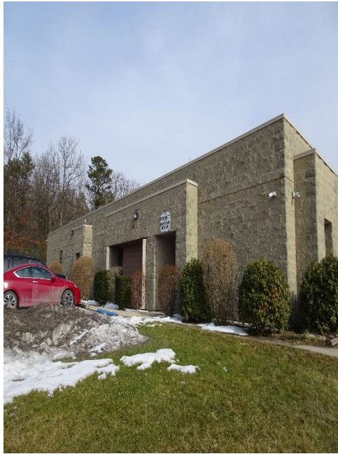
Figure 1 – Front of Treatment Building
