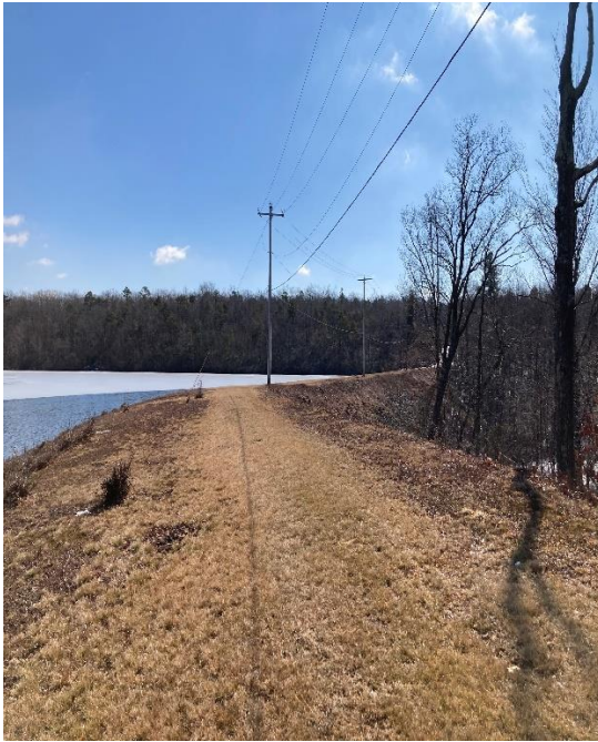
Figure 1 – Raven Run Dam No 3 – Embankment Crest
