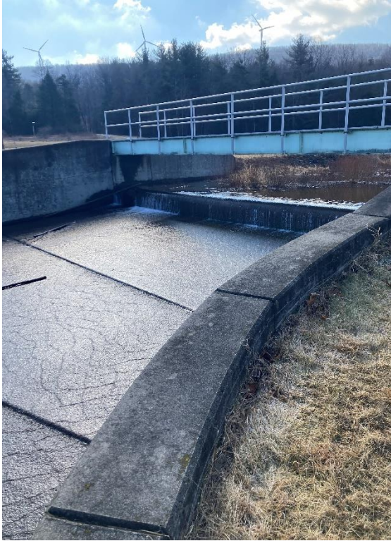
Figure 1 – Ringtown Dam No 6 – Concrete Spillway
