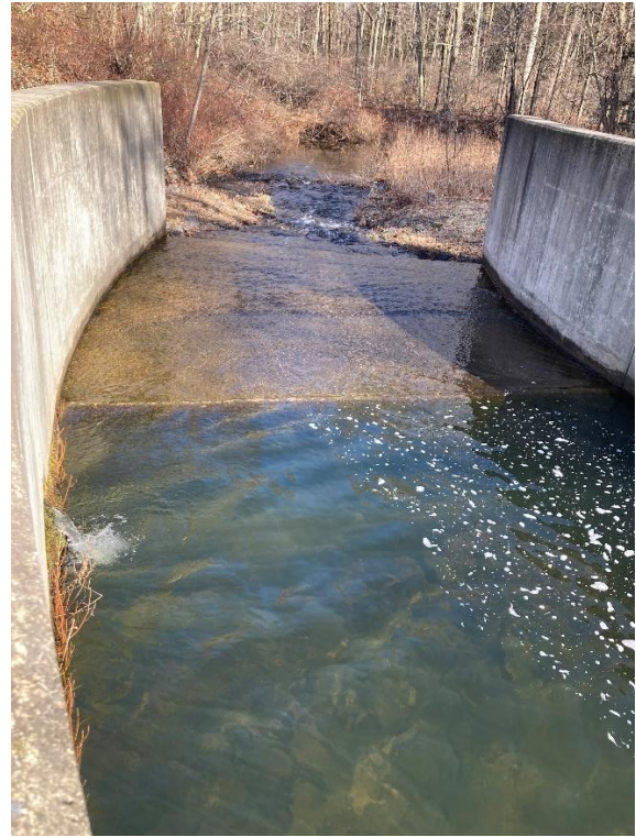
Figure 2 – Ringtown Dam No 6 – Concrete Spillway Channel at Toe
