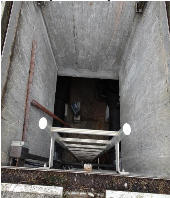
Figure 3 – Entrance to Valve Vault
