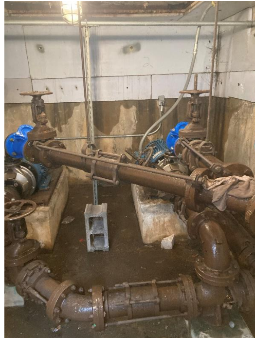
Figure 8 – Discharge Piping
