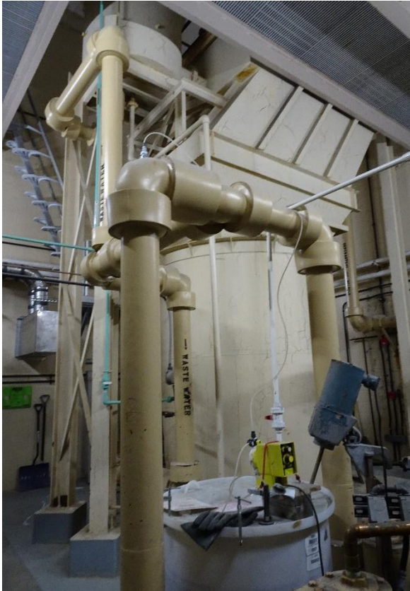
Figure 13 – Plate Separator
