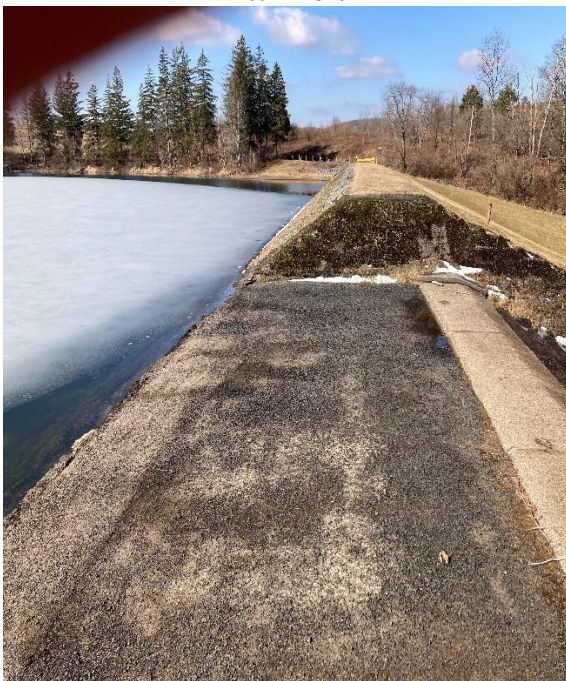
Figure 3 – Ringtown Dam No 5 – Crest of Roller Compacted Concrete Spillway
