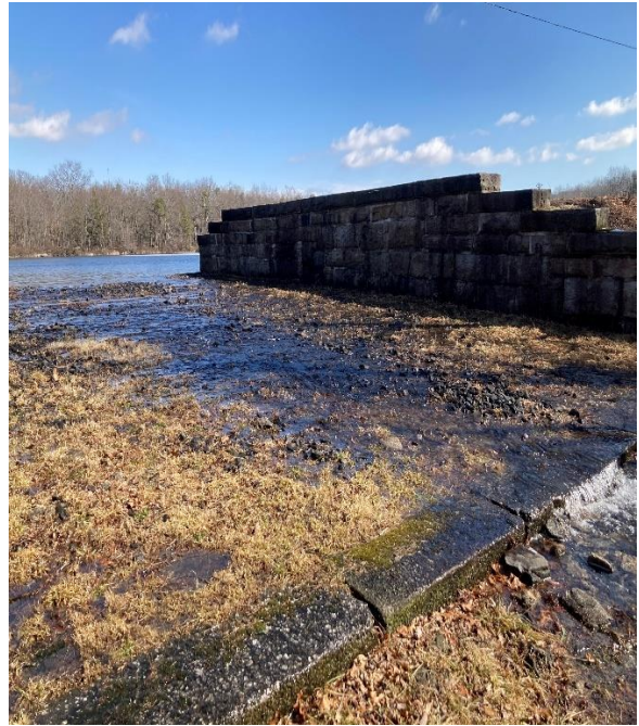
Figure 2 – Raven Run Dam No 3 – Spillway
