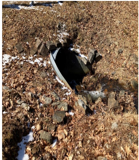
Figure 4 – Raven Run Dam No 2 – Downstream Spillway Channel Culvert
