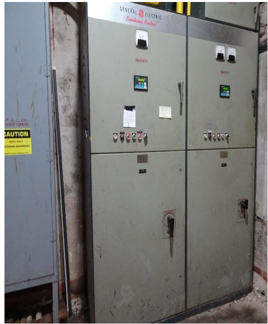
Figure 2 – Motor Starters
