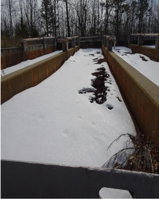
Figure 33 – Sand Filters
