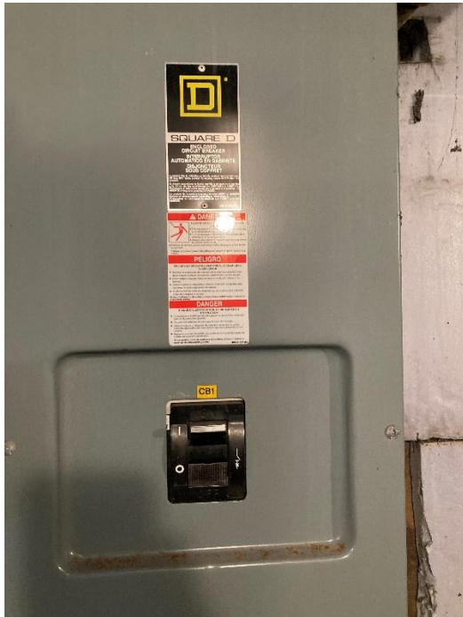
Figure 7 – Power Disconnect
