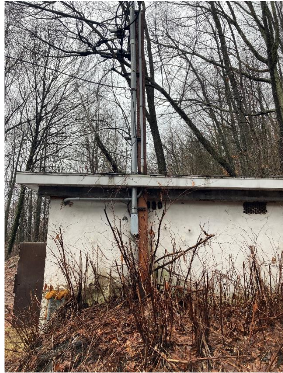
Figure 2 – Side of Building
