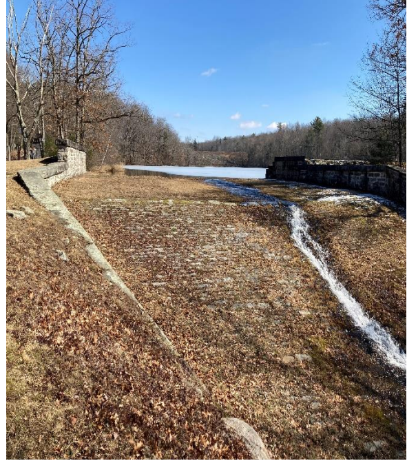
Figure 2 – Raven Run Dam No 2 - Spillway
