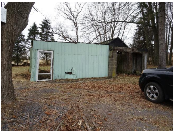
Figure 7 – Caretaker House Garage
