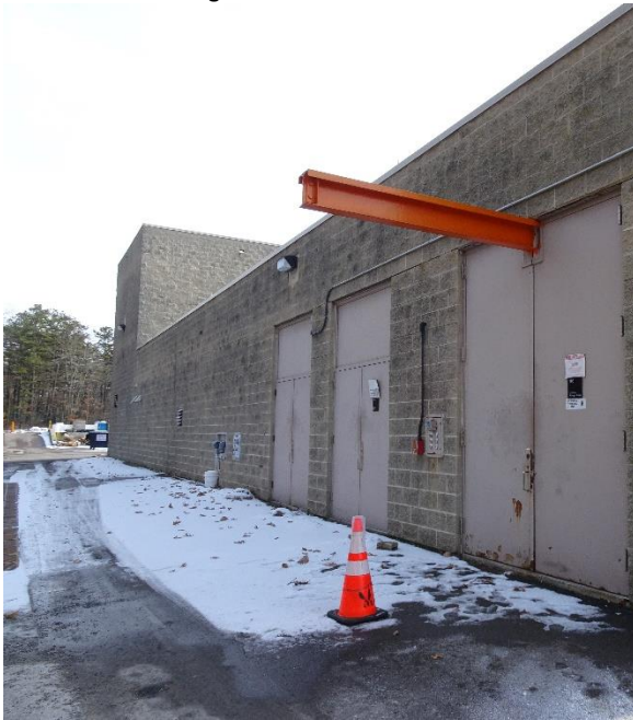
Figure 35 – North Side of WTP Building
