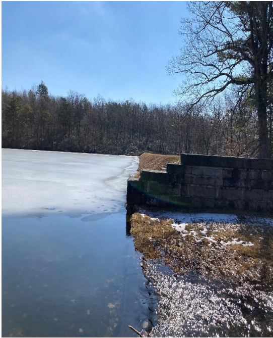
Figure 1 – Raven Run Dam No 2 – Embankment Slope at spillway
