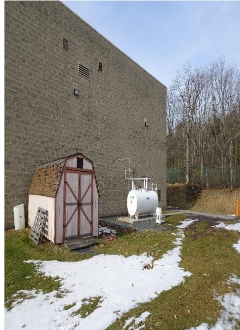
Figure 30 – Rear of Treatment Building
