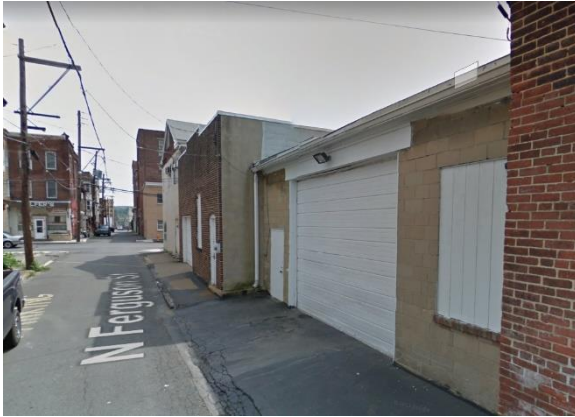
Figure 5 –Maintenance and Warehouse Buildings
