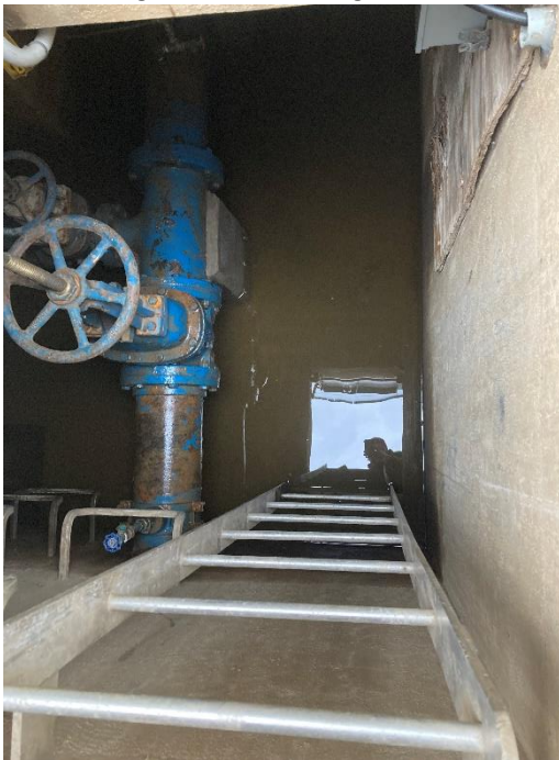
Figure 3 – Entrance to Valve Vault
