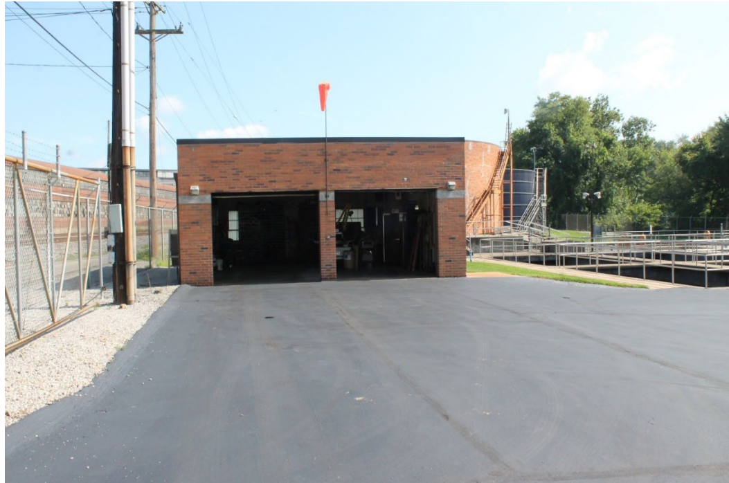
FIGURE 5.3 - 51: MAINTENANCE GARAGE AND TOOL SHOP BUILDING
