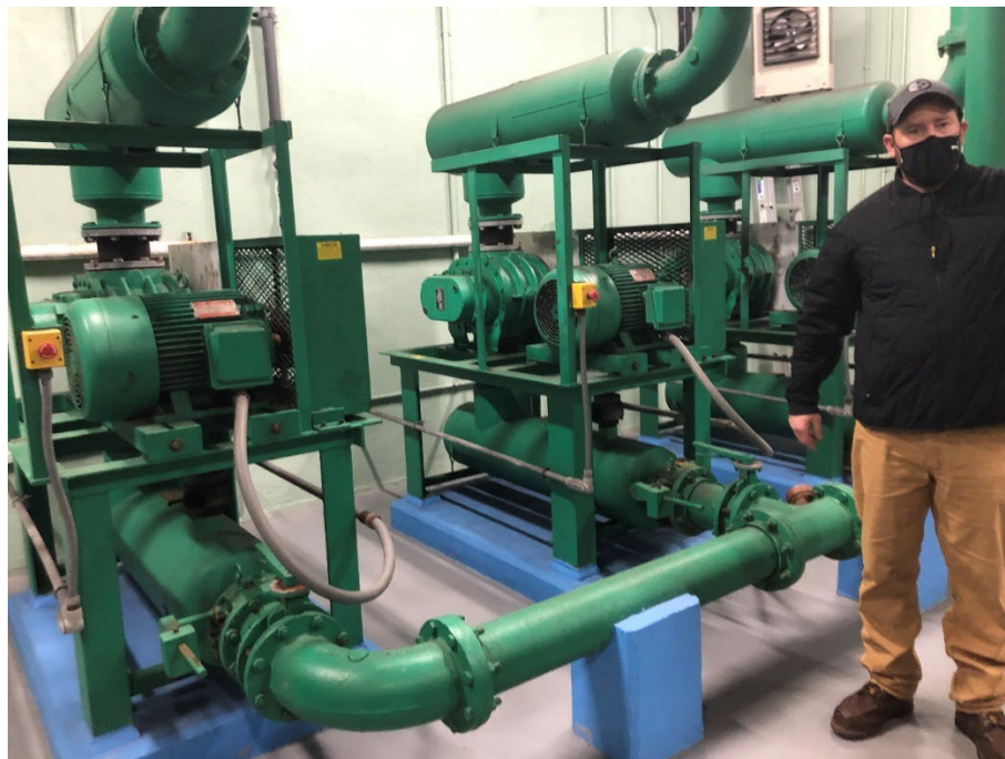
FIGURE 5.3 - 5: SECONDARY/PRIMARY EFFLUENT PUMPS
