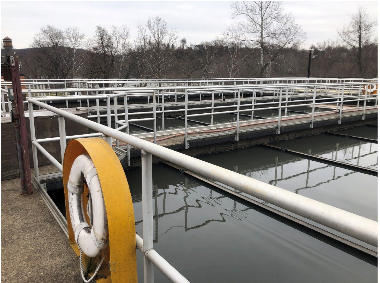
FIGURE 5.3 - 7: PRIMARY SETTLING TANKS-TOP VIEW
