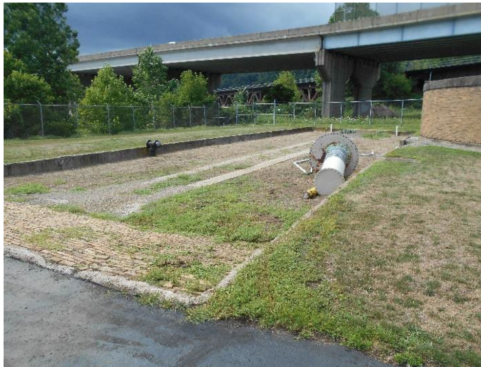
FIGURE 5.3 - 26: REMAINING SLUDGE DRYING BED
