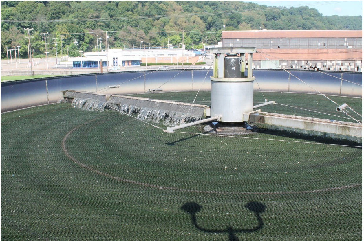
FIGURE 5.3 - 9: OXIDATION TOWER-TOP VIEW
