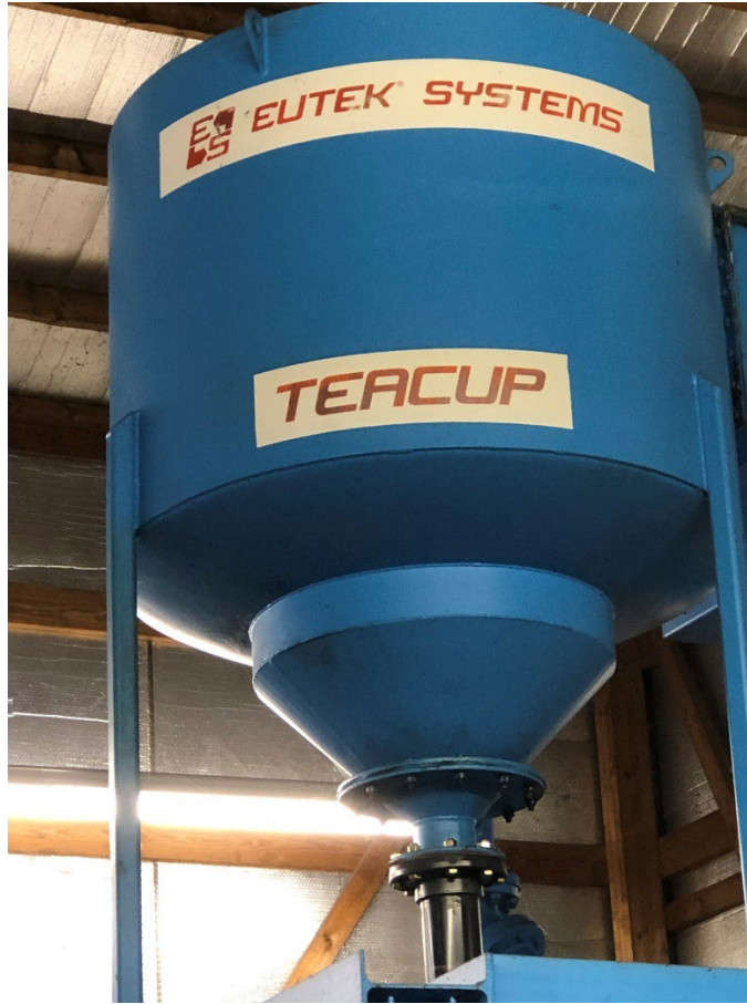
FIGURE 5.3 - 20: GRIT SEPARATOR EQUIPMENT
