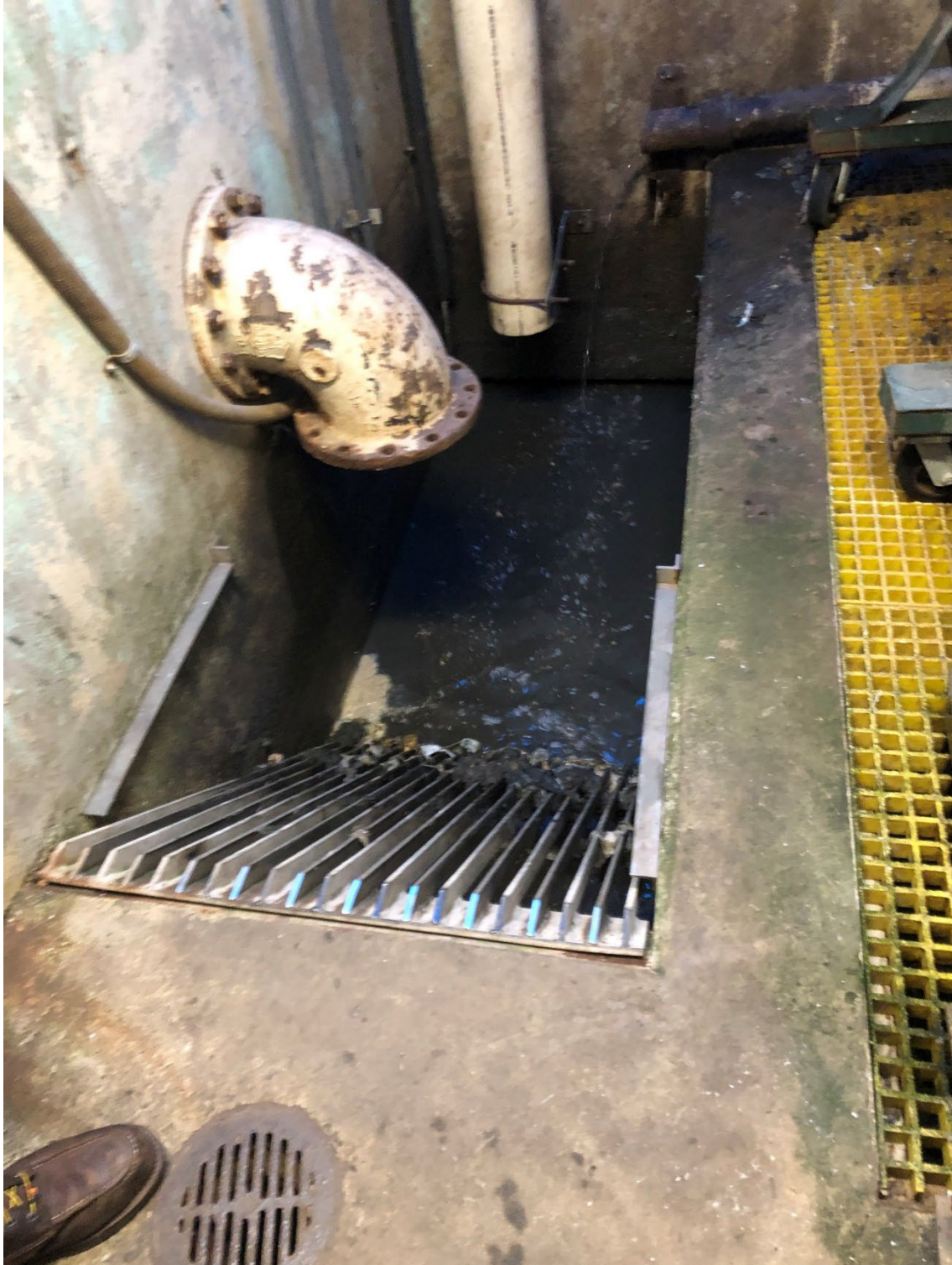
FIGURE 5.3 - 2: MANUAL BAR SCREEN
