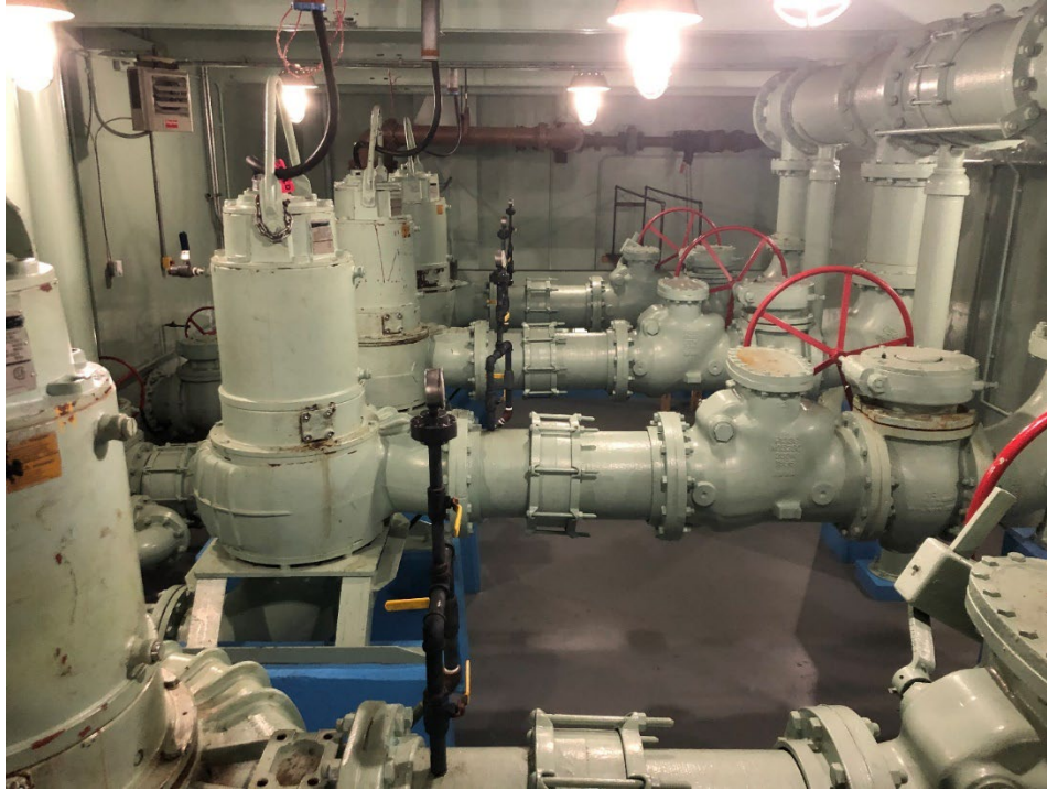
FIGURE 5.3 - 5: SECONDARY/PRIMARY EFFLUENT PUMPS
