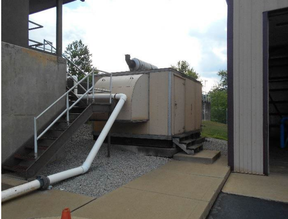
FIGURE 5.3 - 37: EMERGENCY GENERATOR
