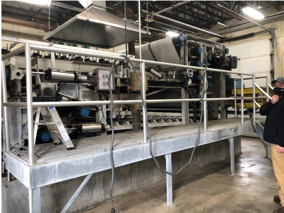
FIGURE 5.3 - 17: BELT FILTER PRESS
