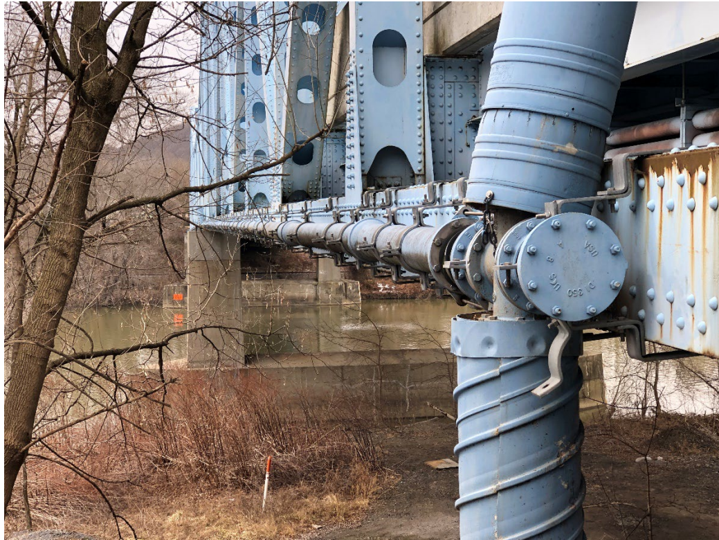
FIGURE 5.1-1: EASTVALE PUMP STATION FORCE MAIN RIDING THE SR0588 BRIDGE
