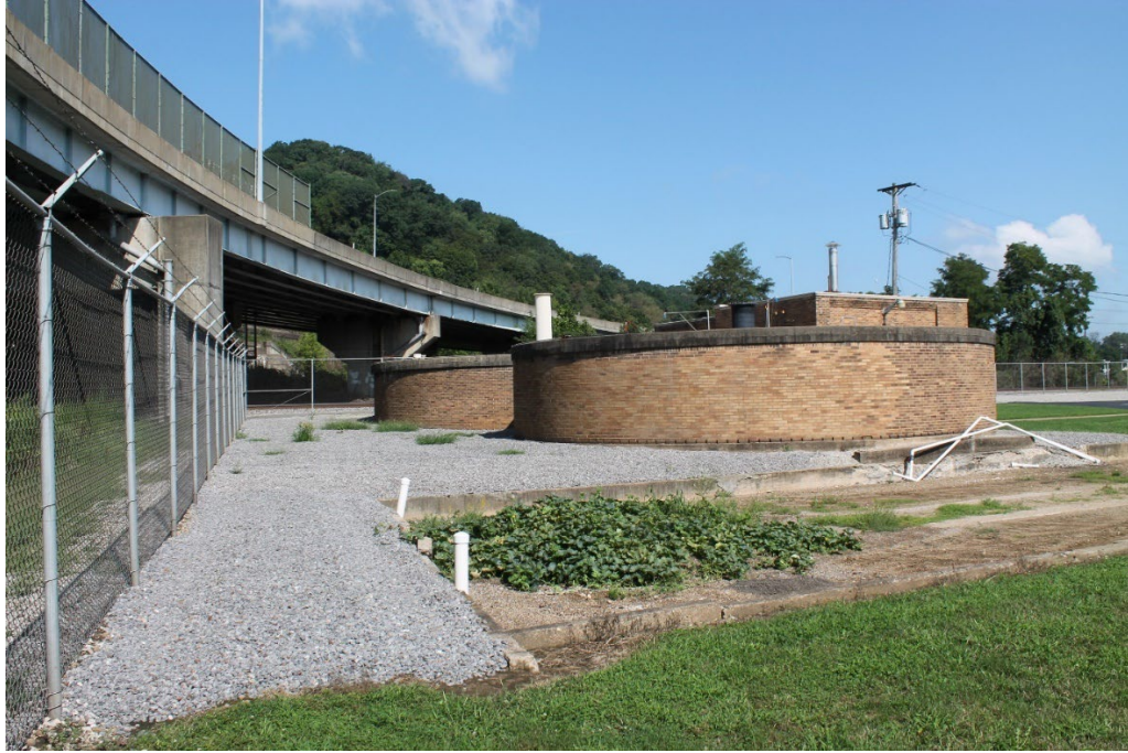
FIGURE 5.3 - 23: ANAEROBIC DIGESTER TANKS - SIDE VIEW
