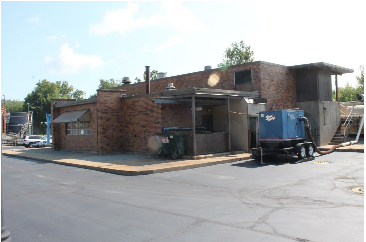
FIGURE 5.3 - 1: HEADWORKS-PRELIMINARY TREATMENT BUILDING
