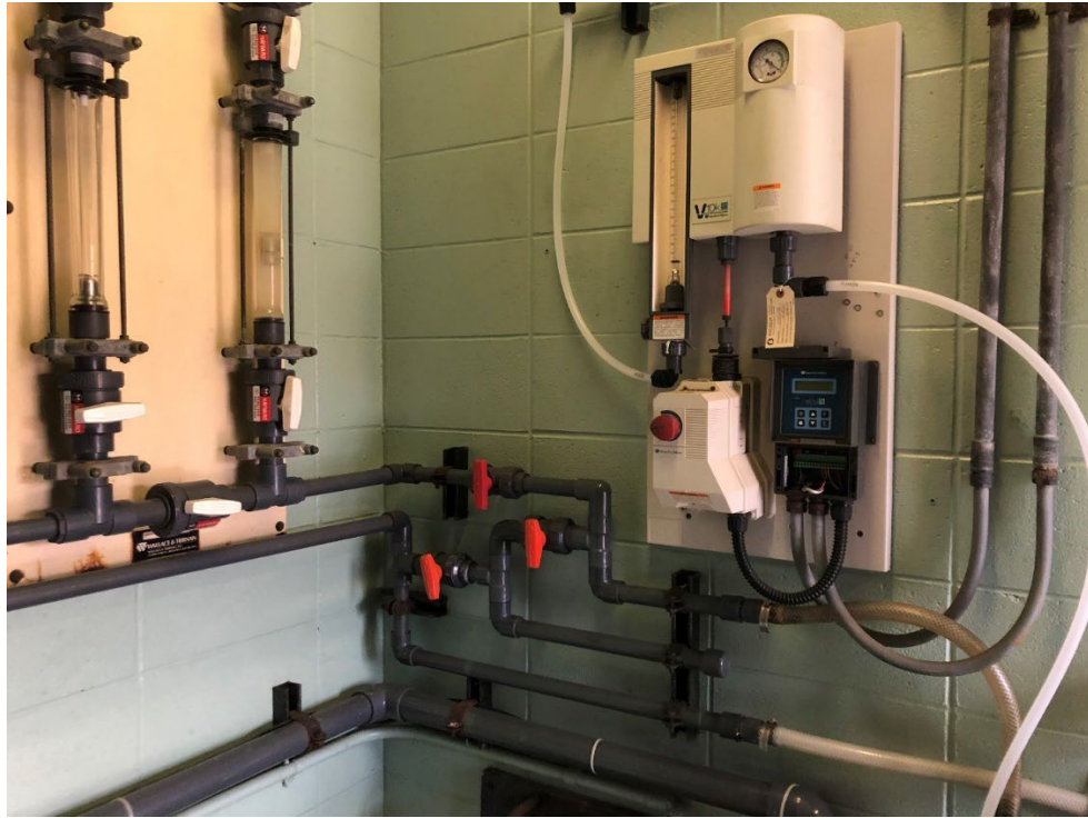
FIGURE 5.3 - 12: CHLORINATOR
