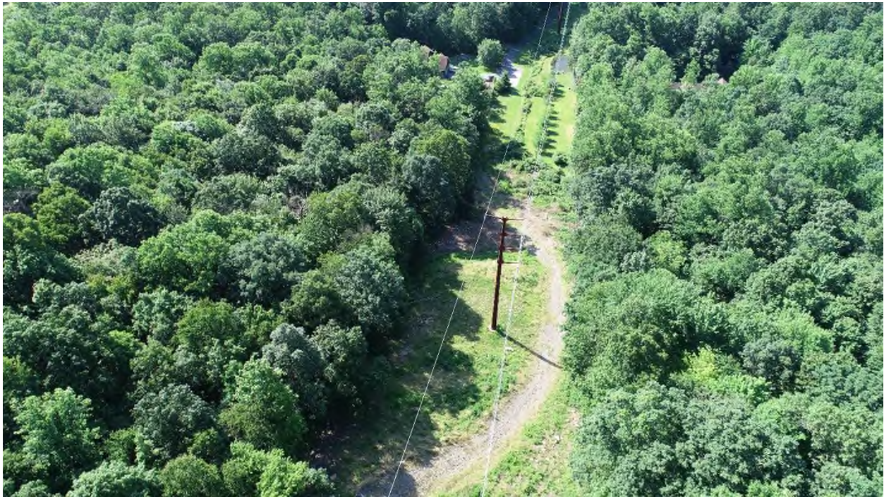
Photograph 2 – June 19, 2022 Photograph Facing Southeast
