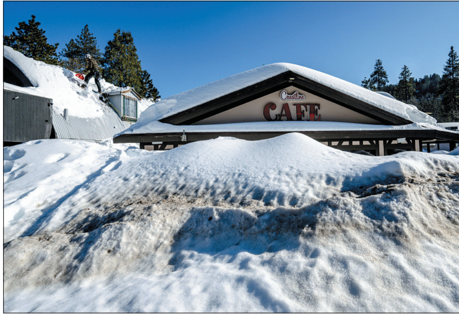
WATCHARA PHOMICINDA — THE ORANGE COUNTY REGISTER VIA AP A man shovels snow off the roof of a store in Crestline on Friday as buildings remain buried in several feet of snow from recent winter storms.
