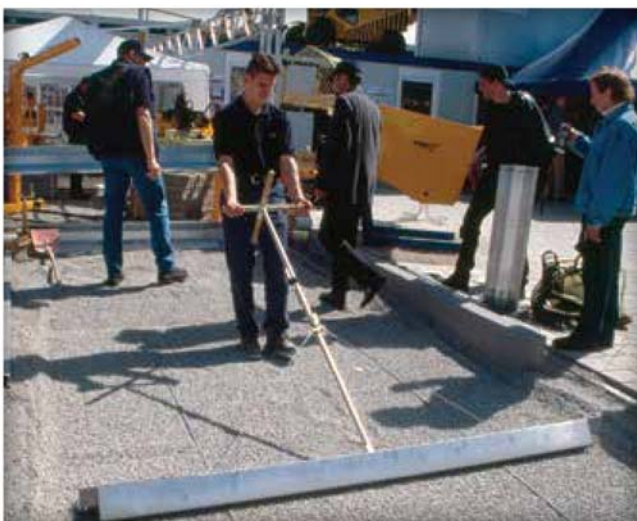
Figure 25. Manually screeding the No. 8 stone setting bed.
