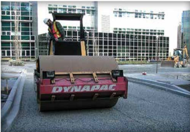
Figure 21. A 10 ton (9 T) roller compacts the ASTM No. 57 base.
