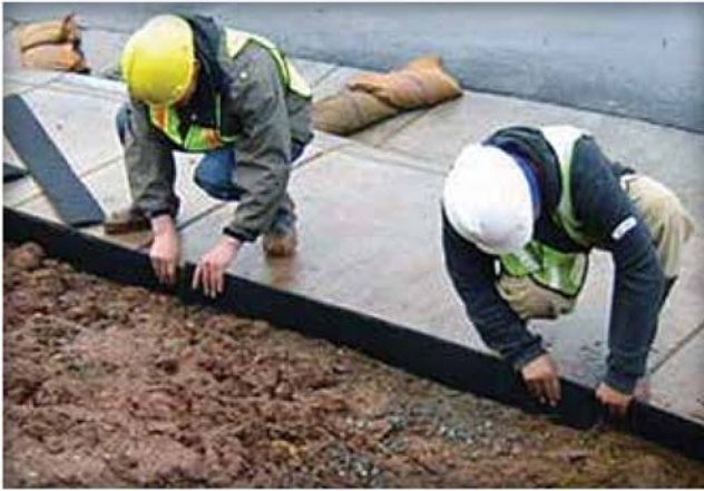
Figure 10. This temporary permeable edging around bare soil replaces silt fencing because it restrains sediment while allowing water to pass.
