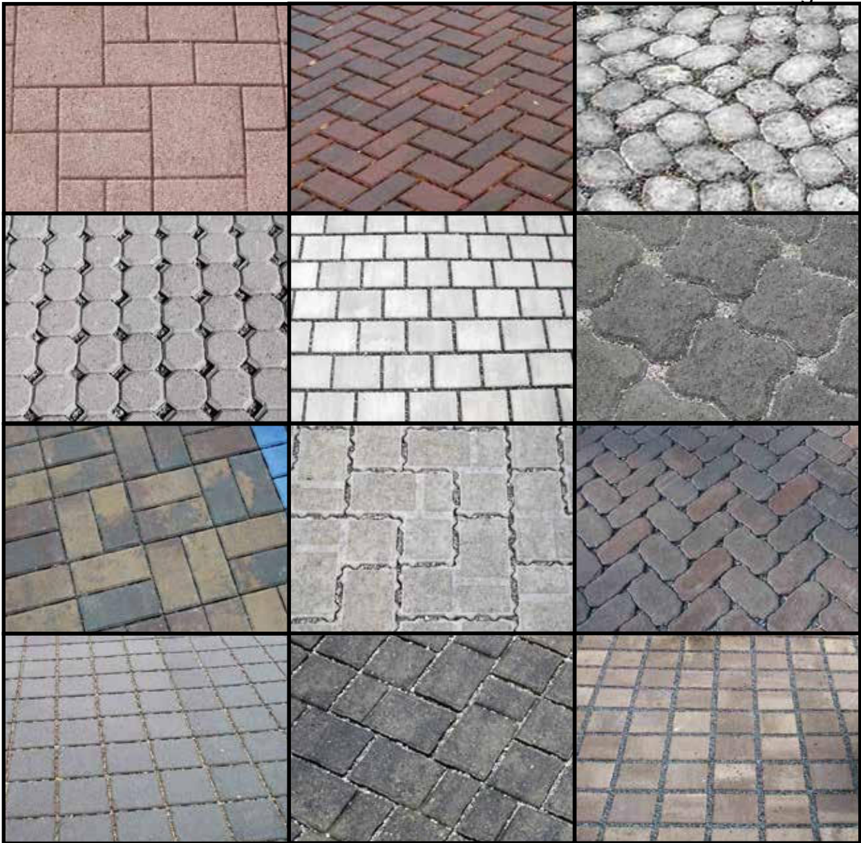
Figure 2. Various types of paving units used in PICP
