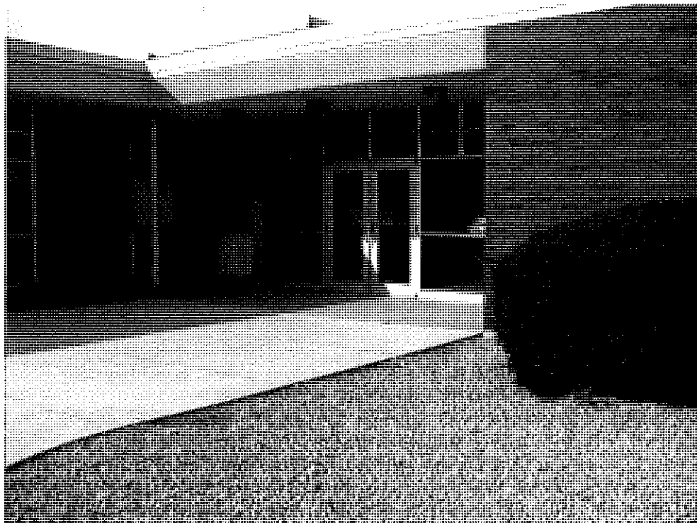
Figure 5-A ALCOSAN Old Operations & Maintenance Building
