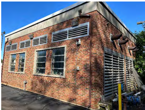
Emergency Generator Building
