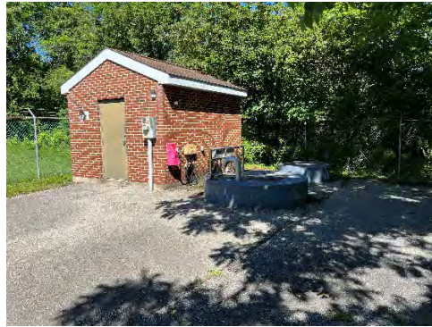
Control Building and Wetwell
