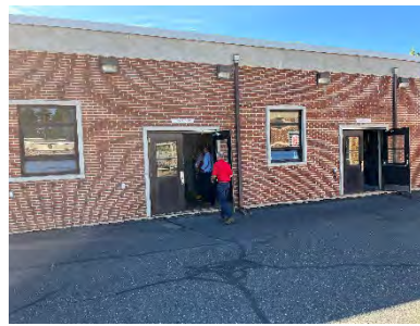
Sludge Blower/Pump Building
