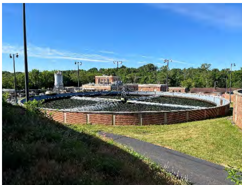
Trickling Filter
