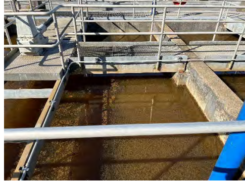
Flocculation Tanks
