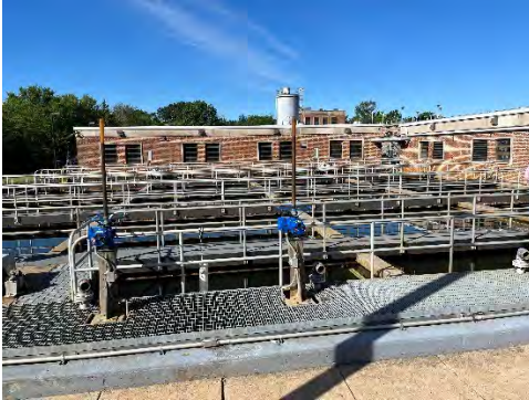
Final Settling Tanks
