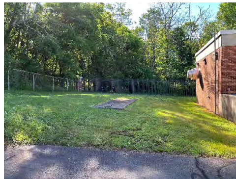
Underground Diesel Tanks
