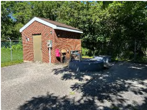
Control Building and Wetwell
