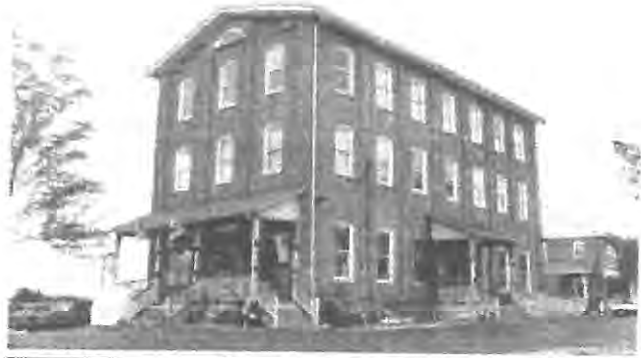
Vernfield is one of the many on-site sewer problem areas that have been corrected since 1972.
