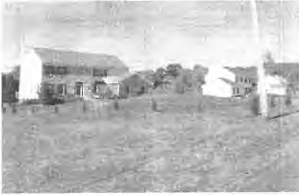
This home in Upper Salford Township uses a sand mound for sewage collection treatment and disposal.
