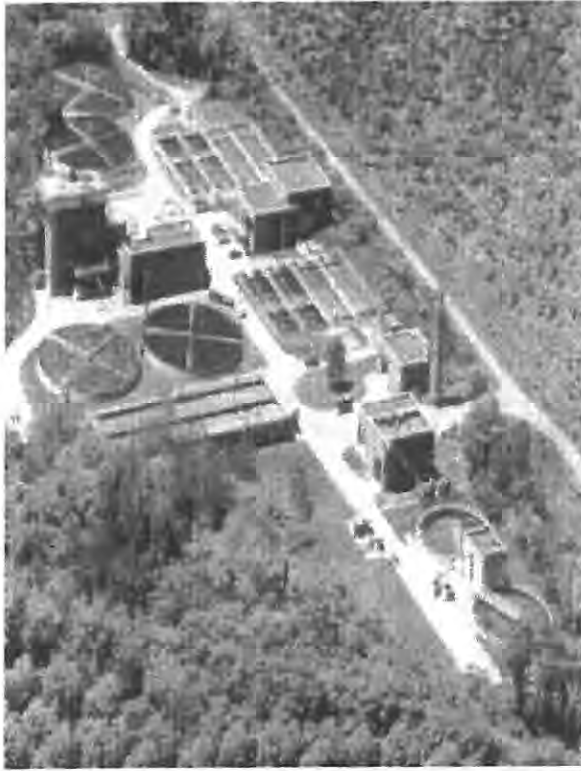
Example sewage treatment plant.
