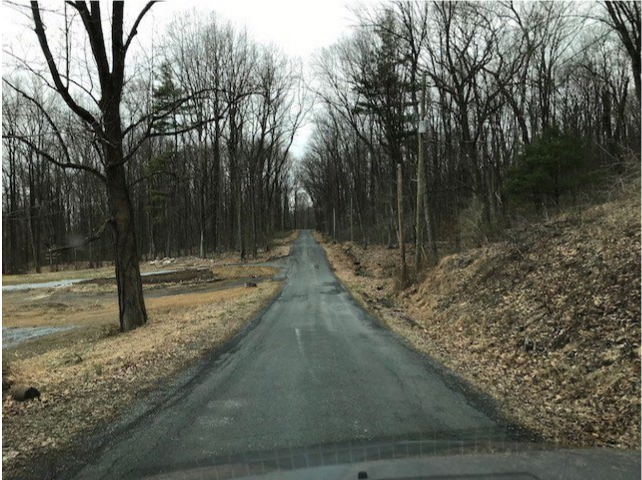
Figure 1: Single phase primary along Sousley Road. Note the tall, overhanging limbs from OROW trees.
