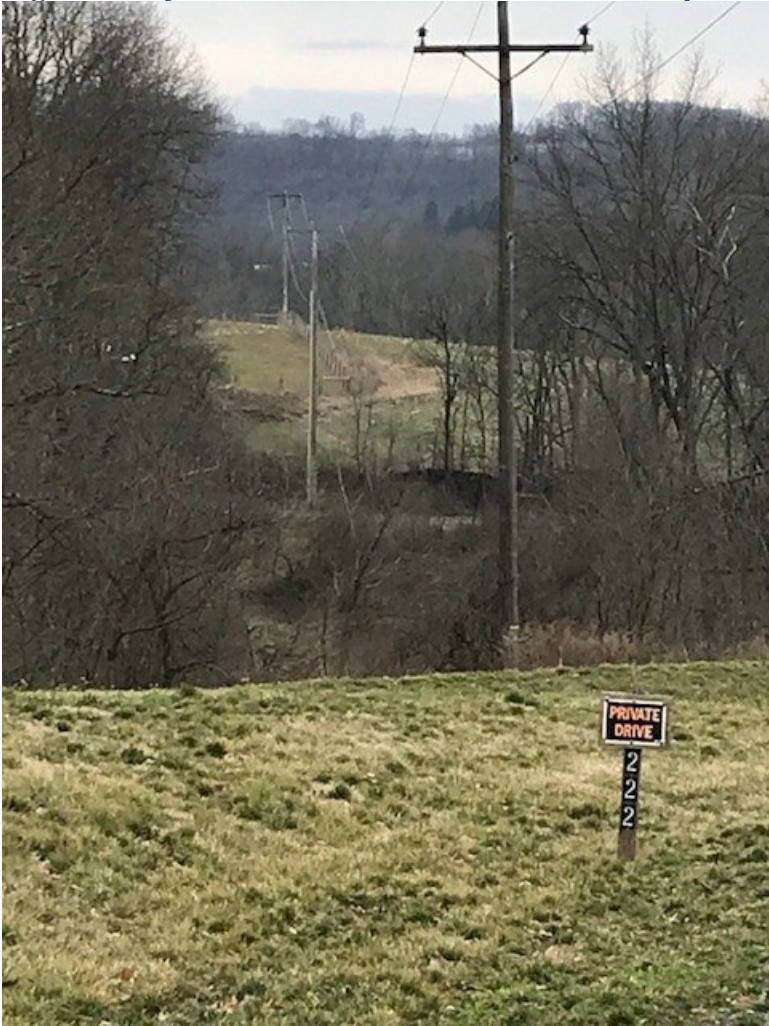
Figure 4: Lynnville 737-1 12kV OROW with adequate tree trimming.
