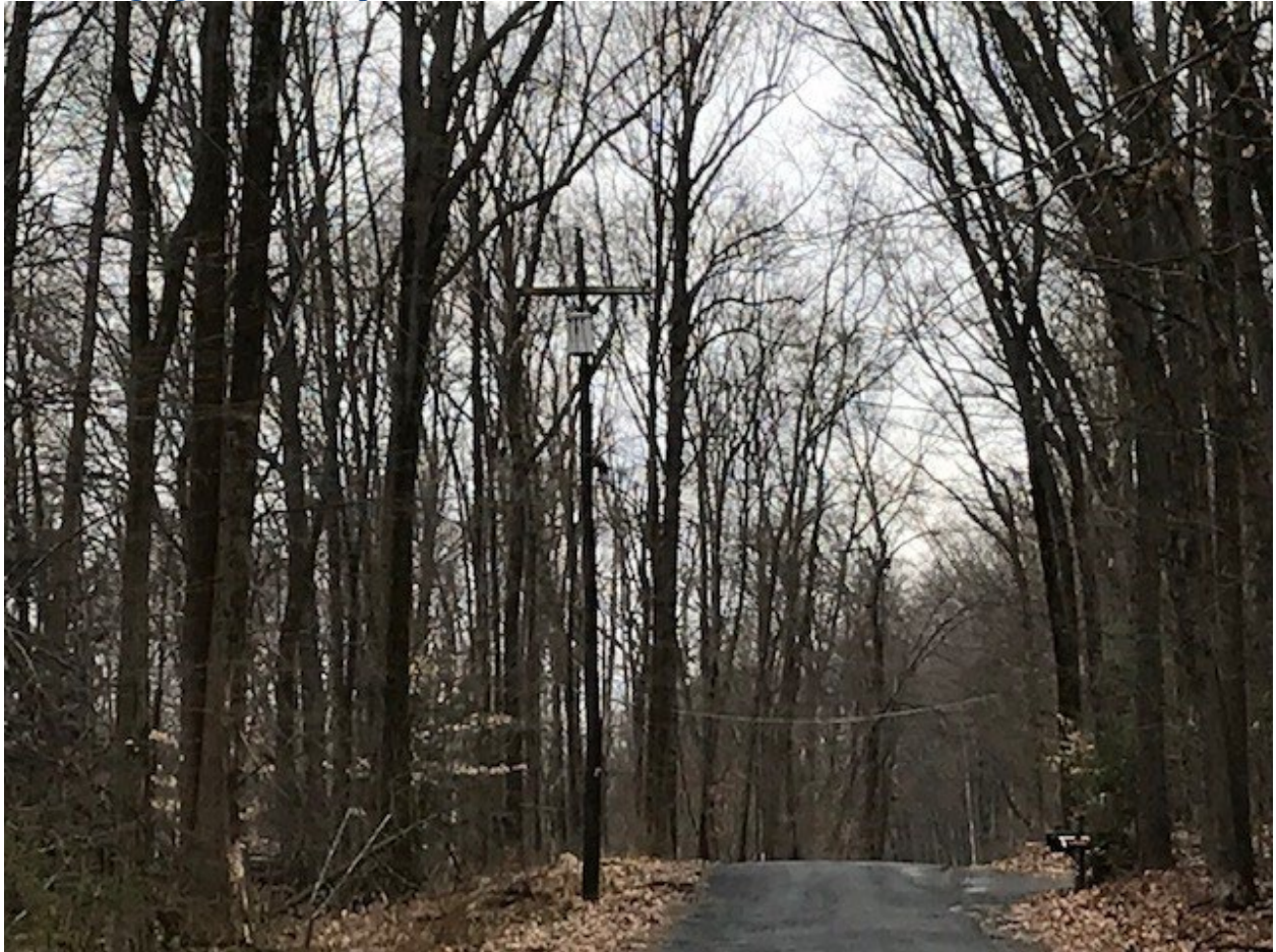
Figure 6: Sousley Rd looking West. Note the very tall canopy trees and overhanging limbs. This area is trimmed in accordance with Met-Ed's Vegetation Management Policy, but over-hanging limbs are a possible issue.
