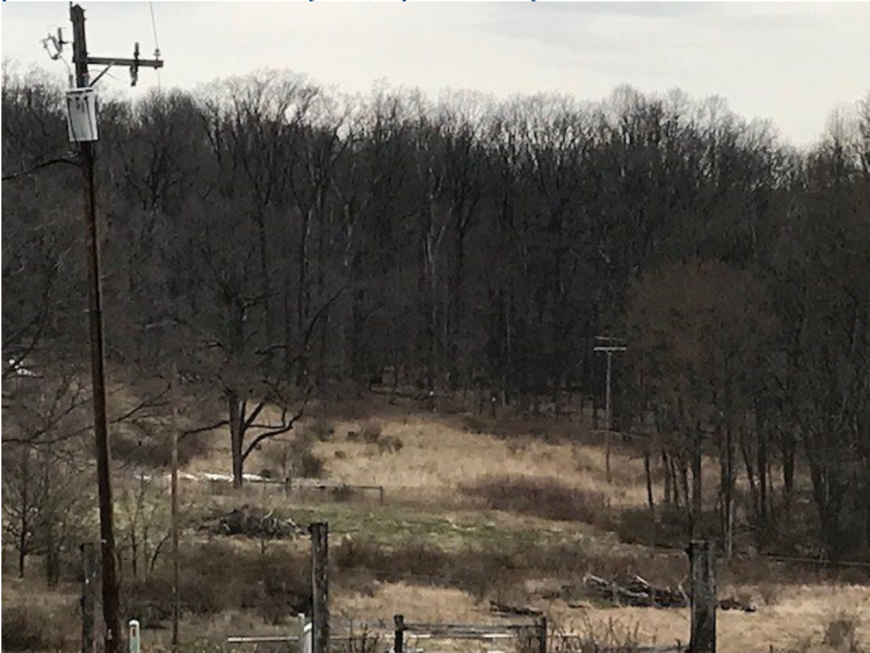
Figure 5: Single-phase tap off of the two-phase tap that serves Sousley Rd. Note the two-phase location is South of Sousley Rd and predominantly forested and inaccessible.
