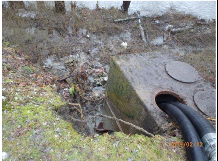
Greenville Sanitary Authority STP PA0027367 2/12/2019 Siphon Chamber
