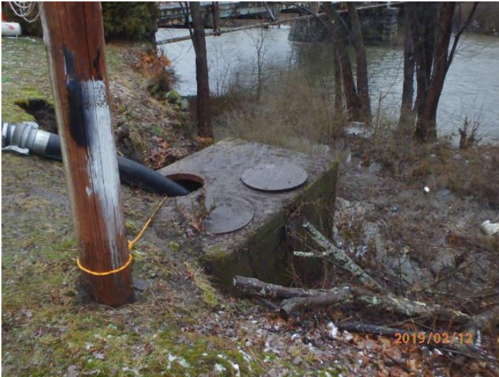
Greenville Sanitary Authority STP PA0027367 2/12/2019 Siphon Chamber
