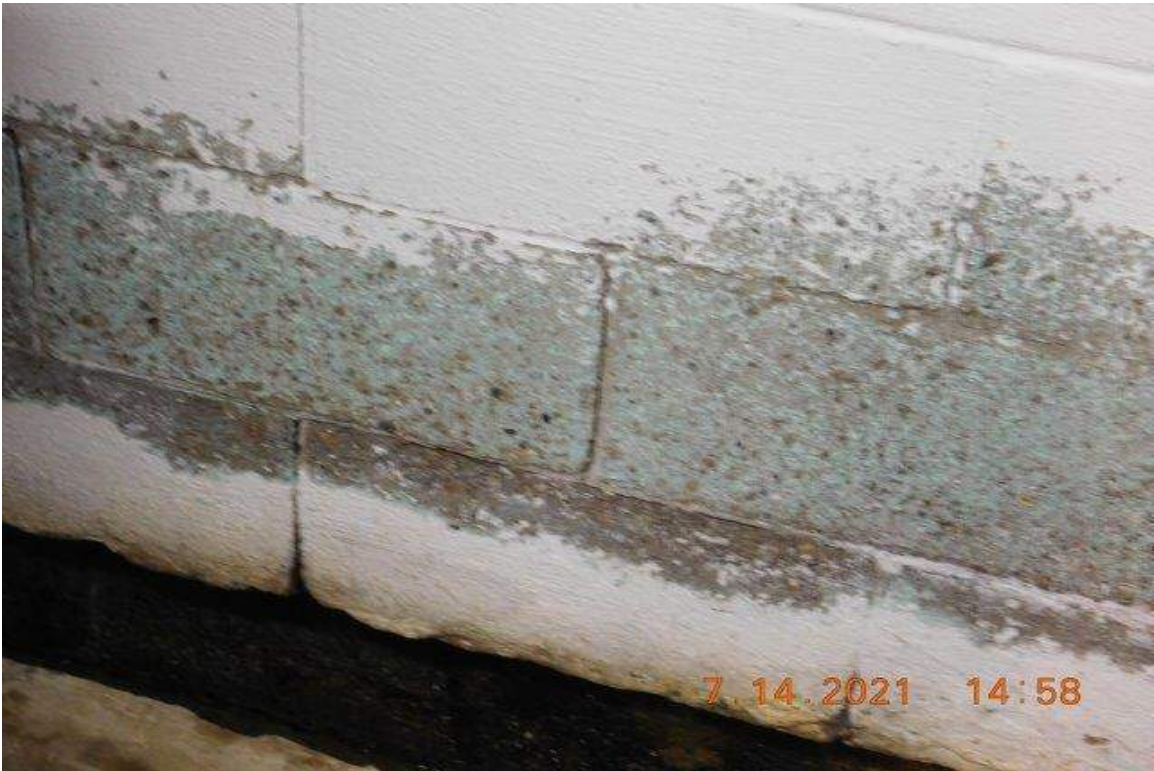
PHOTO 31 - CLOSE-UP OF AREA ON PHOTO 30
