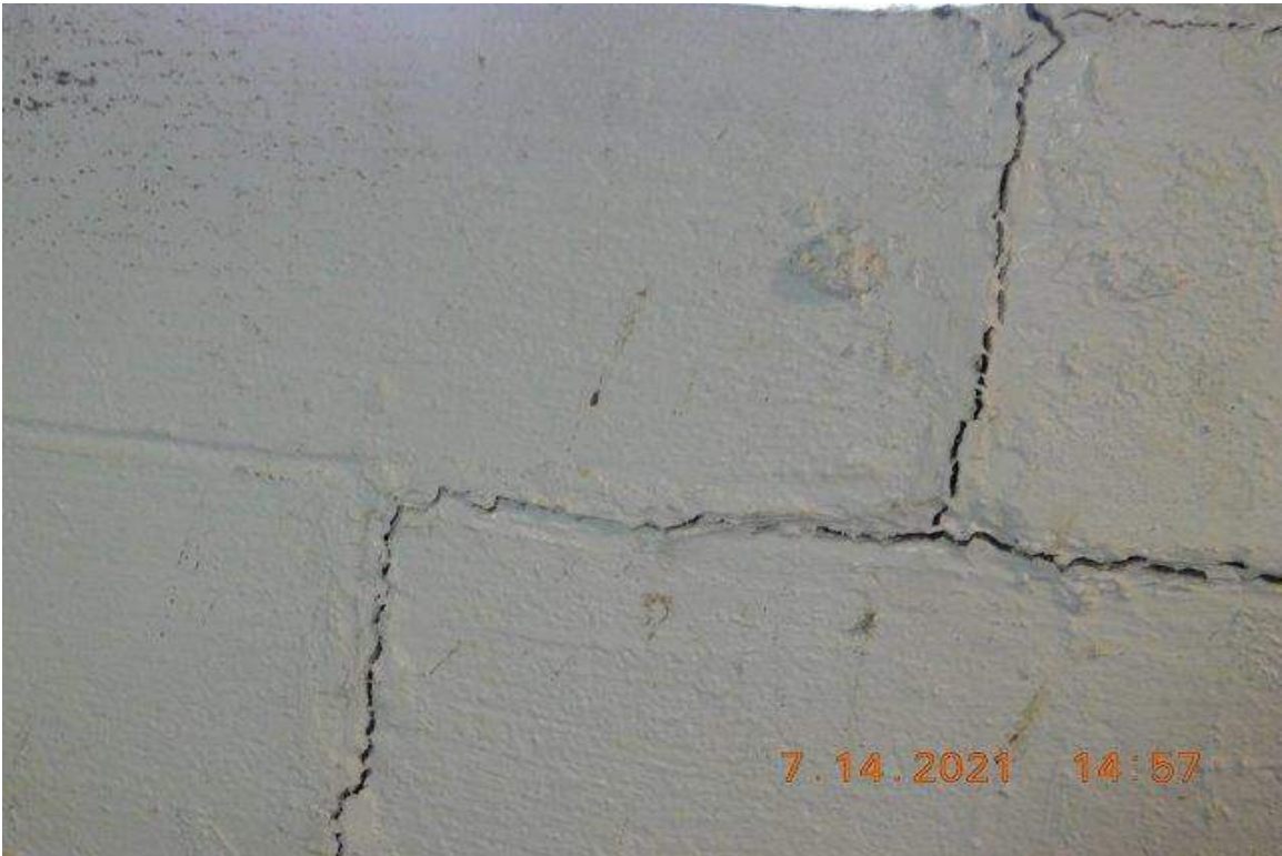
PHOTO 13 - CLOSE-UP OF AREA ON PHOTO 12
