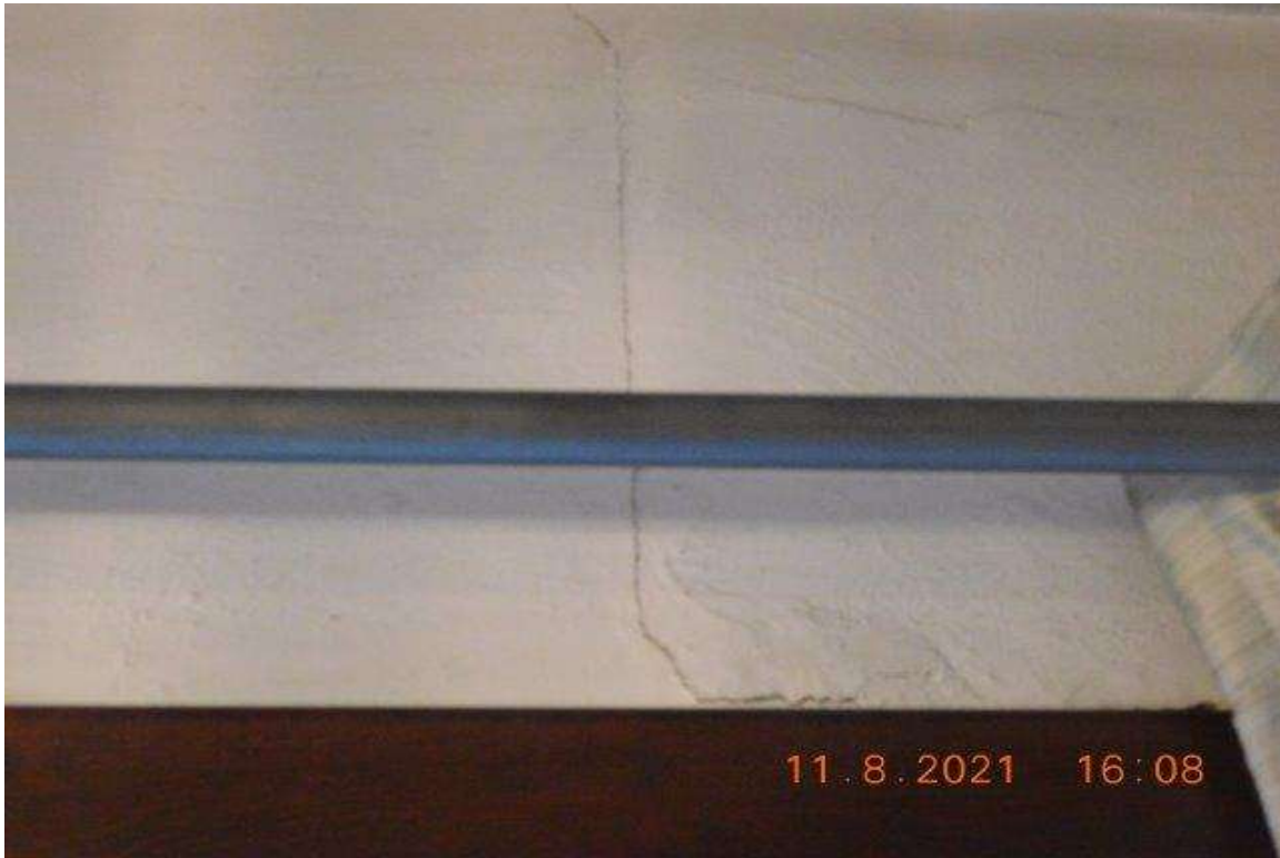
PHOTO 43 - CLOSE-UP OF AREA ON PHOTO 42
