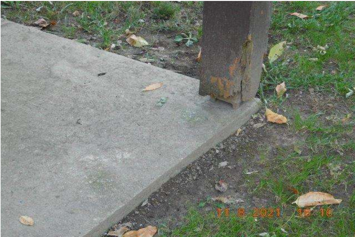
PHOTO 13 - CLOSE-UP OF REAR (SOUTH) PATIO RIGHT ROOF SUPPORT POST
