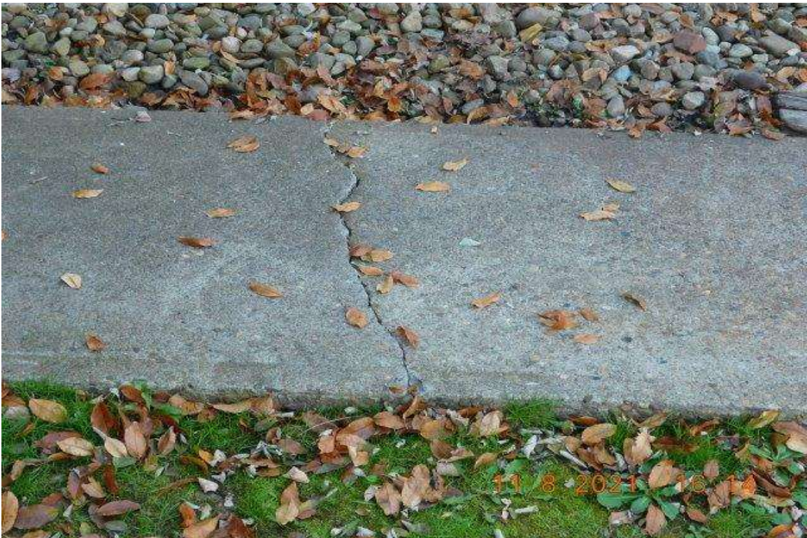
PHOTO 2 - CLOSE-UP OF AREA ON PHOTO 1
