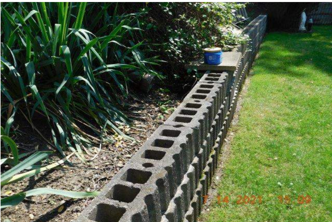
PHOTO 54 - LEFT YARD RETAINING WALL LOOKING SOUTH
