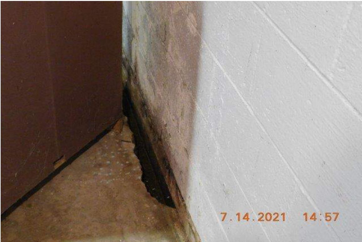
PHOTO 23 - AREA LEFT OF PHOTO 22
