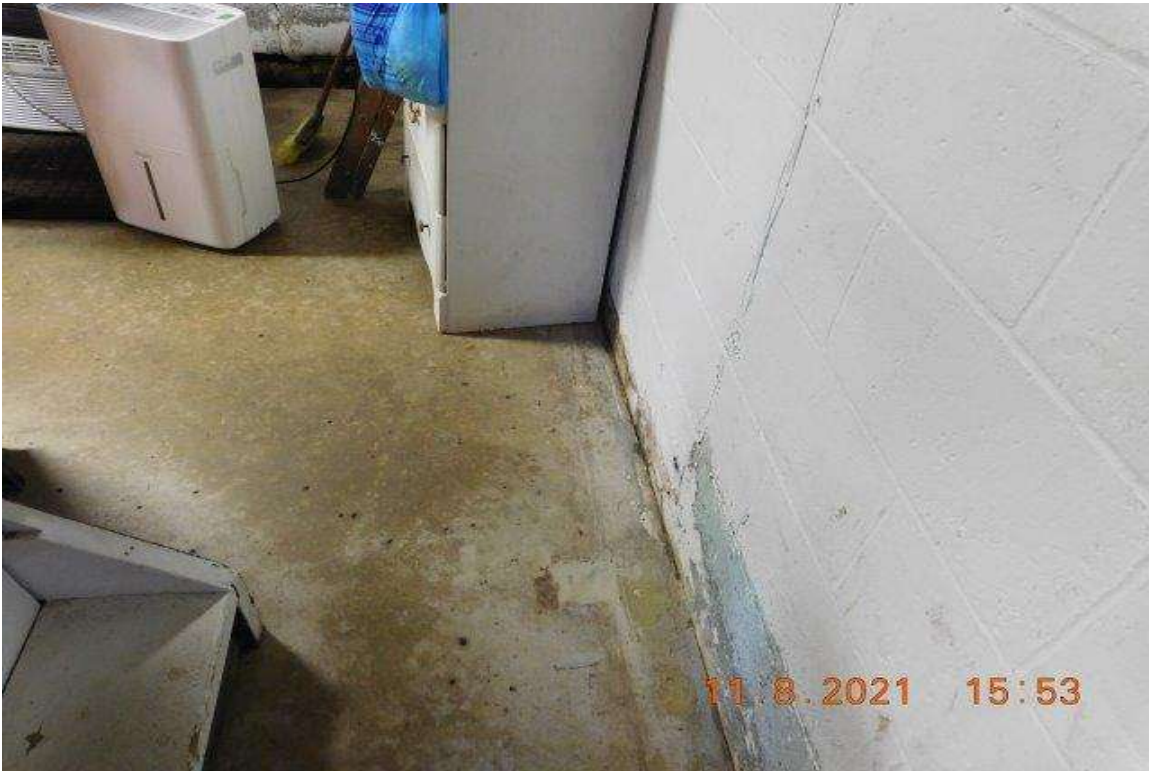
PHOTO 31 - RIGHT WALL OF BASEMENT REAR ROOM
