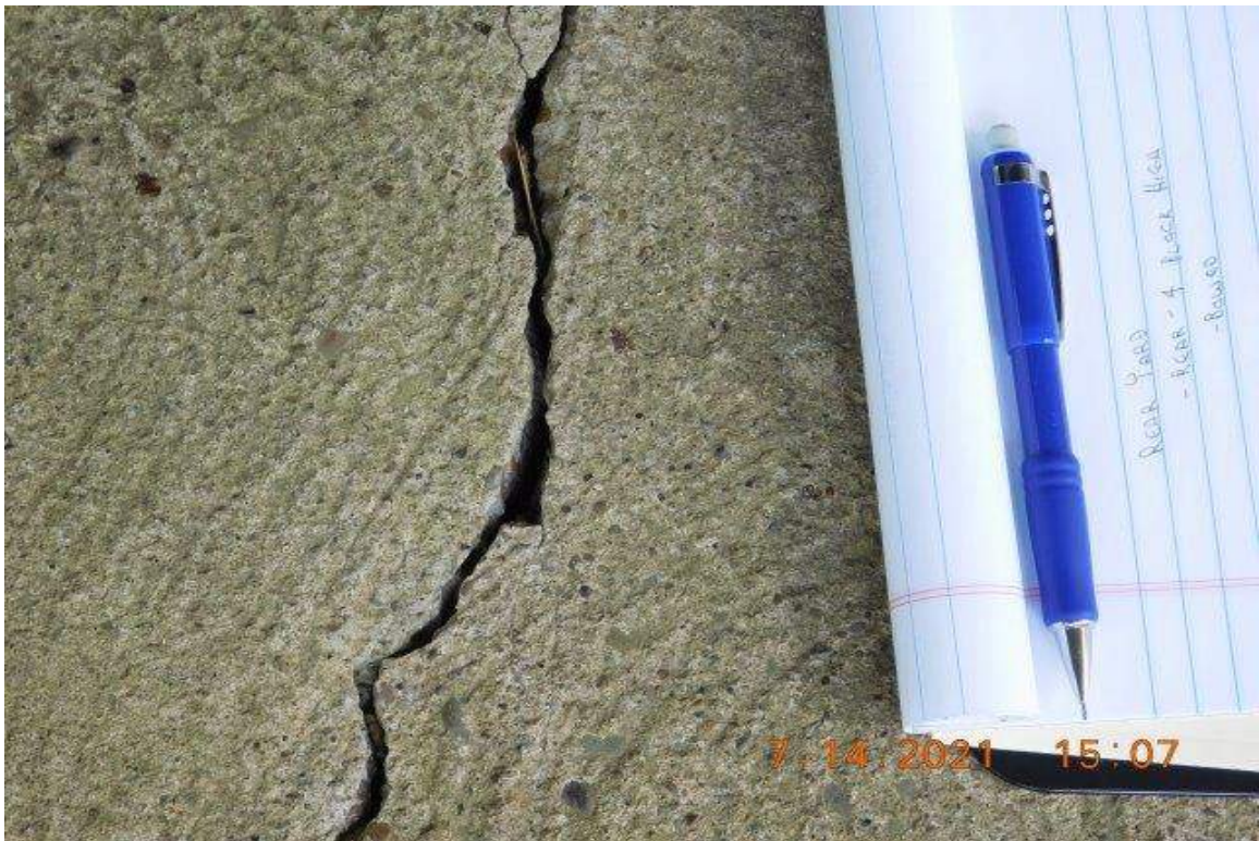
PHOTO 47 - CLOSE-UP OF AREA ON PHOTO 46
