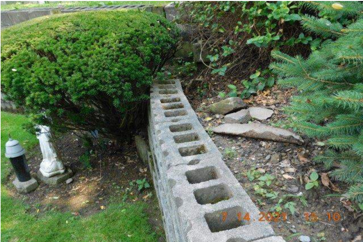
PHOTO 53 - CLOSE-UP OF AREA ON PHOTO 52
