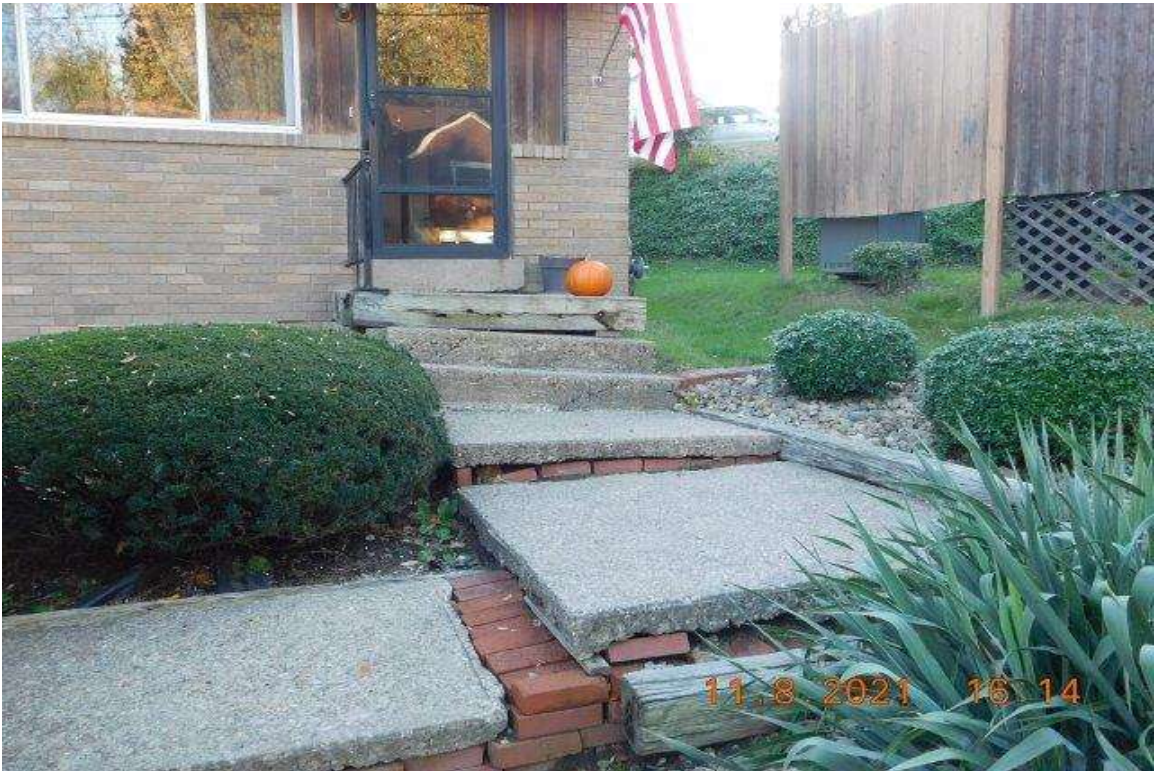
PHOTO 7 - CLOSE-UP OF AREA ON PHOTO 6
