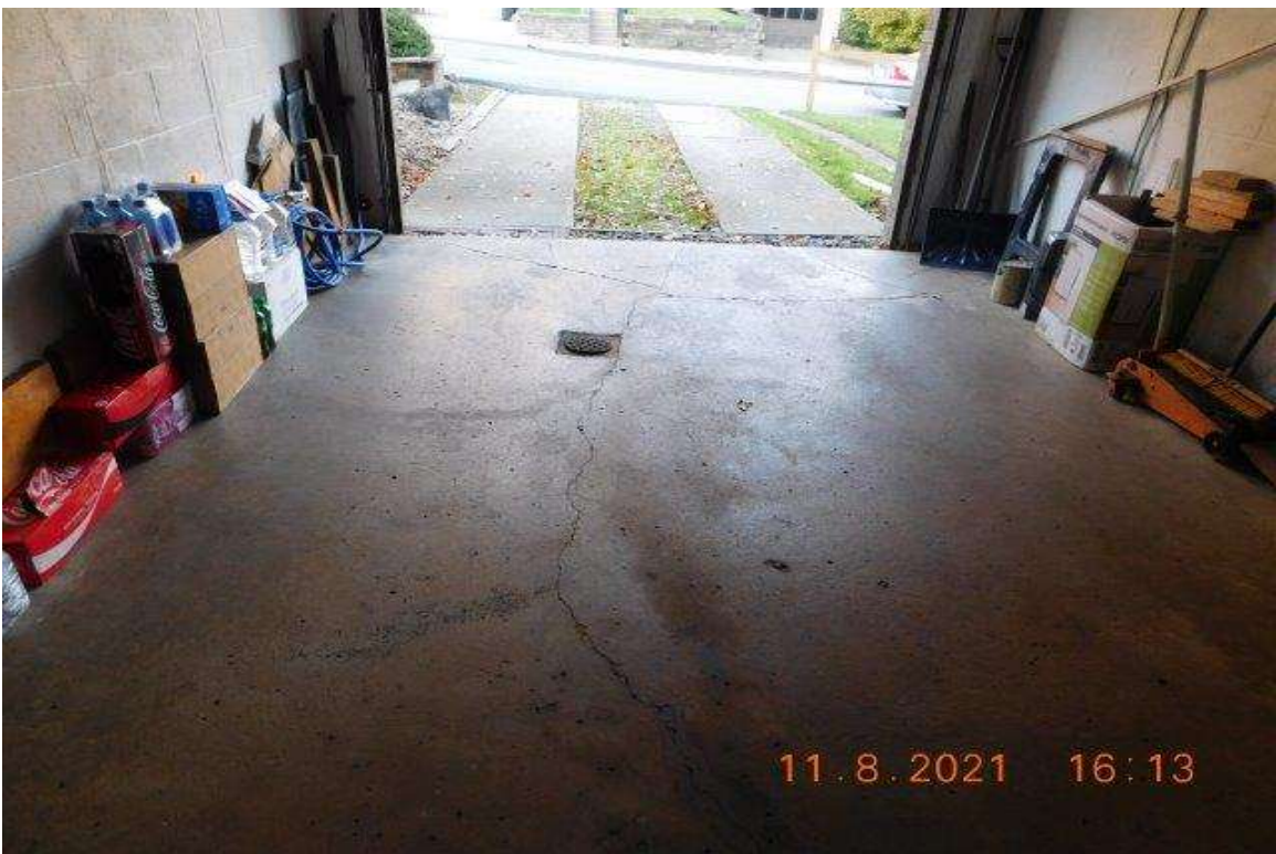
PHOTO 38 - GARAGE FLOOR LOOKING NORTH
