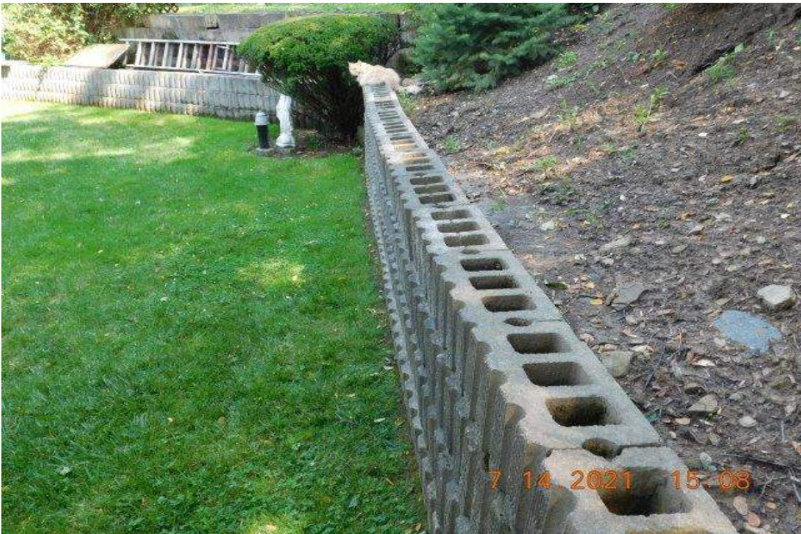
PHOTO 52 - CLOSE-UP OF AREA ON PHOTO 51
