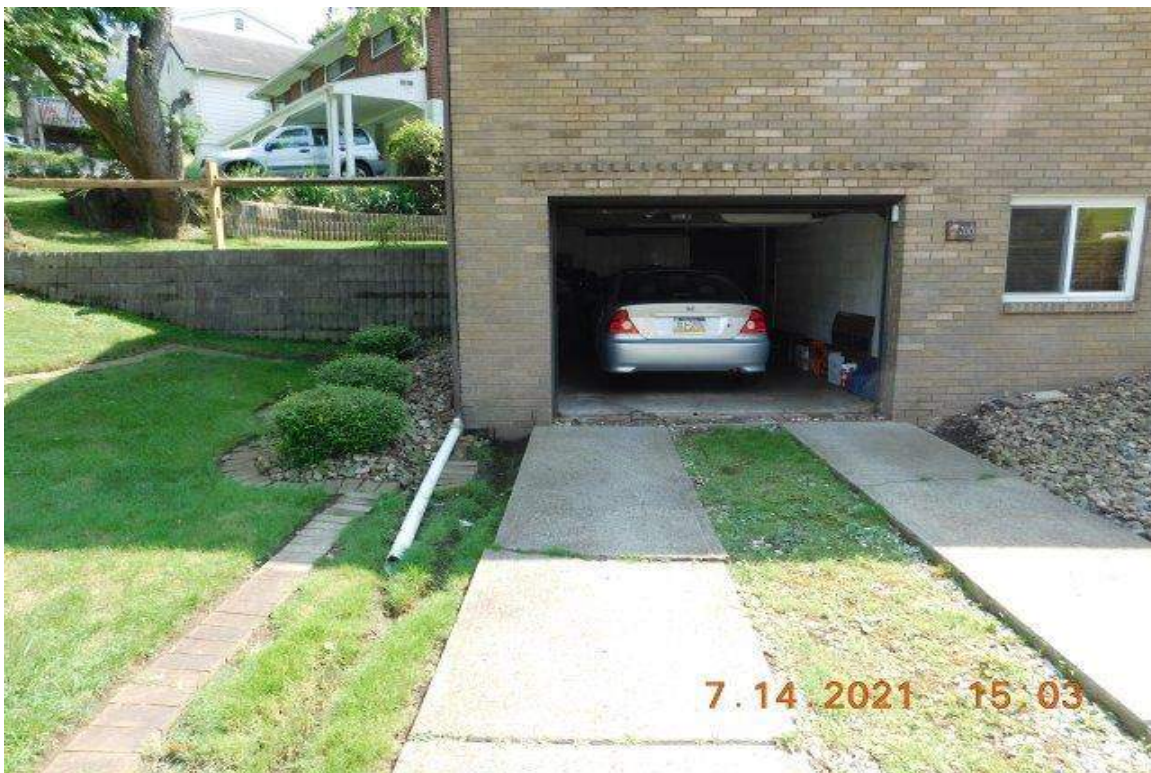
PHOTO 40 - DWELLING FRONT WALL GARAGE ENTRANCE
