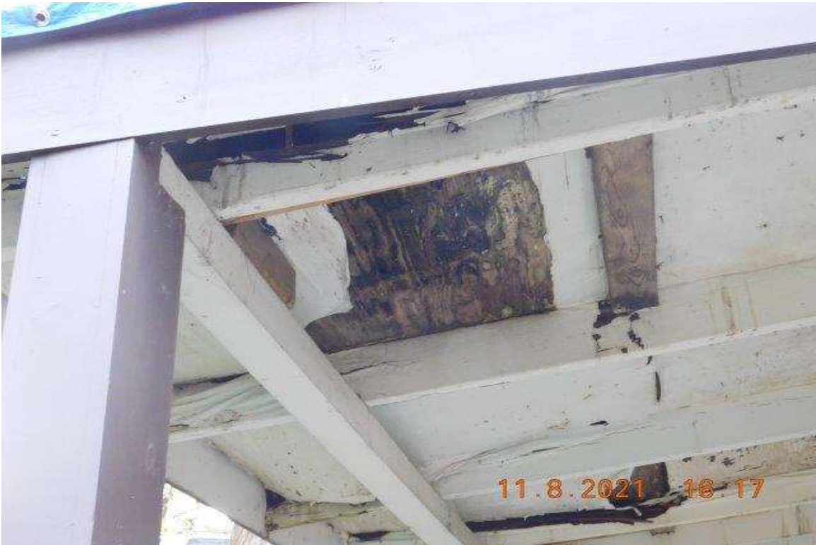
PHOTO 17 - CLOSE-UP OF AREA ON PHOTO 16
