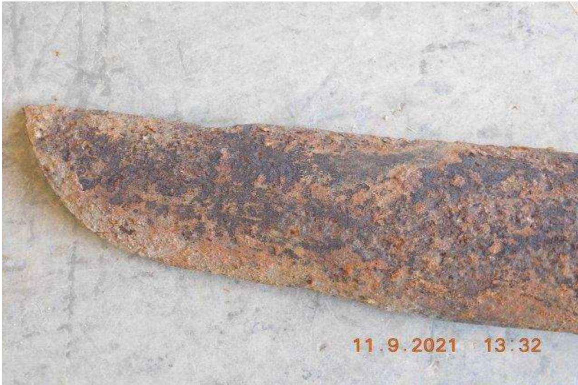
PHOTO 49 - AREA LEFT OF PHOTO 48
