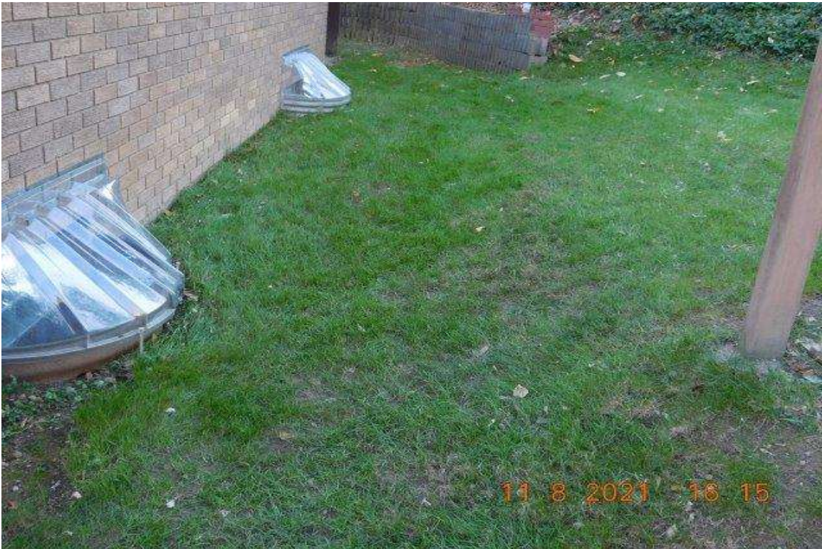
PHOTO 11 - CLOSE-UP OF AREA ON PHOTO 12
