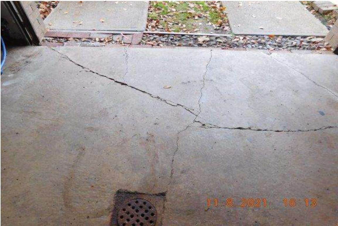
PHOTO 39 - CLOSE-UP OF AREA ON PHOTO 38
