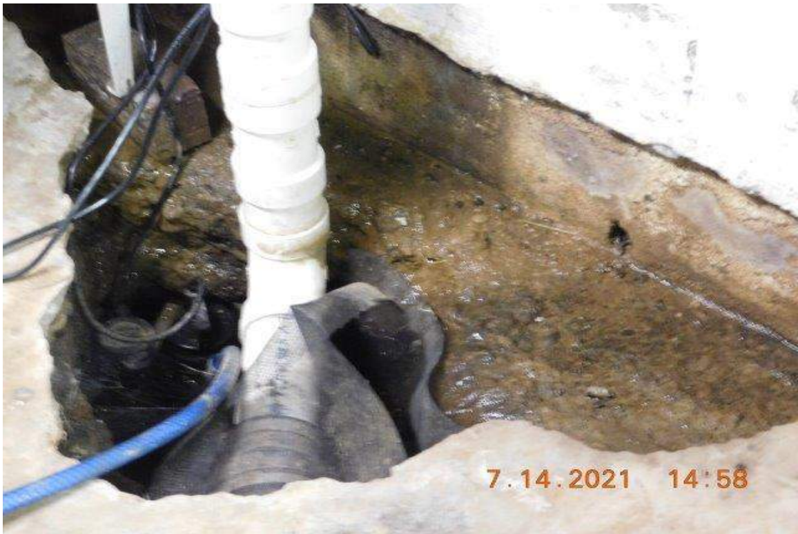
PHOTO 35 - CLOSE-UP OF AREA ON PHOTO 34
