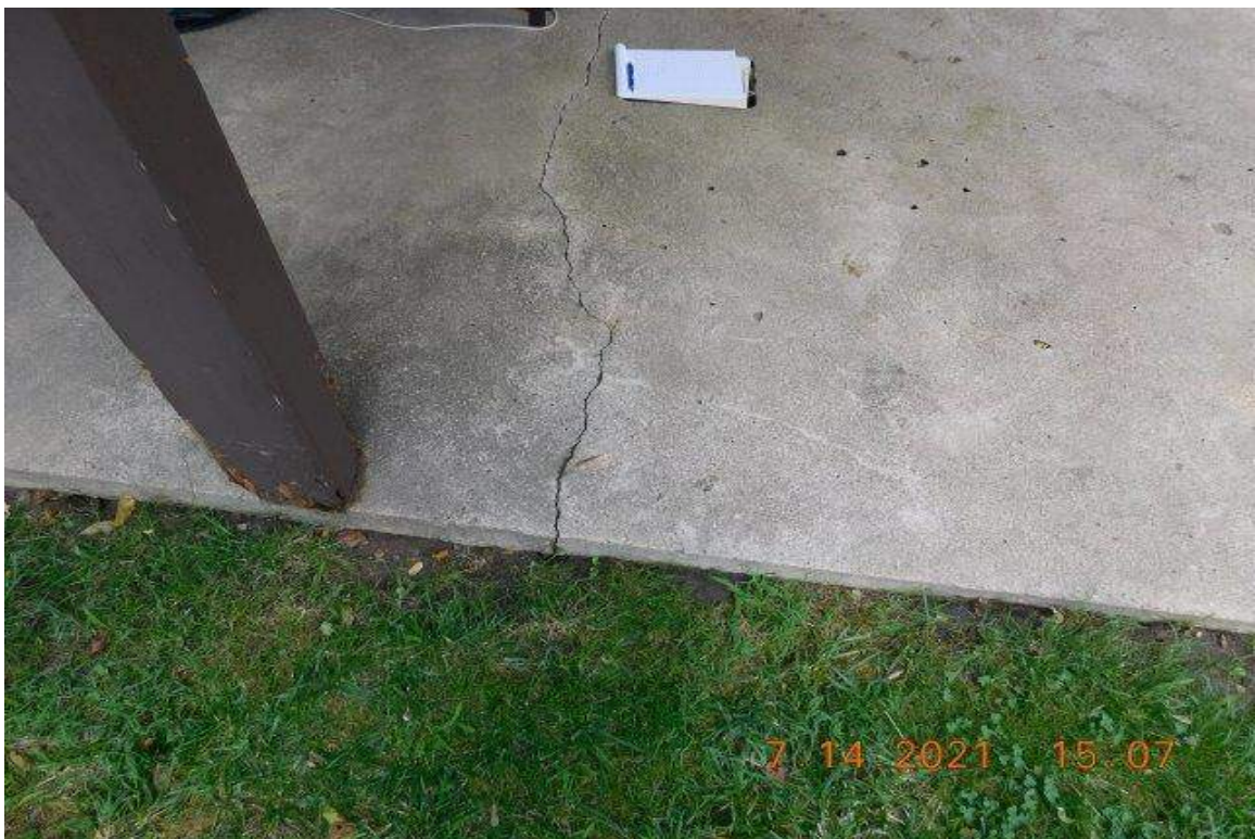
PHOTO 44 - CLOSE-UP OF AREA ON PHOTO 43
