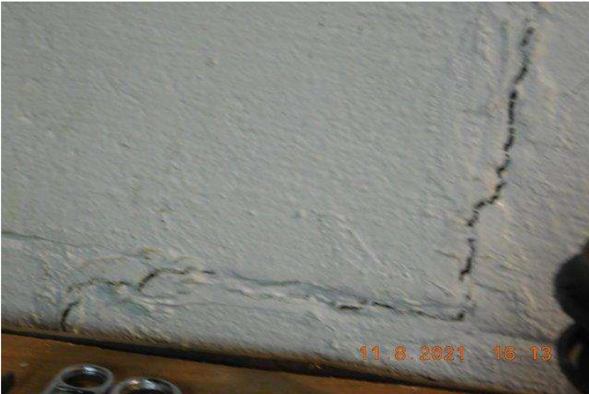
PHOTO 35 - AREA BELOW PHOTO 34
