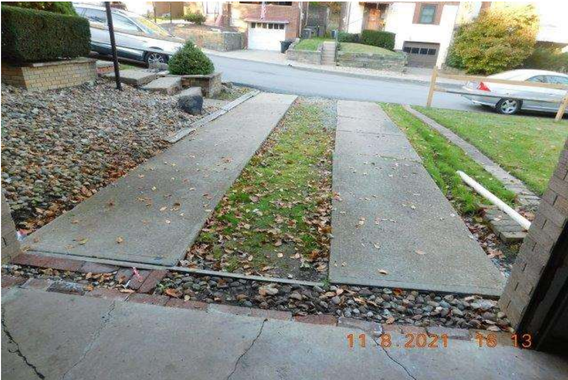
PHOTO 1 - DERIAN DRIVEWAY LOOKING NORTH
