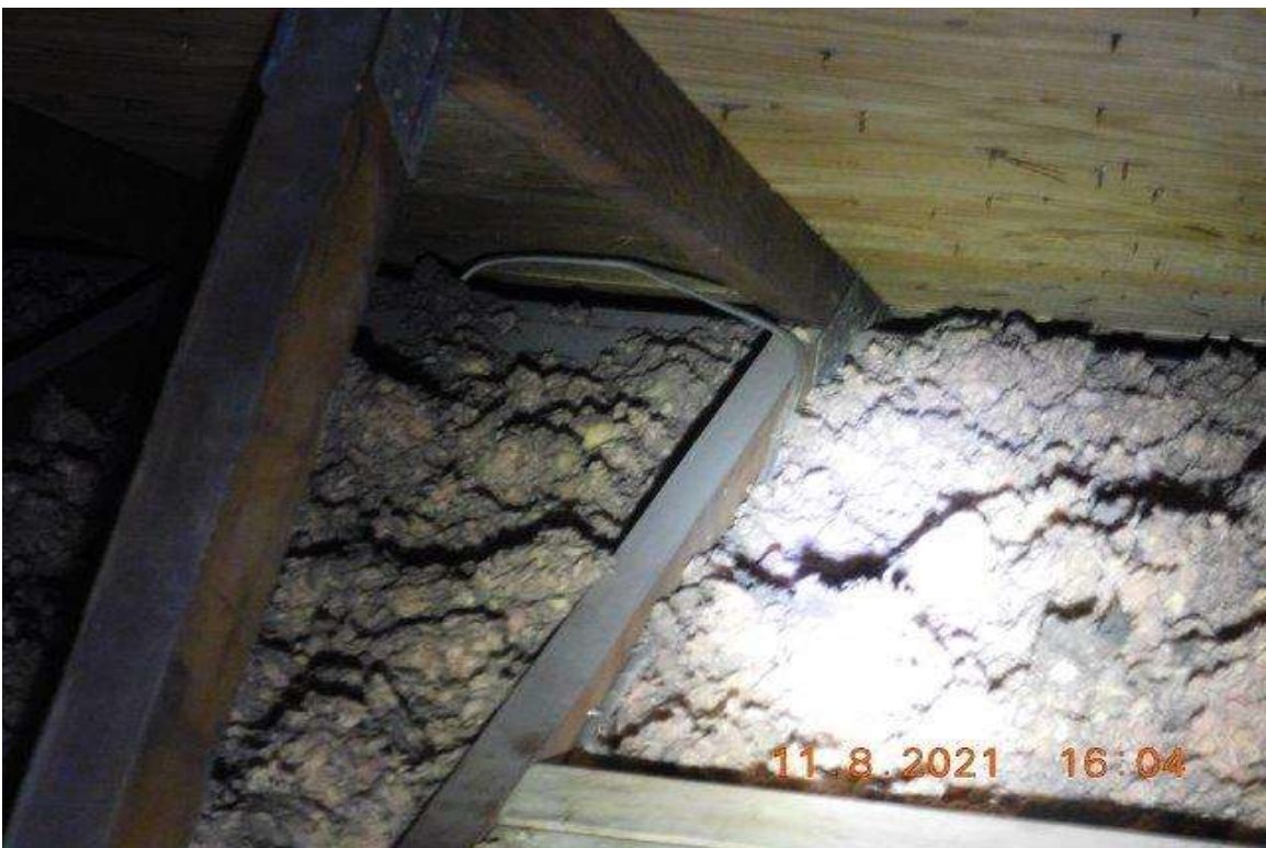
PHOTO 46 - CLOSE-UP OF AREA ON PHOTO 45
