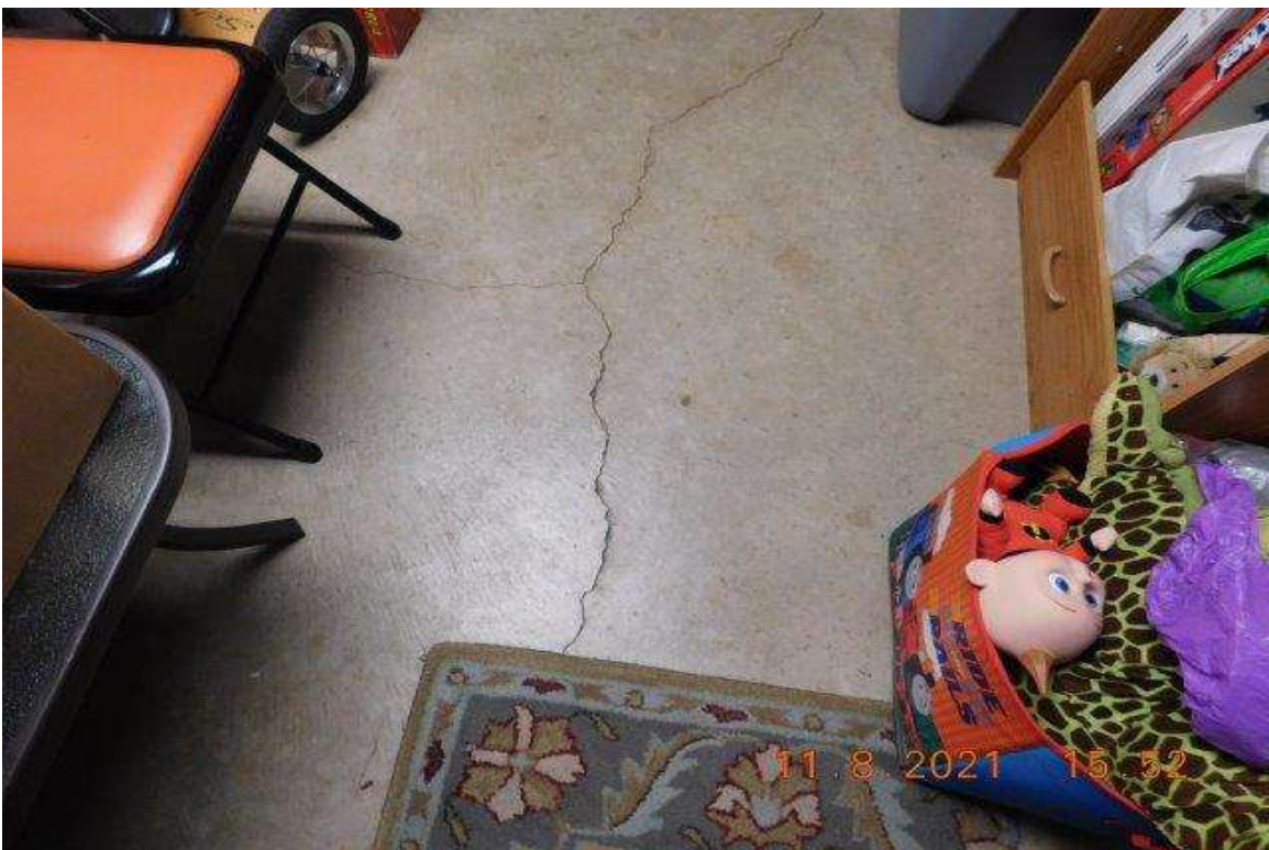
PHOTO 28 - CLOSE-UP OF AREA ON PHOTO 27
