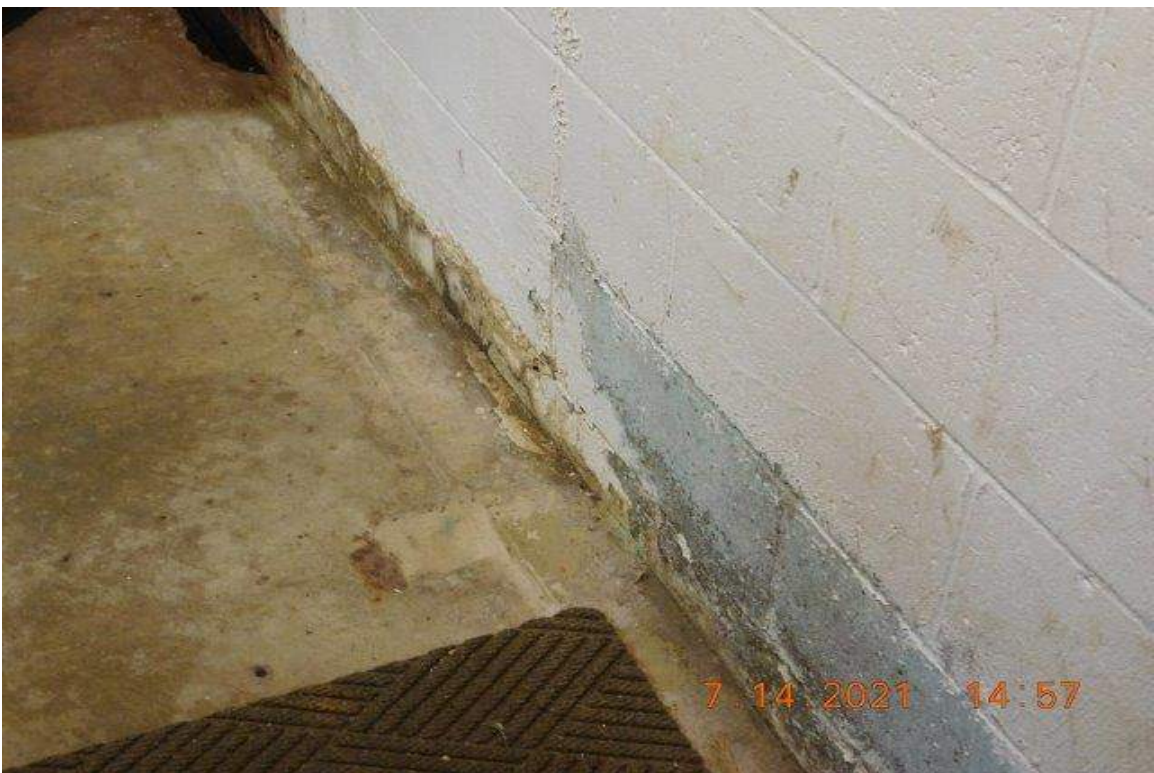
PHOTO 22 - AREA LEFT OF PHOTO 21
