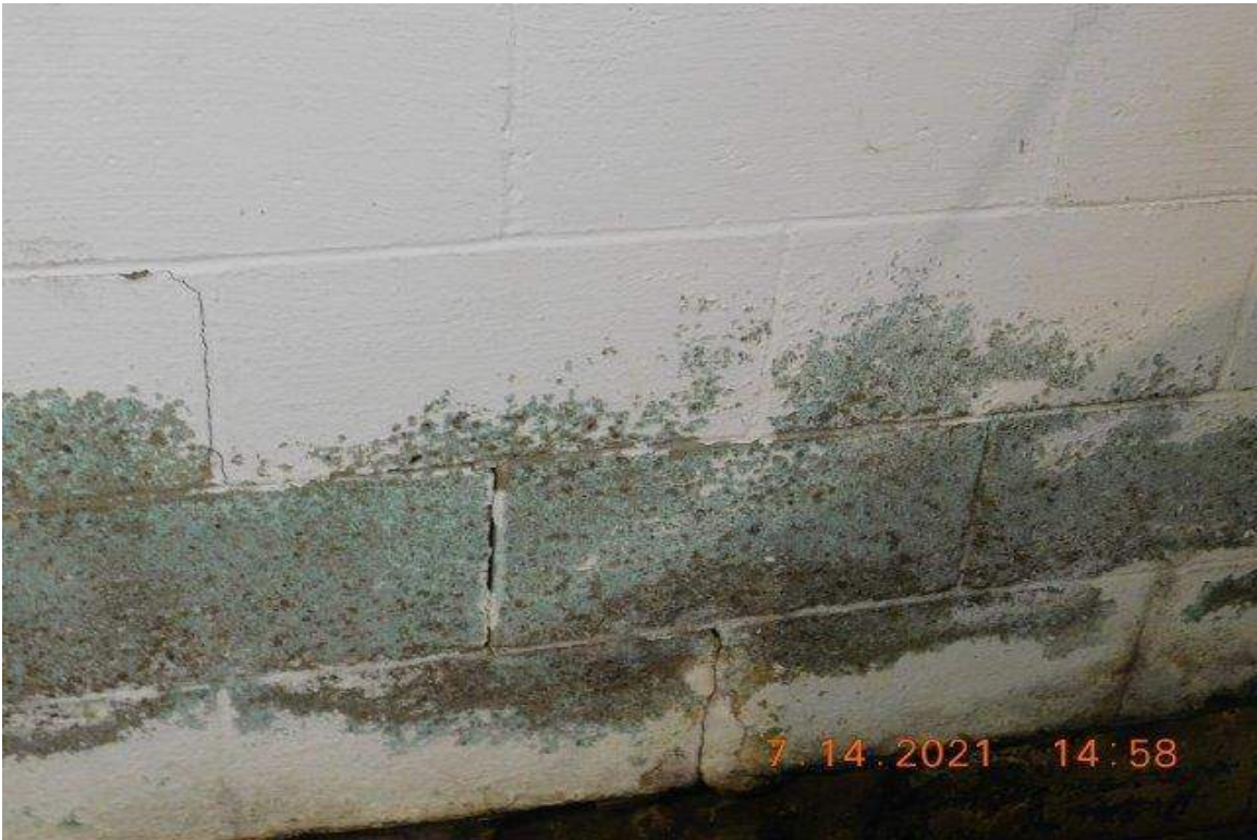
PHOTO 27 - AREA BELOW PHOTO 26
