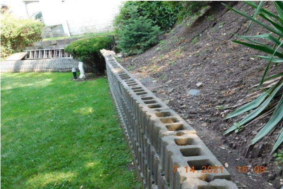
PHOTO 51 - REAR YARD RETAINING WALL LOOKING EAST
