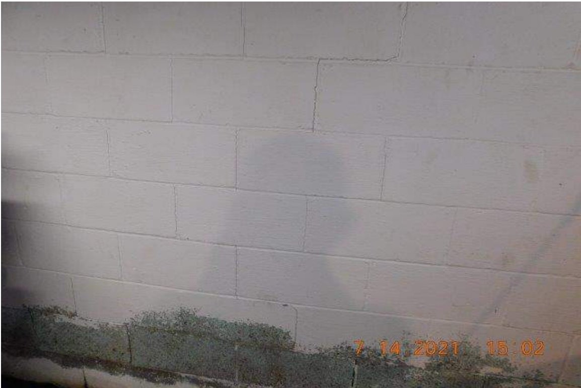
PHOTO 29 - AREA LEFT OF PHOTO 26
