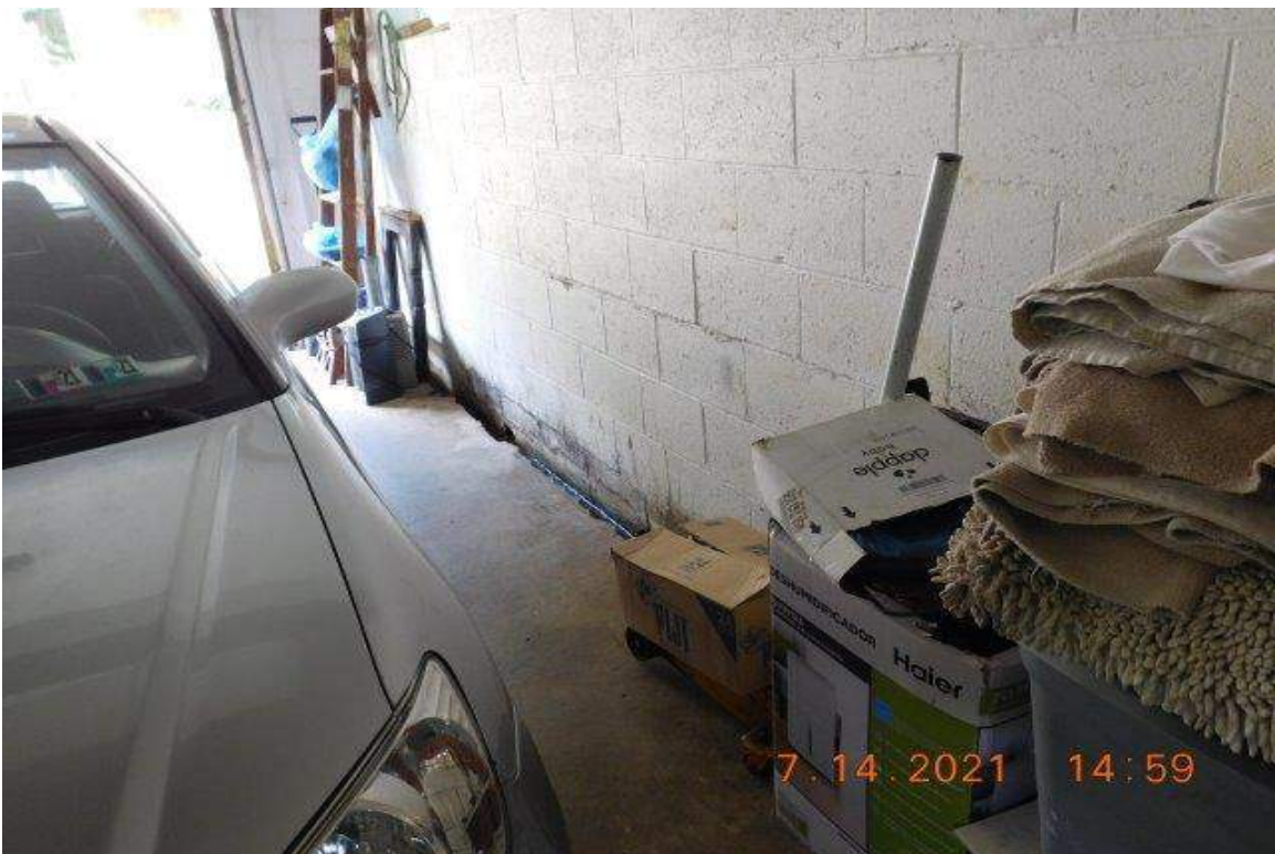
PHOTO 38 - GARAGE LEFT WALL
