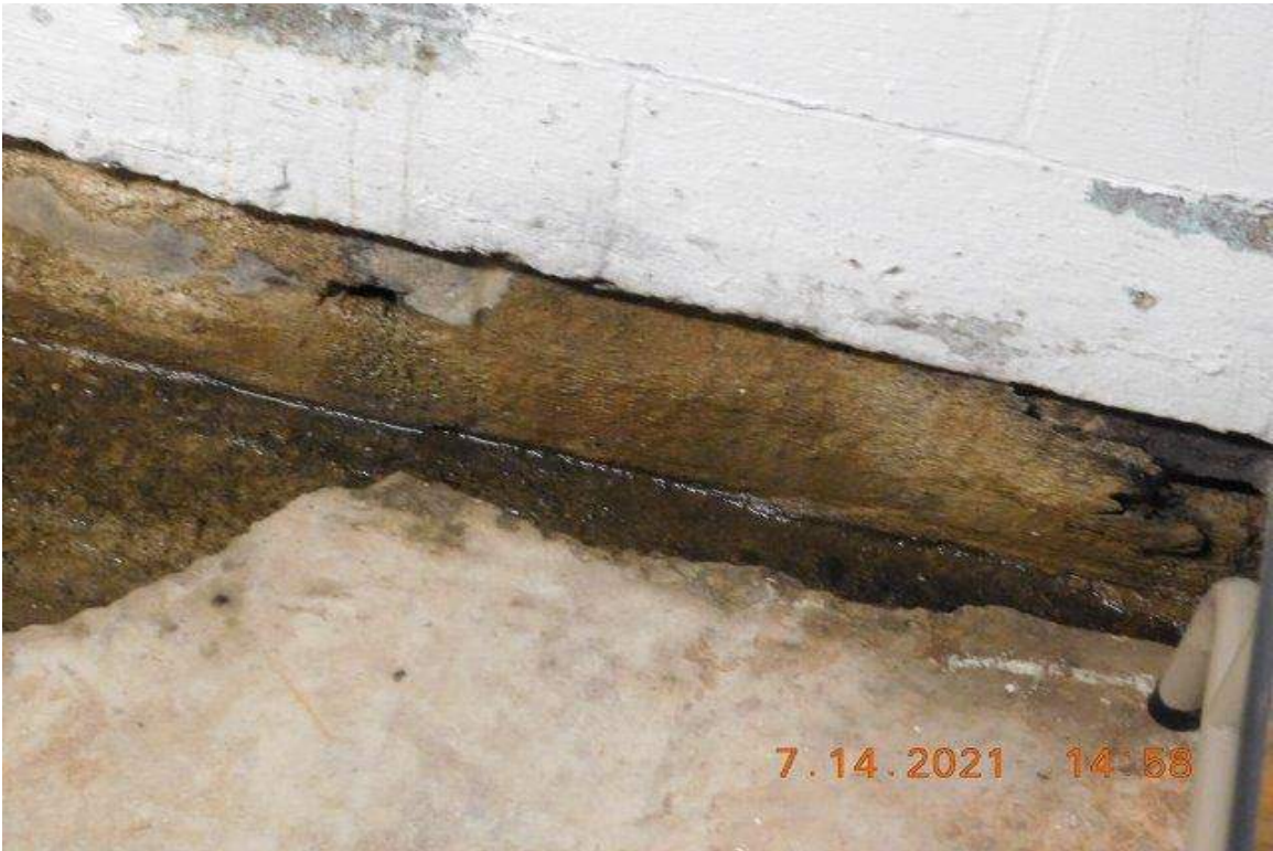
PHOTO 33 - AREA LEFT OF PHOTO 32
