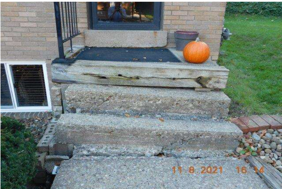
PHOTO 8 - CLOSE-UP OF AREA ON PHOTO 7
