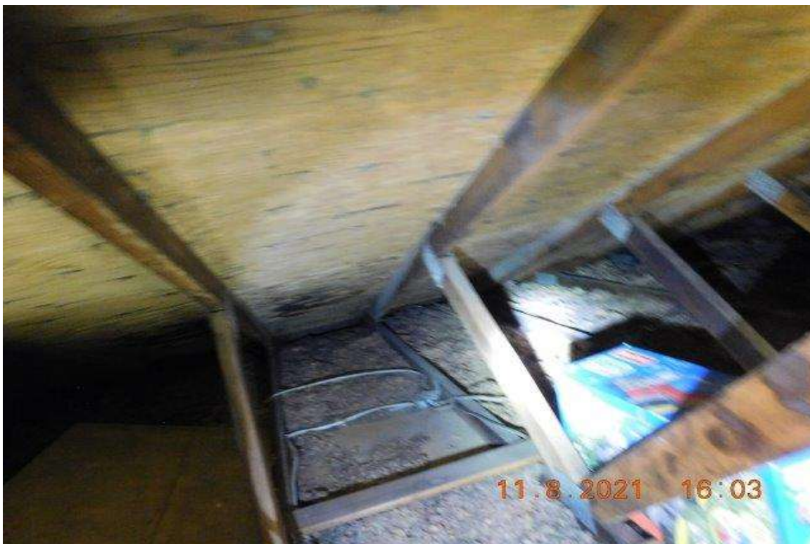
PHOTO 44 - ATTIC ROOF FRAMING
