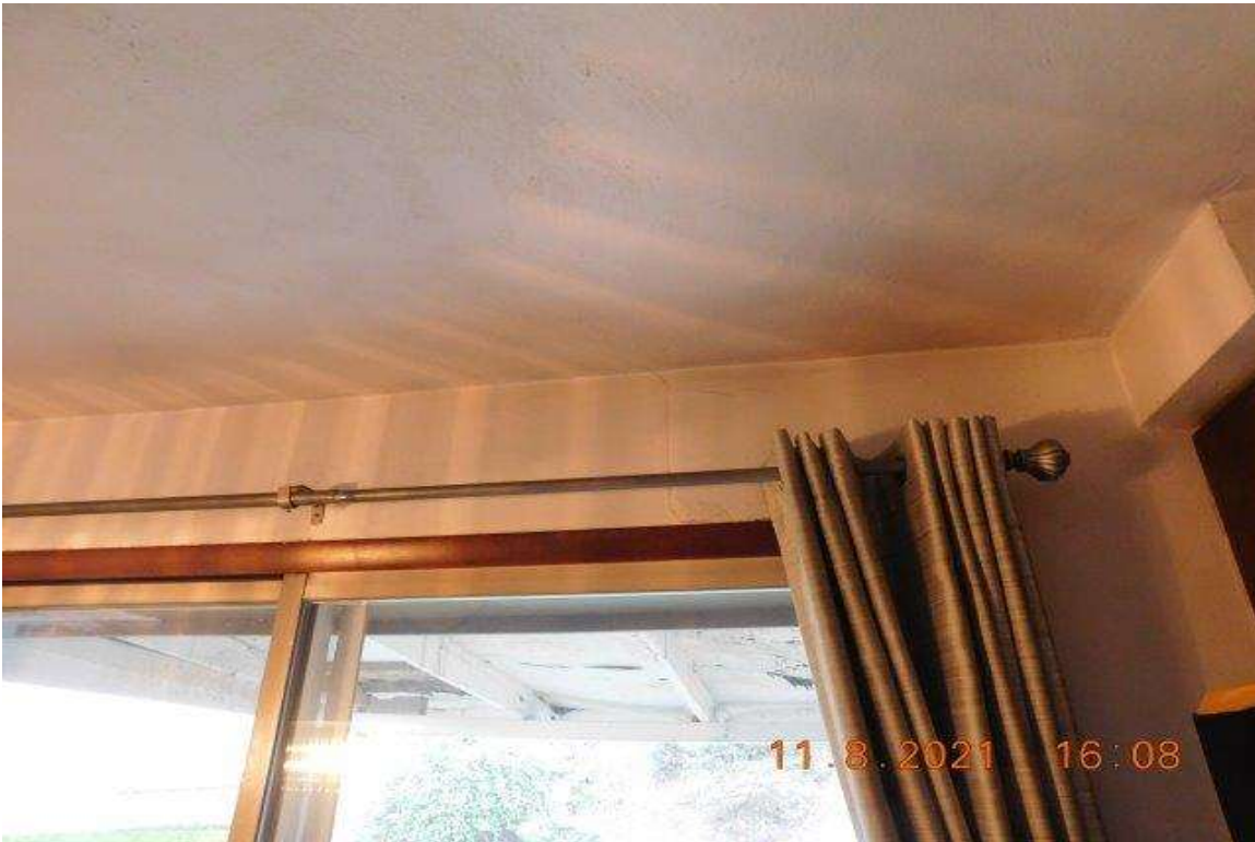
PHOTO 41 - AREA ABOVE REAR WALL EXIT TO PATIO
