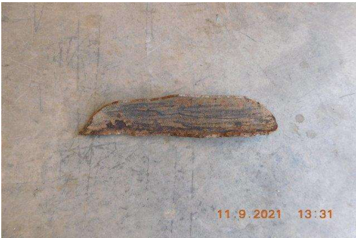
PHOTO 50 - INTERIOR FACE OF PIECE OF BROKEN WATER LINE
