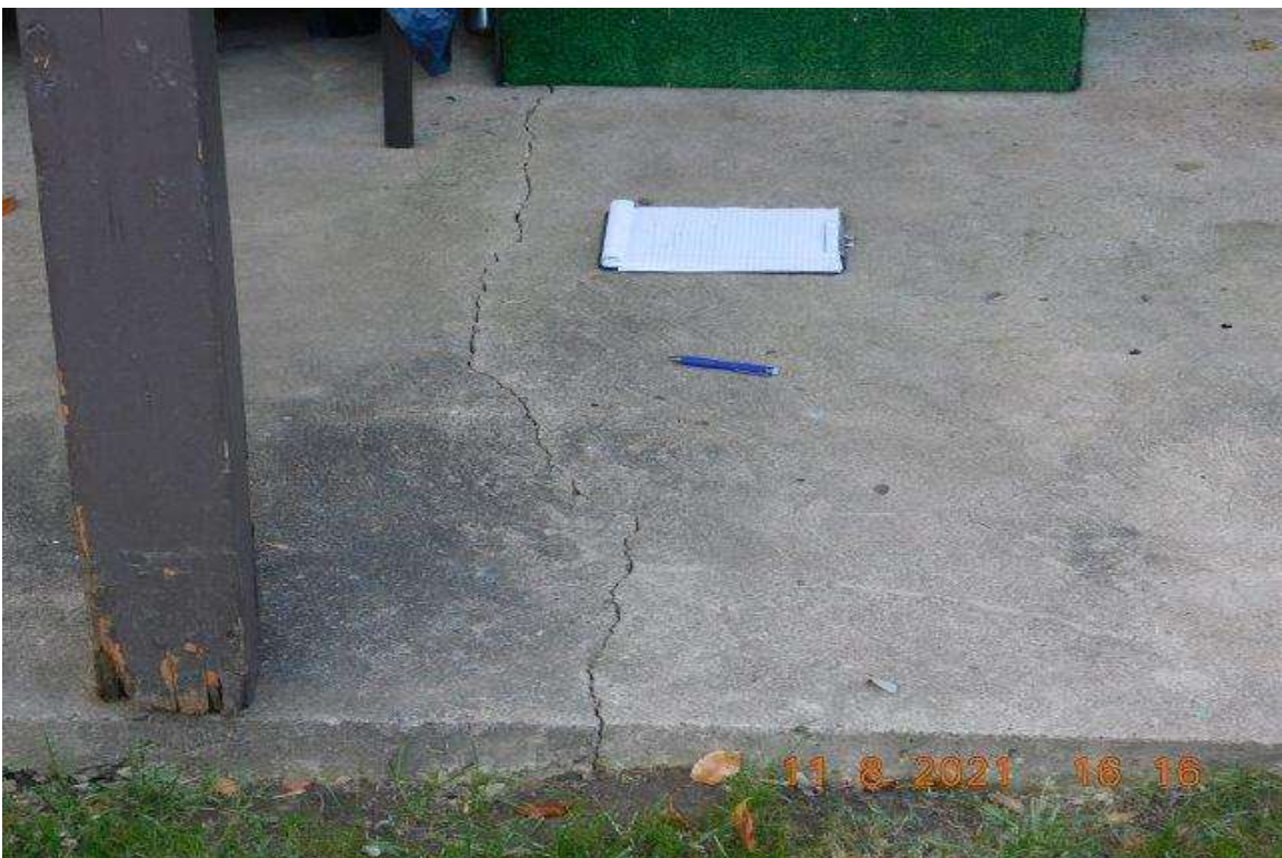
PHOTO 18 - REAR PATIO SLAB LOOKING NORTH
