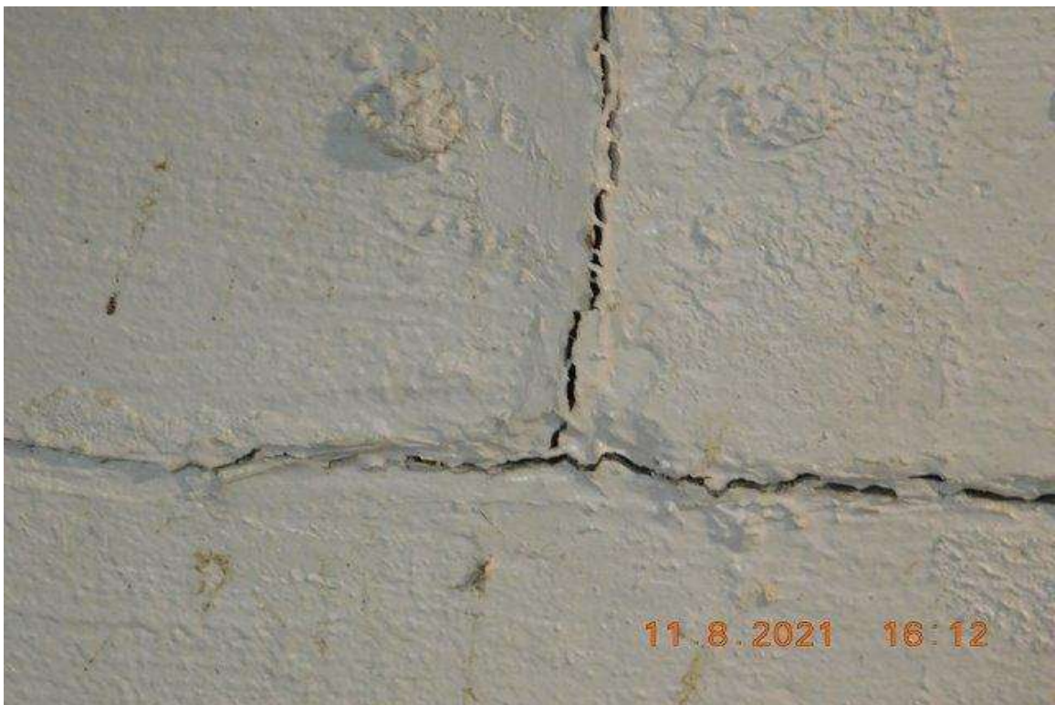
PHOTO 34 - CLOSE-UP OF AREA ON PHOTO 33
