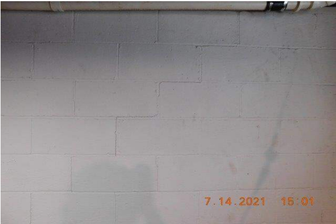
PHOTO 26 - AREA LEFT OF PHOTO 24
