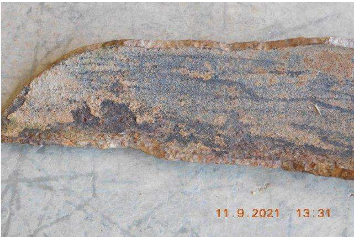
PHOTO 52 - AREA LEFT OF PHOTO 51
