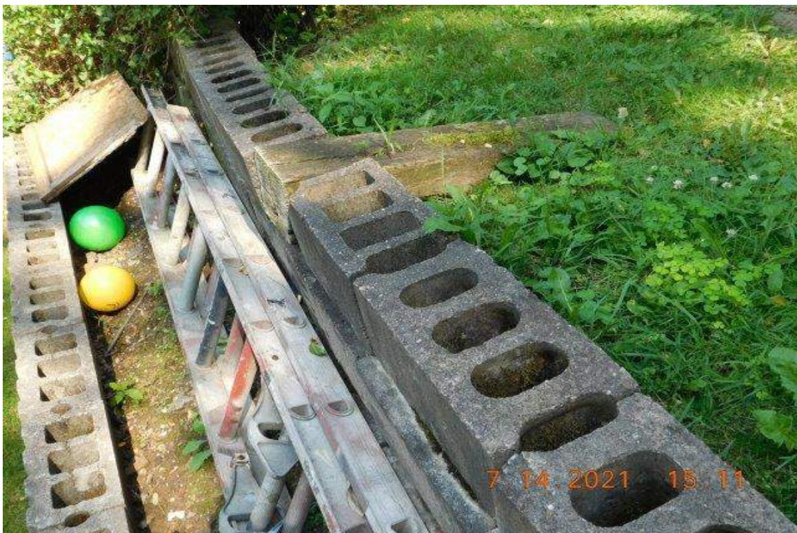
PHOTO 56 - UPPER LEFT YARD RETAINING WALL
