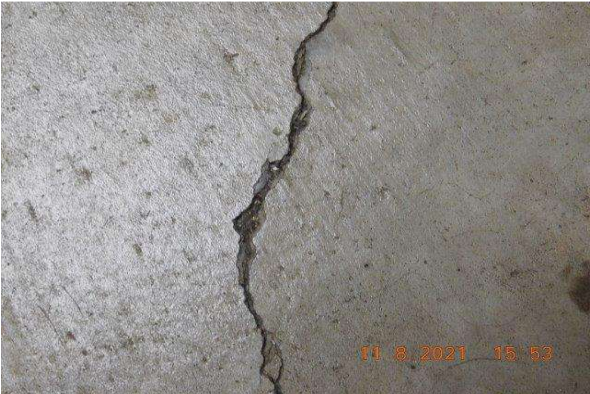
PHOTO 29 - CLOSE-UP OF AREA ON PHOTO 28
