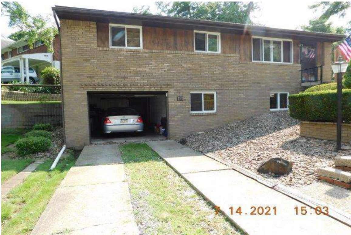
PHOTO 9 - DERIAN DWELLING FRONT (NORTH) WALL
