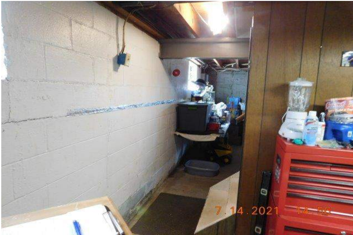
PHOTO 11 - BASEMENT RIGHT WALL RIGHT OF PHOTO 10
