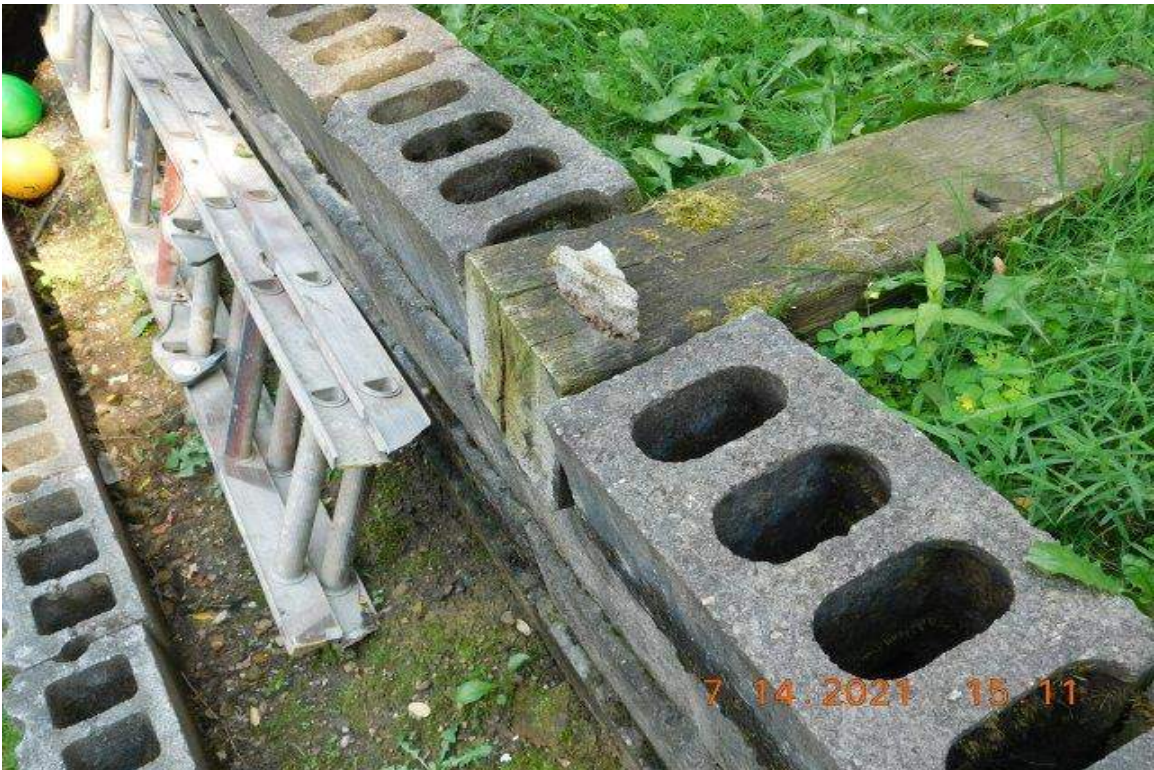
PHOTO 58 - CLOSE-UP OF AREA ON PHOTO 57
