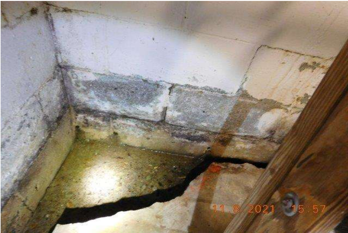
PHOTO 37 - CLOSE-UP OF AREA ON PHOTO 36
