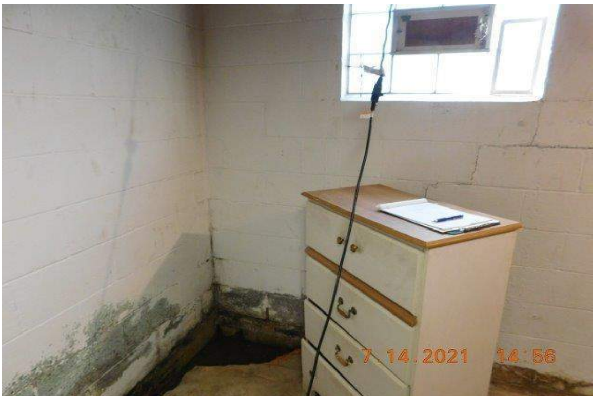
PHOTO 10 - RIGHT (WEST) REAR CORNER OF BASEMENT
