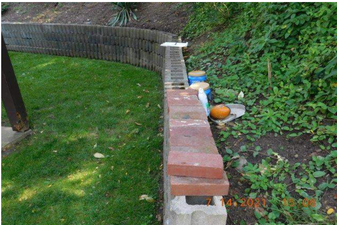
PHOTO 50 - RETAINING WALL IN REAR PORTION OF RIGHT YARD
