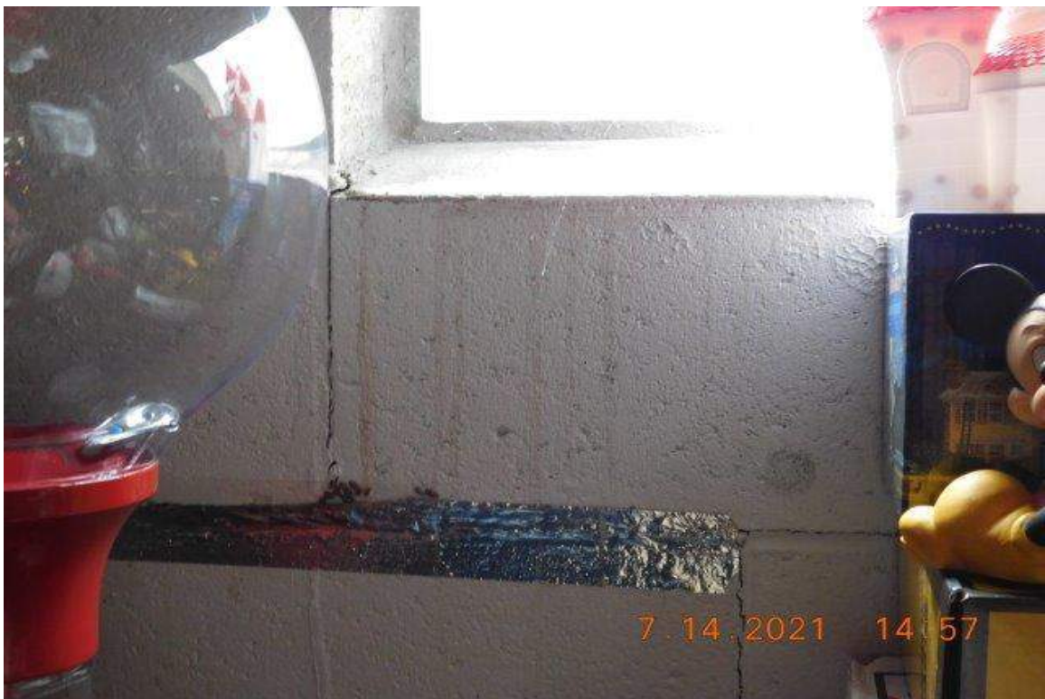
PHOTO 18 - BASEMENT RIGHT WALL FRONT WINDOW
