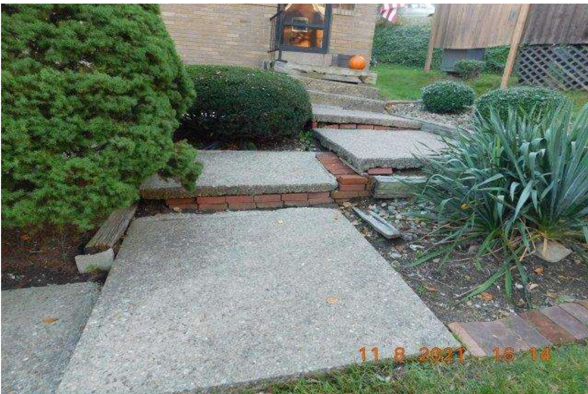
PHOTO 6 - SIDEWALK WEST OF PHOTO 5
