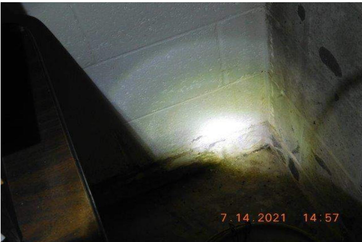
PHOTO 20 - BASEMENT RIGHT FRONT CORNER
