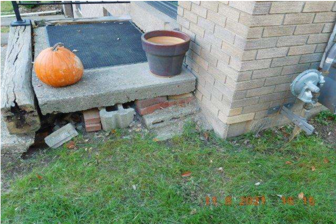
PHOTO 9 - FRONT ENTRY STOOP LOOKING EAST
