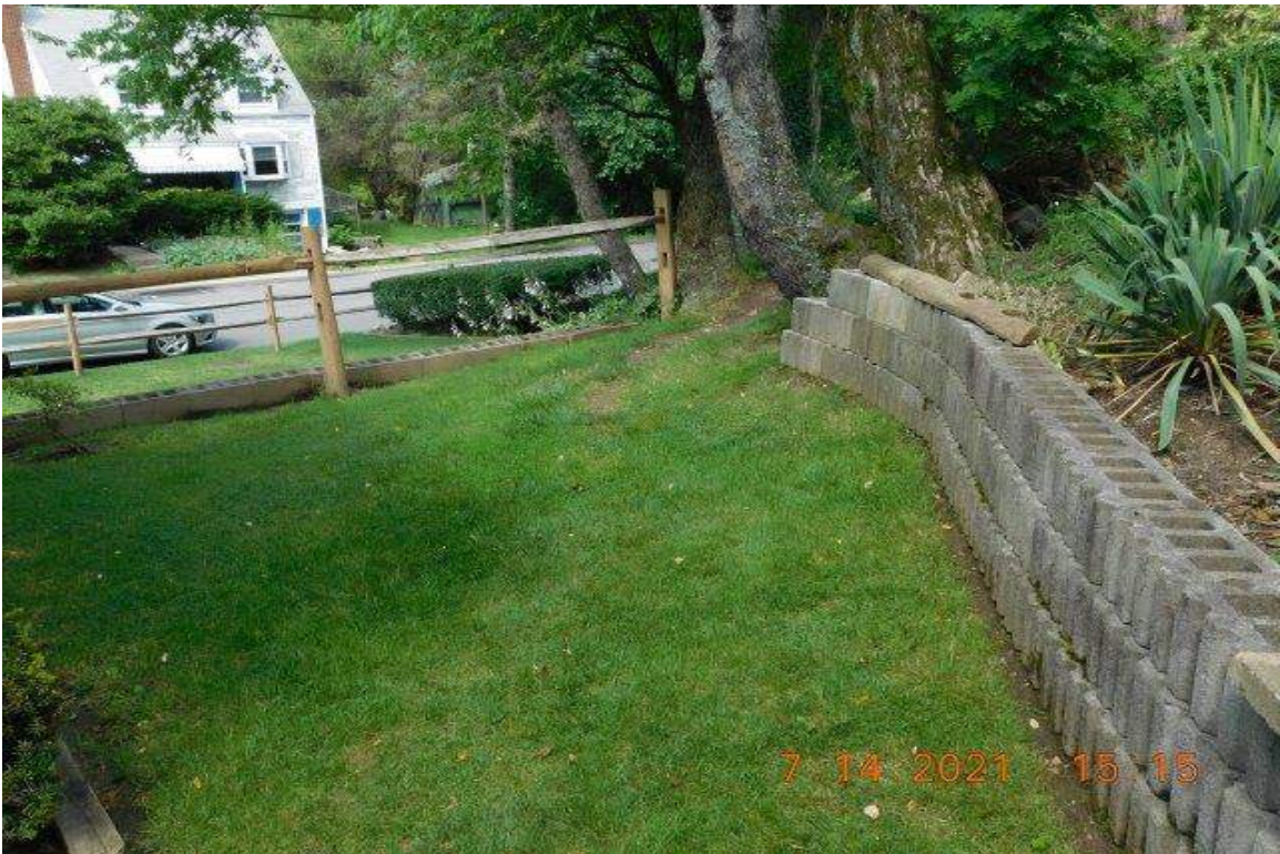
PHOTO 60 - FRONT PORTION OF LOWER LEFT YARD RETAINING WALL
