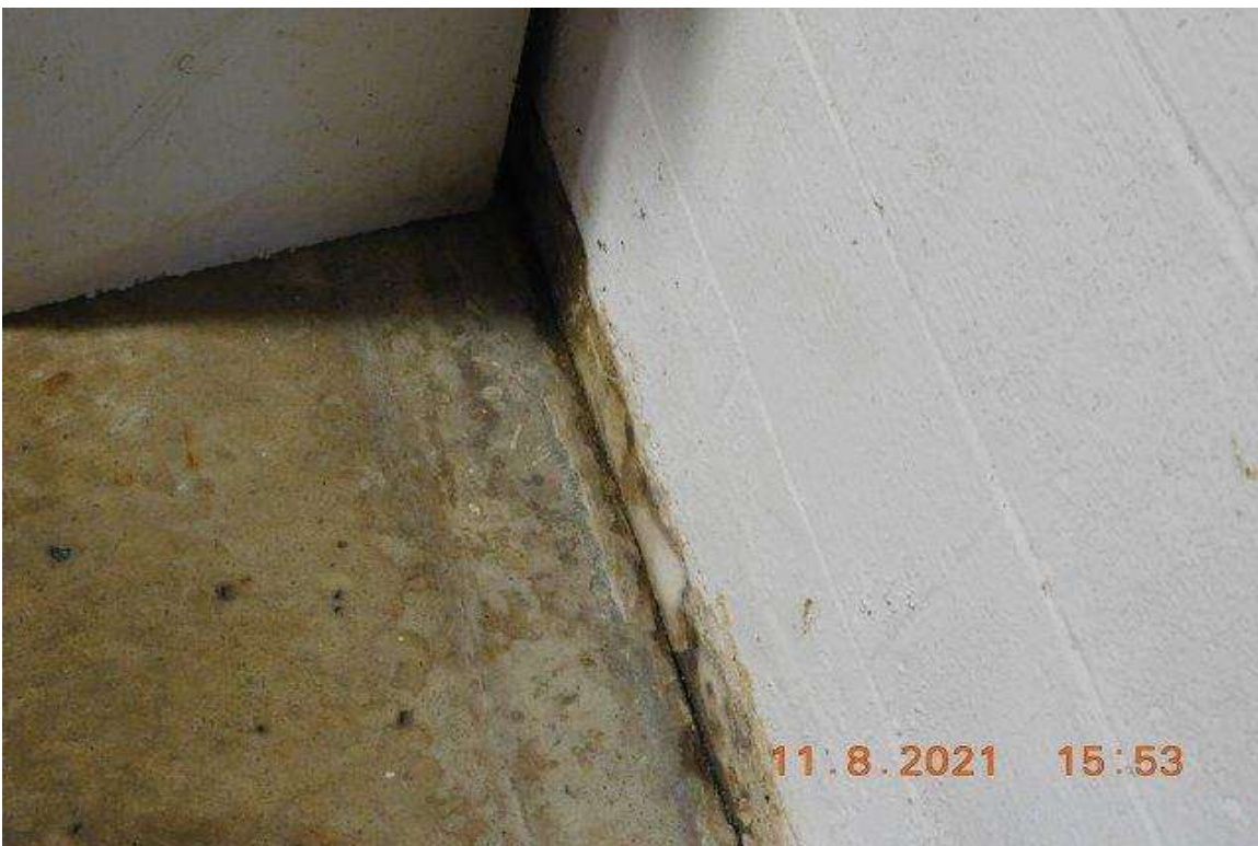
PHOTO 32 - CLOSE-UP OF AREA ON PHOTO 31
