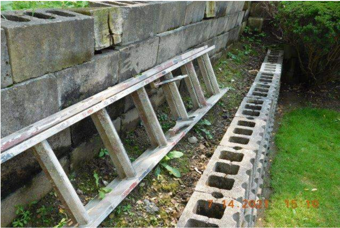
PHOTO 57 - REAR PORTION OF UPPER LEFT YARD RETAINING WALL LOOKING SOUTH
