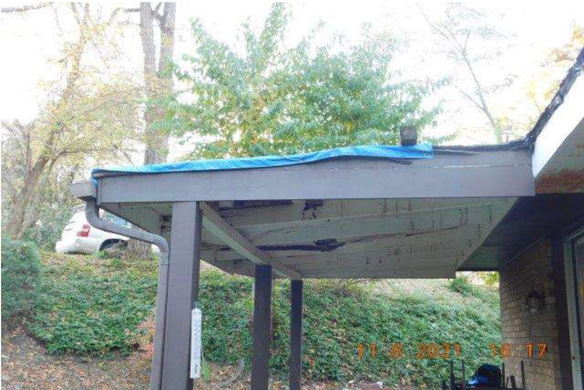
PHOTO 16 - REAR PATIO ROOF LOOKING WEST
