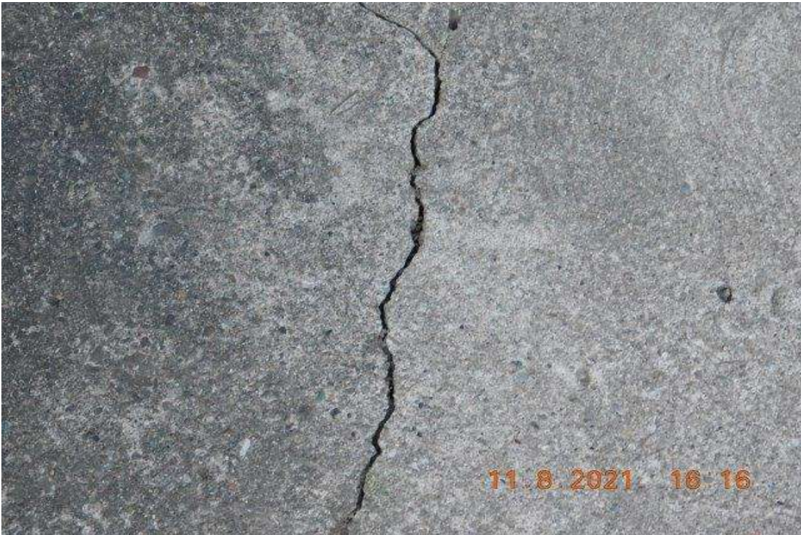
PHOTO 19 - CLOSE-UP OF AREA ON PHOTO 18
