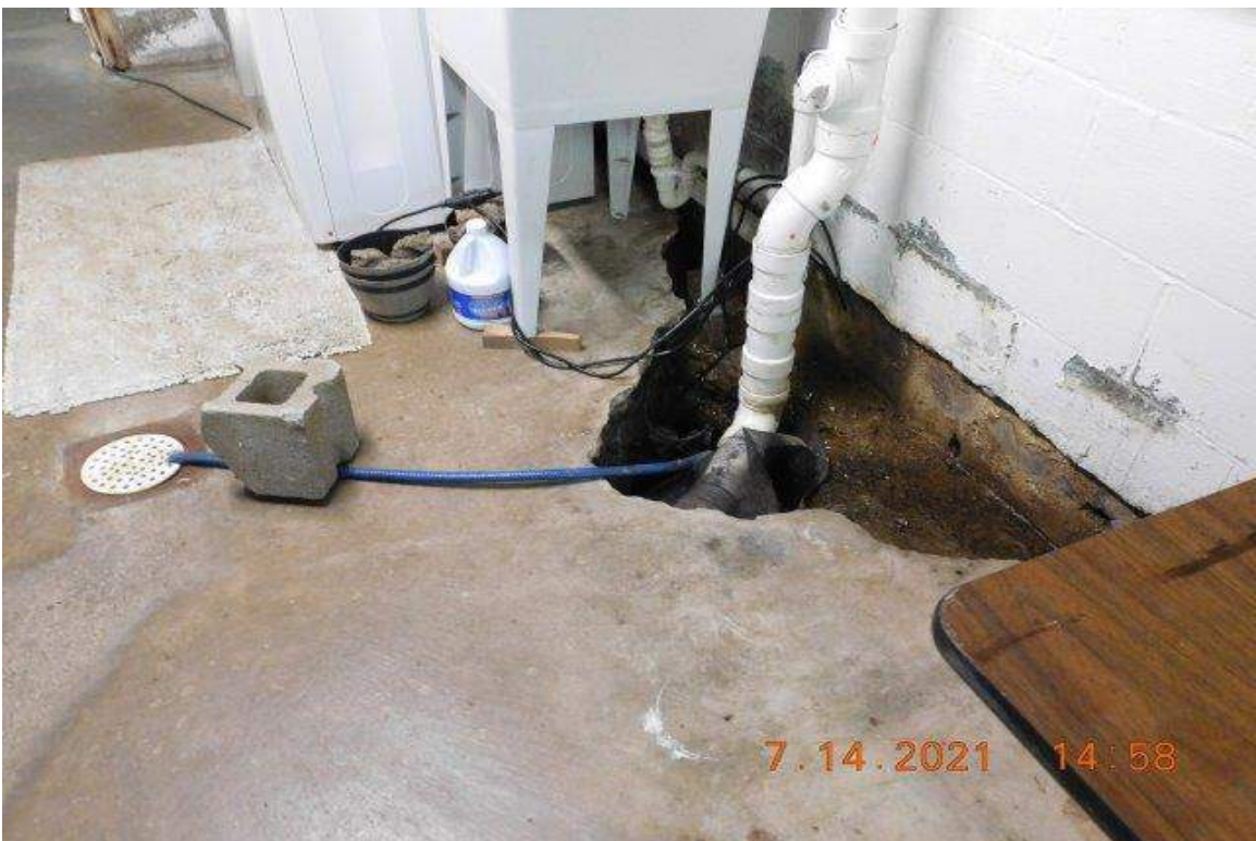
PHOTO 34 - LEFT REAR PORTION OF BASEMENT
