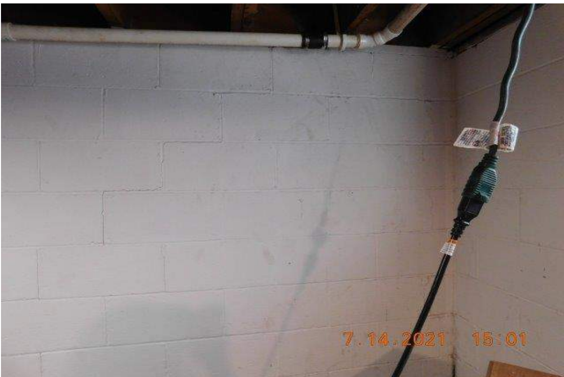
PHOTO 24 - RIGHT REAR CORNER OF BASEMENT
