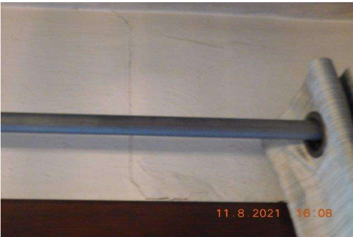
PHOTO 42 - CLOSE-UP OF AREA ON PHOTO 41
