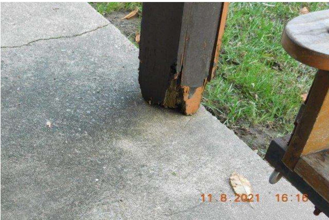
PHOTO 14 - CLOSE-UP OF REAR PATIO CENTER ROOF SUPPORT POST
