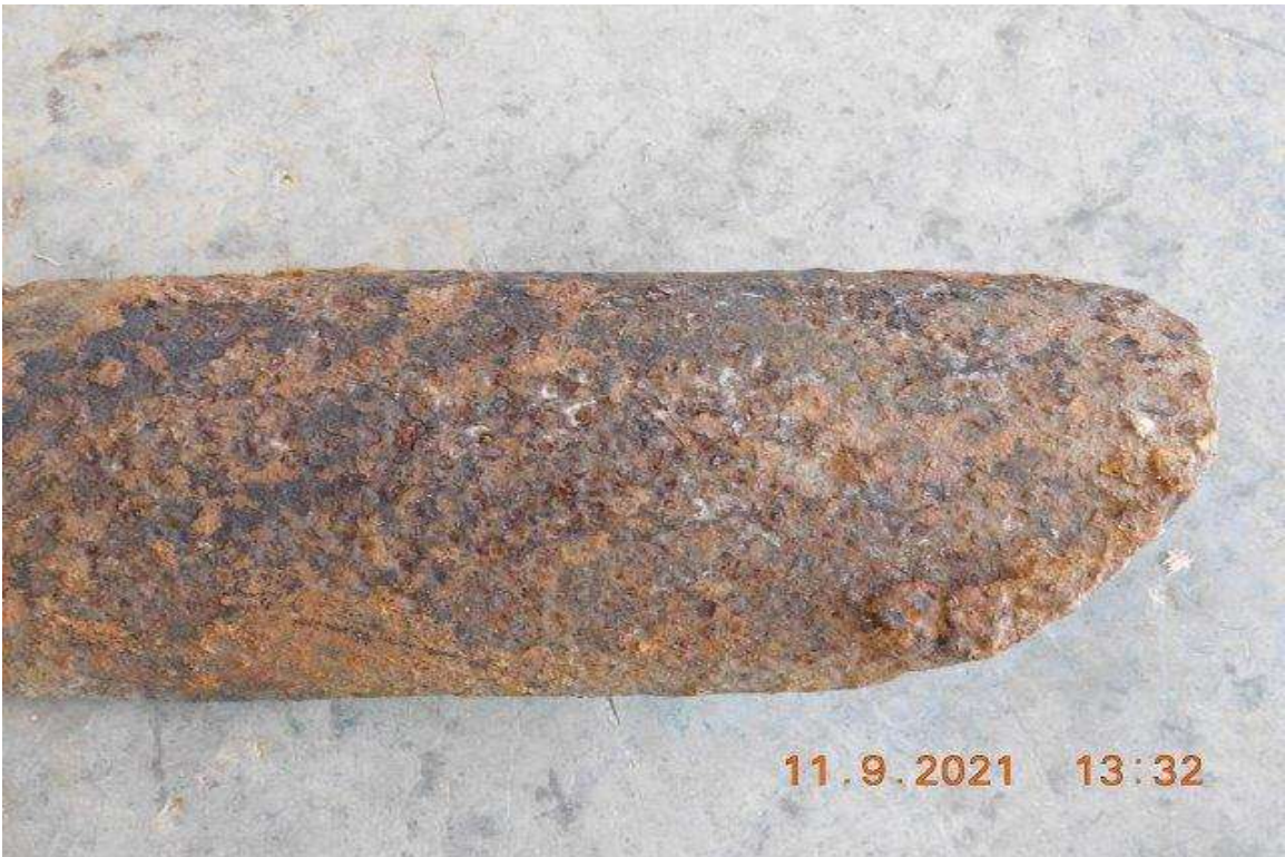
PHOTO 48 - CLOSE-UP OF AREA ON PHOTO 47
