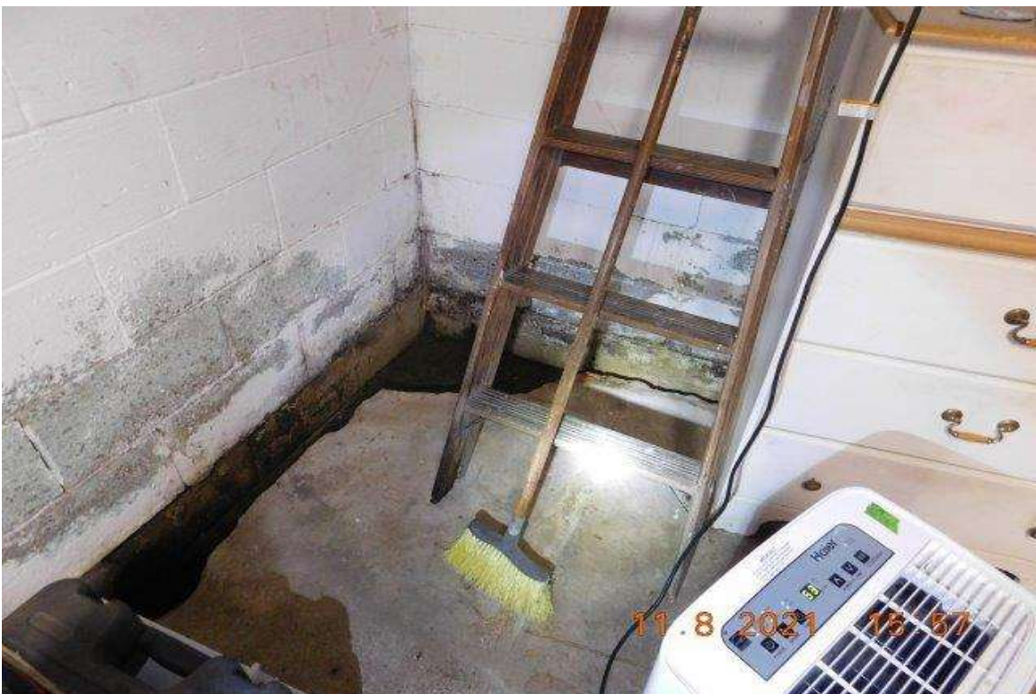
PHOTO 36 - RIGHT REAR CORNER OF BASEMENT REAR ROOM
