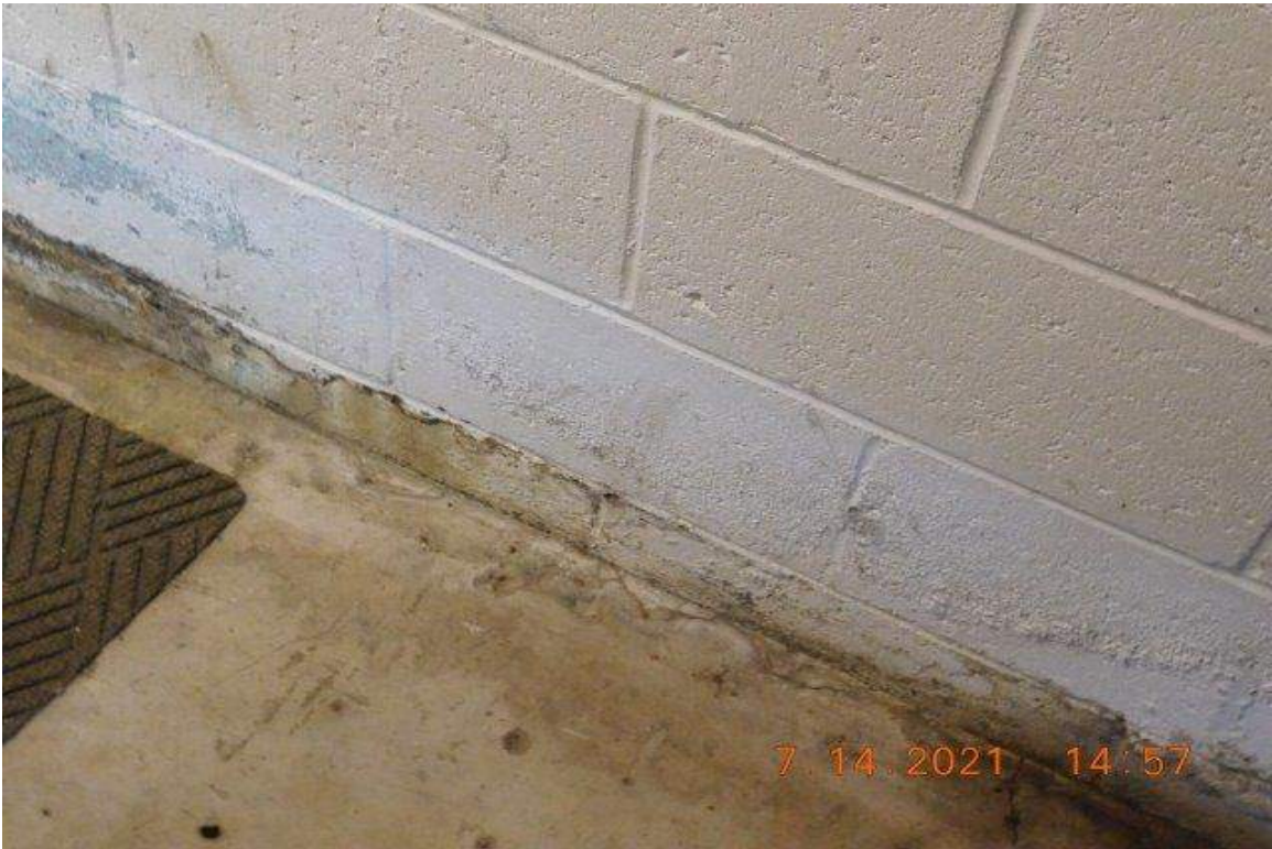
PHOTO 21 - CENTER OF BASEMENT RIGHT WALL AT FLOOR
