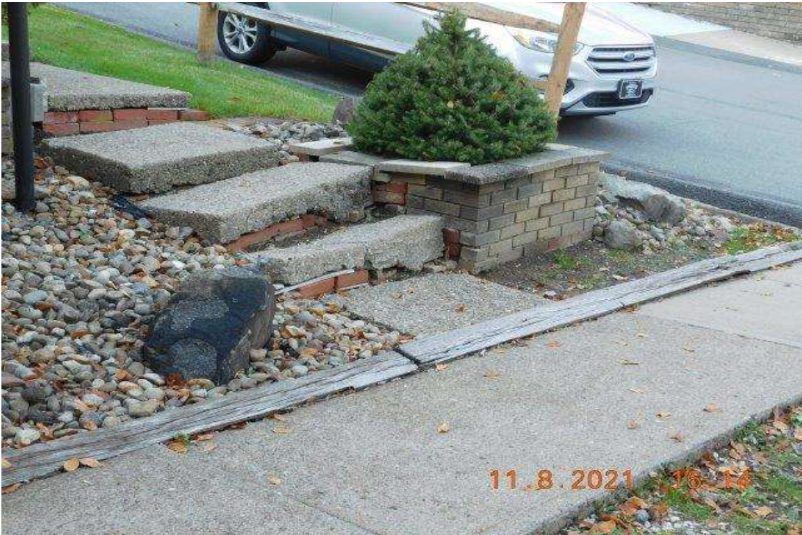
PHOTO 3 - FRONT (NORTH) YARD SIDEWALK LOOKING NORTHWEST
