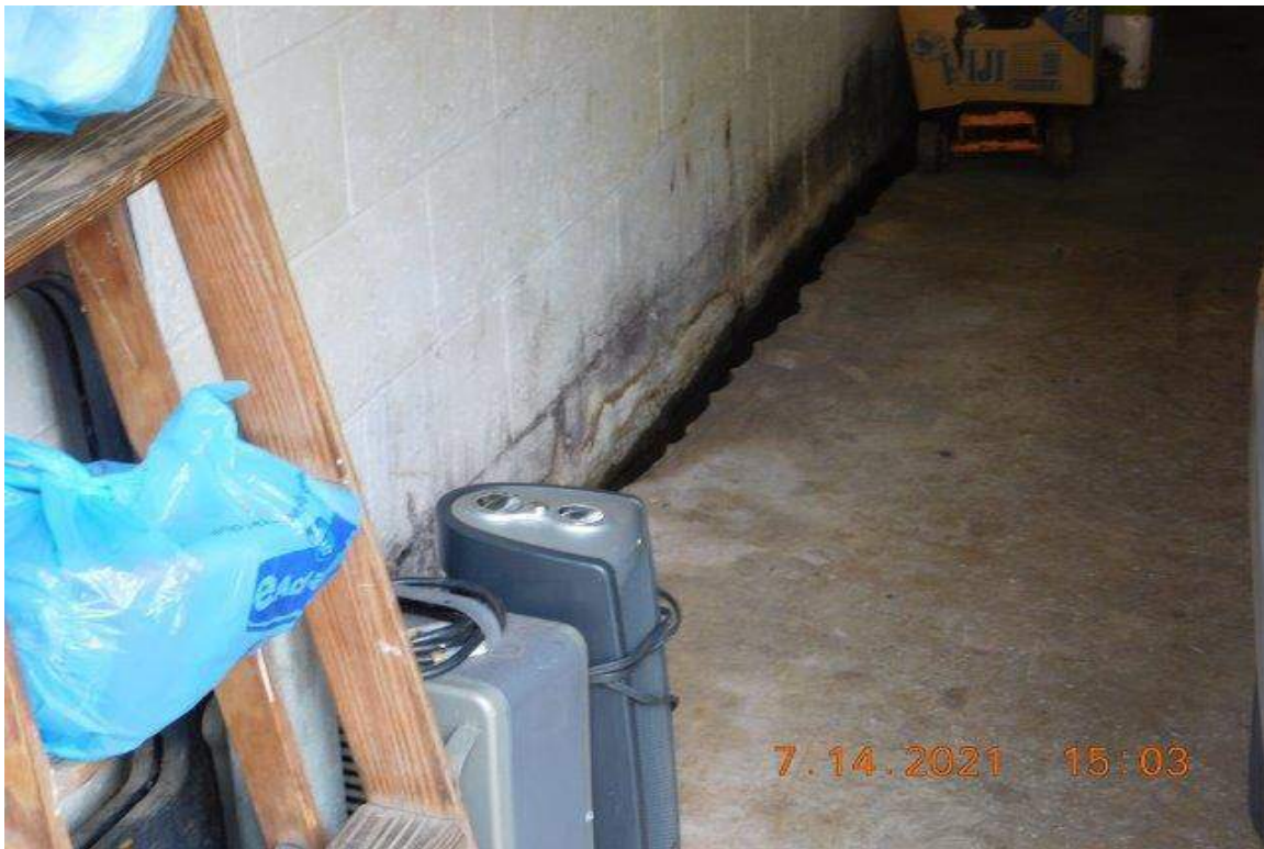
PHOTO 39 - CLOSE-UP OF GARAGE LEFT WALL
