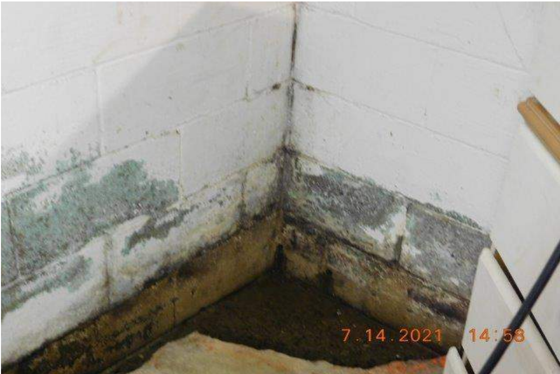
PHOTO 25 - AREA BELOW PHOTO 24
