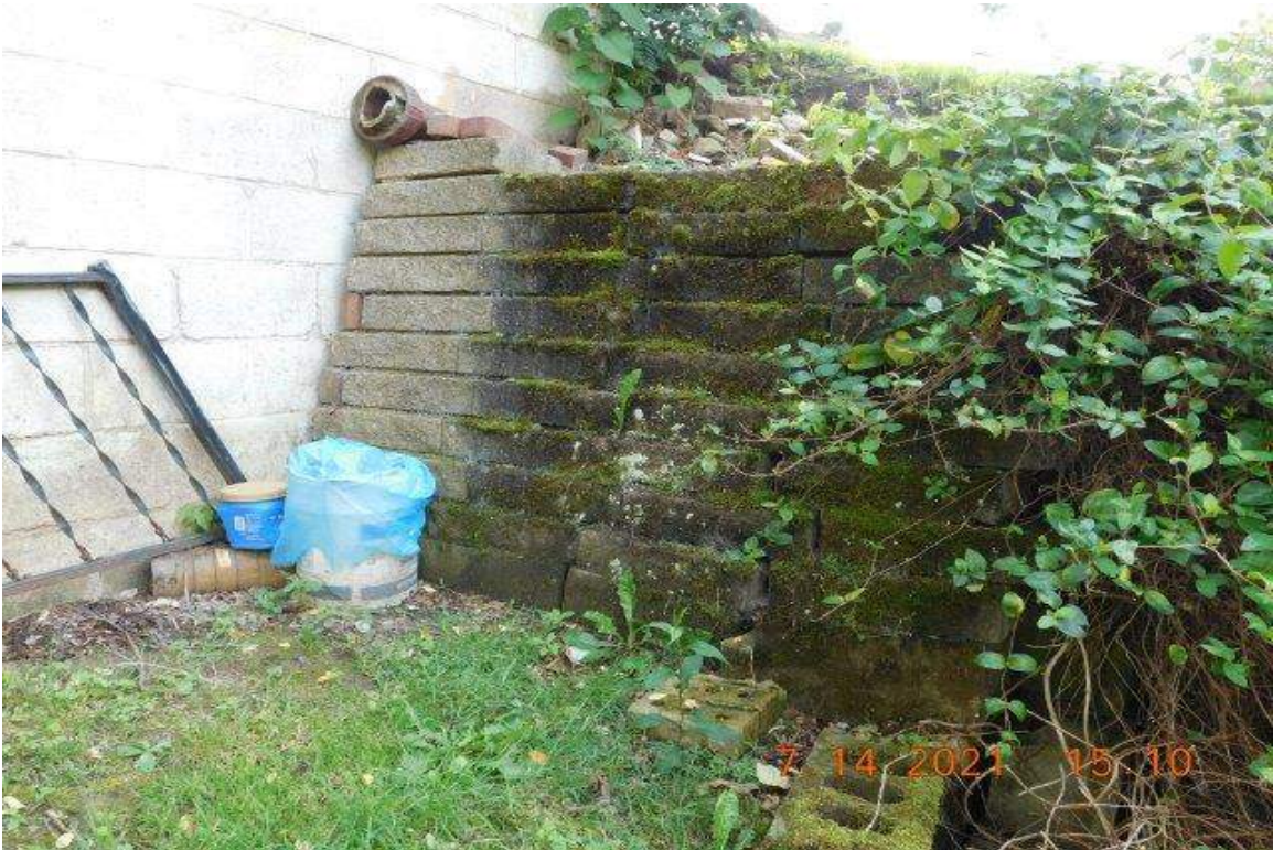
PHOTO 59 - REAR YARD RETAINING WALL ON PROPERTY TO THE EAST
