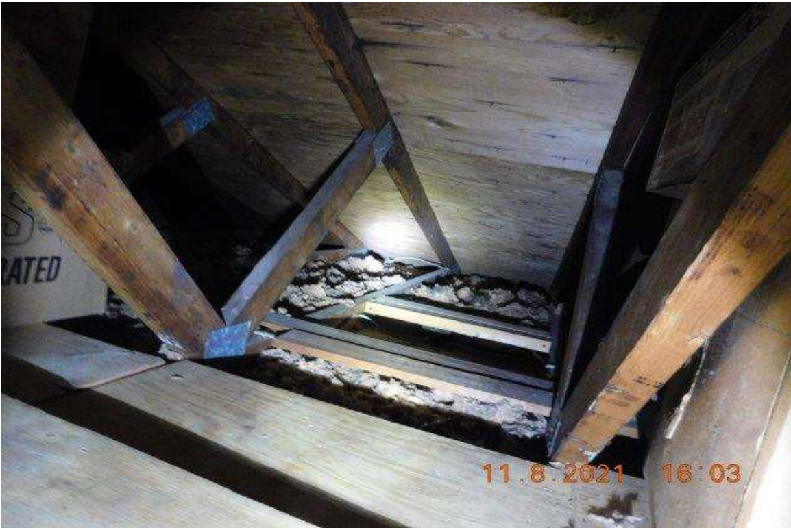
PHOTO 45 - ATTIC ROOF FRAMING
