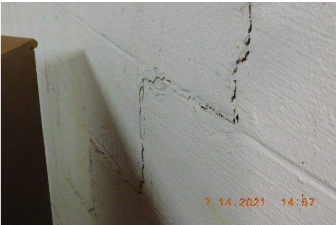
PHOTO 14 - AREA BELOW PHOTO 13
