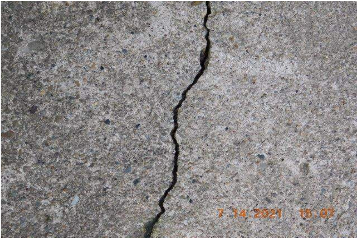
PHOTO 45 - CLOSE-UP OF AREA ON PHOTO 44
