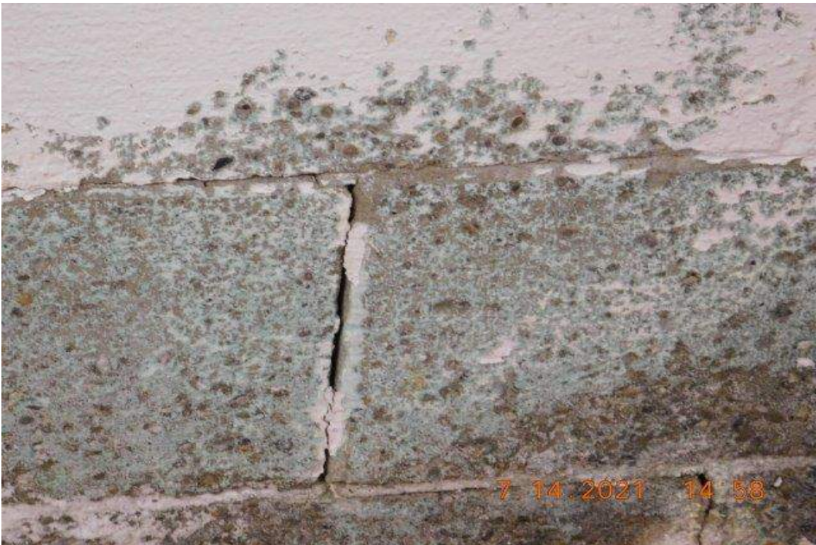
PHOTO 28 - CLOSE-UP OF AREA ON PHOTO 27
