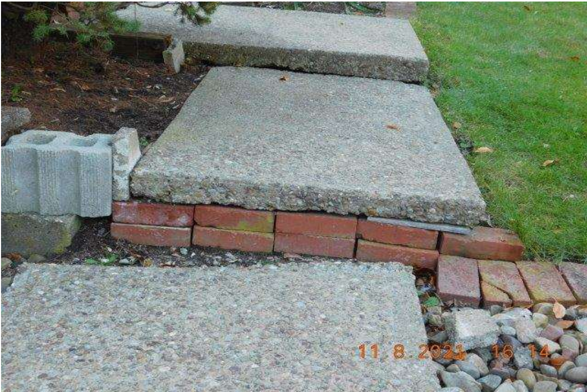
PHOTO 5 - CLOSE-UP OF AREA ON PHOTO 4
