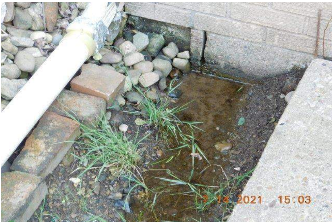
PHOTO 42 - CLOSE-UP OF AREA ON PHOTO 41
