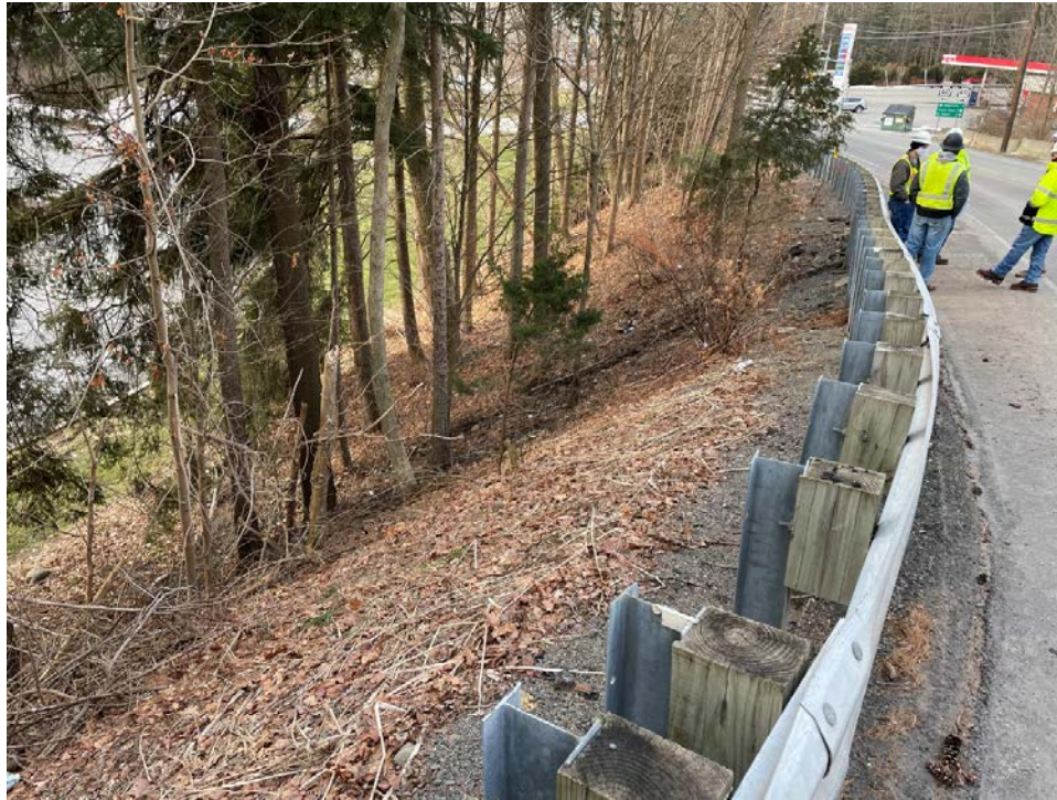
Photo 3 – Slope to South of Gas Release Area
