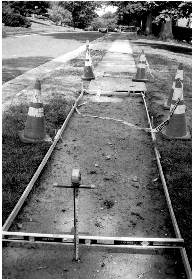
P7 339 PEPPER ROAD - SOIL PROBE DEPTH 27-INCHES BGS LOCATION ID : CENTER OF SLAB LENGTH - STREET SIDE DATE/TIME : 20220613_1112AM_ FOTO ID : P6137596_RS_
