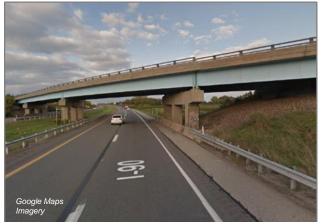
Existing Bort Road bridge profile from eastbound I-90
