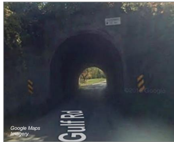
Southbound Gulf Road / CSX Arch approach
