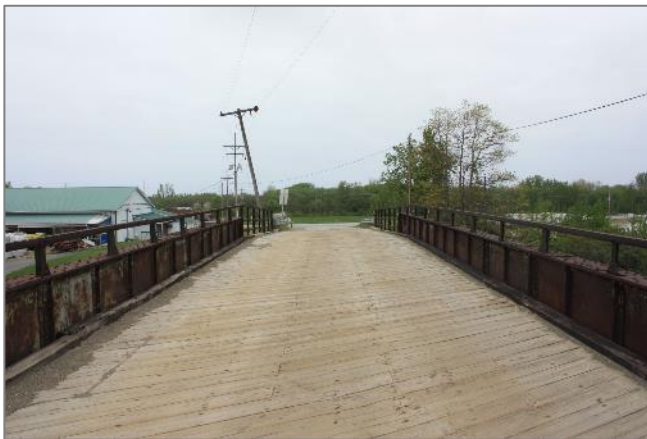
Existing bridge deck/railing
