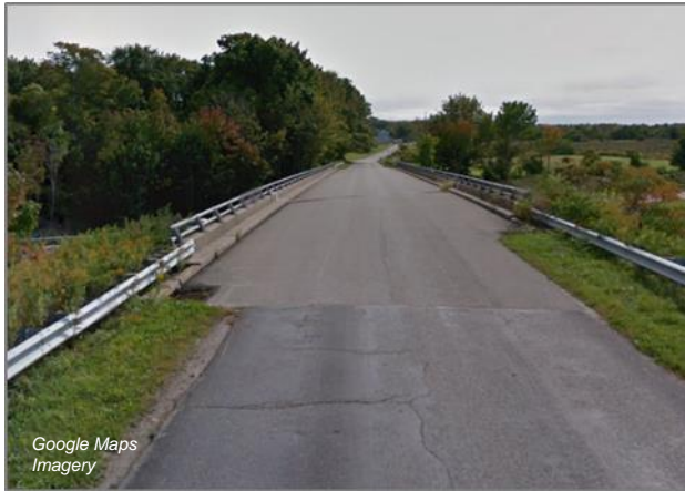
Southbound Remington Road bridge approach over I-90
