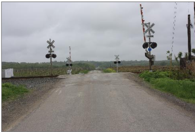
Southbound Remington Road approach to CSX/NS crossing
