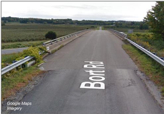
Southbound Bort Road bridge approach over I-90
