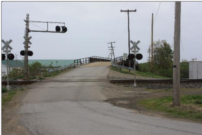
Northbound bridge approach and NS at-grade crossing
