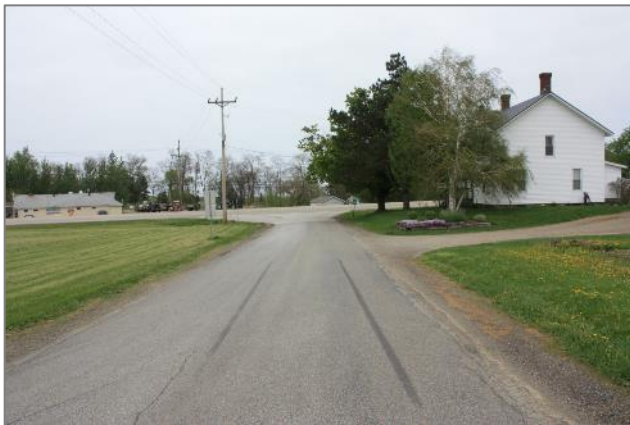
Northbound Remington Road approaching US 20
