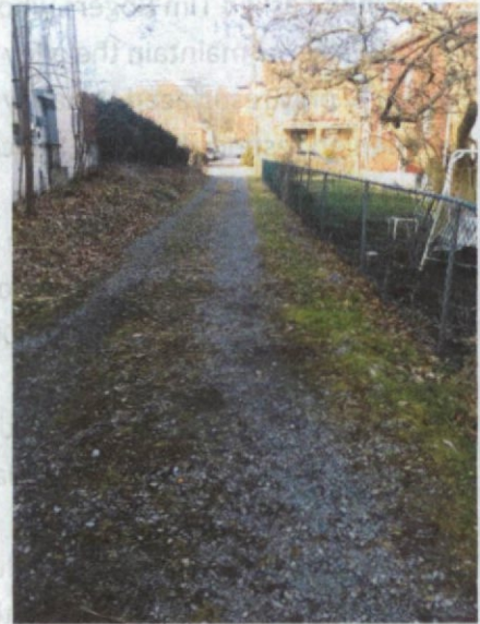
Unpaved section of Argonne Avenue; 103 E Littlewood top right corner ("unmaintained")
