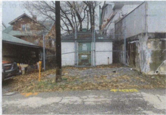
Peoples Gas Substation on Argonne Avenue
