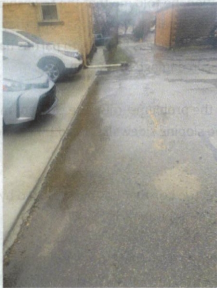
Back and side of 103 E Littlewood along Argonne Avenue ("unmaintained")
