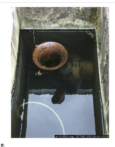
Photo #: 5 DP Discharge Point-001 Description: discharge pipe leading to river from the plant Photo taken by MELISSA L CARVER
