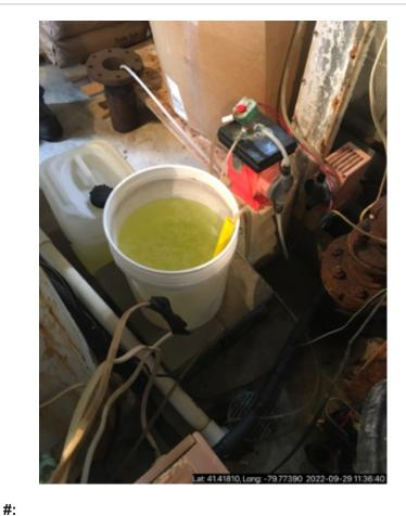
Photo #: 3 TP Treatment Plant-PA0039225 Description: sodium hypochlorite. Bucket Drums stored at office in 55 gallon drums Photo taken by MELISSA L CARVER
