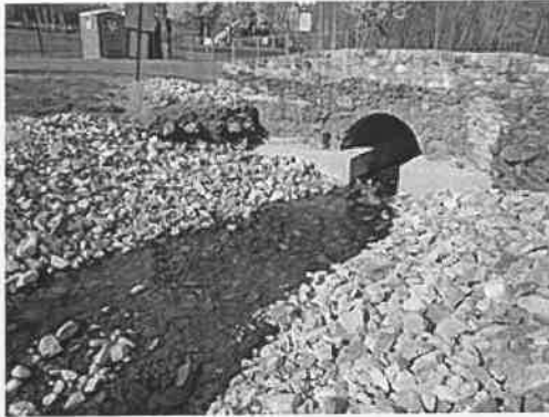
Riprap used to protect a streambank from erosion
