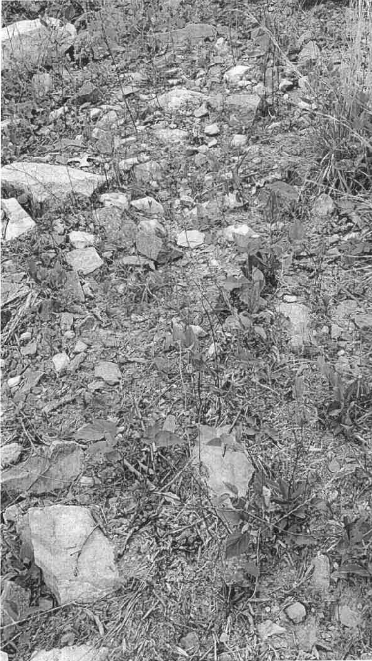
June 6, 2022 Photograph 16 – Access Road Stone that washed off access road onto former vegetated area
