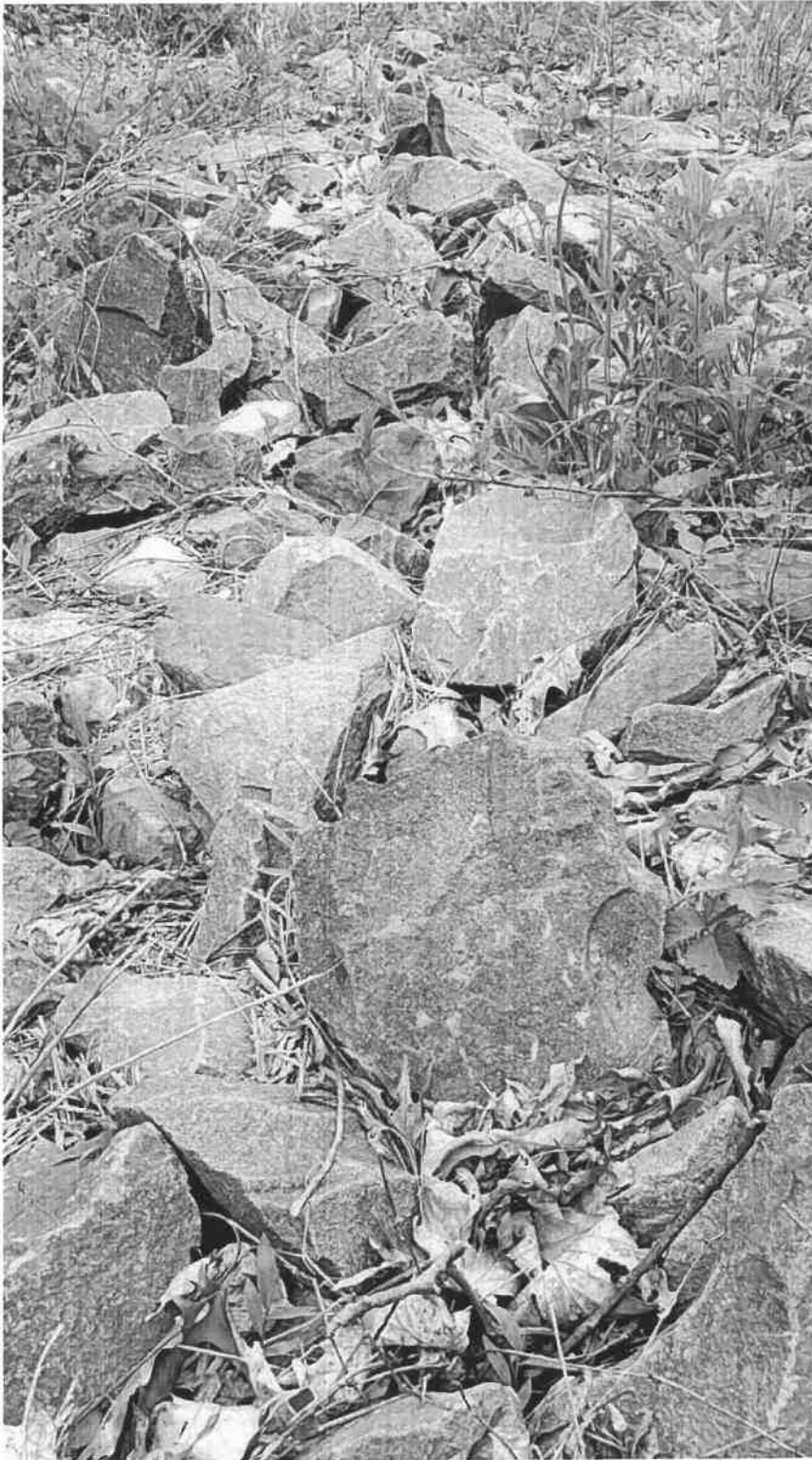
June 6, 2022 Photograph 13 – Sharp Edged Rip Rap soon to be concealed by invasive weeds
