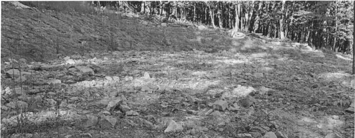
Crane Pad 75 September 21, 2020
