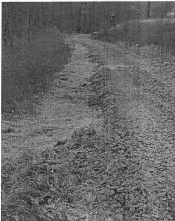
Hartman Pole 76 Access Road Shoulder
