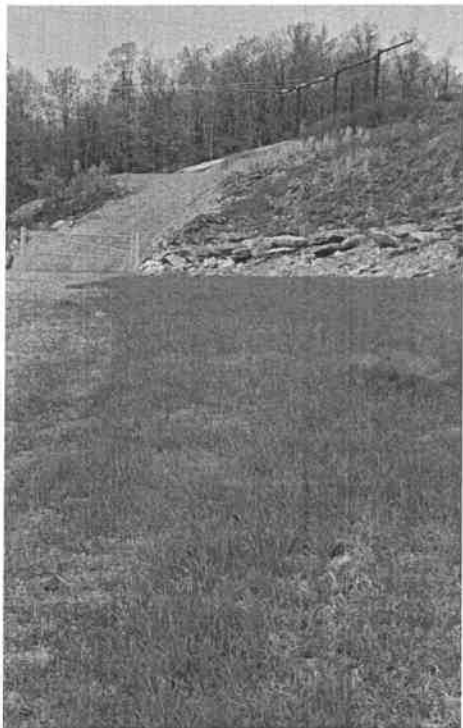
NPS Pole 73 and Pole 74 Access Road Shoulder
