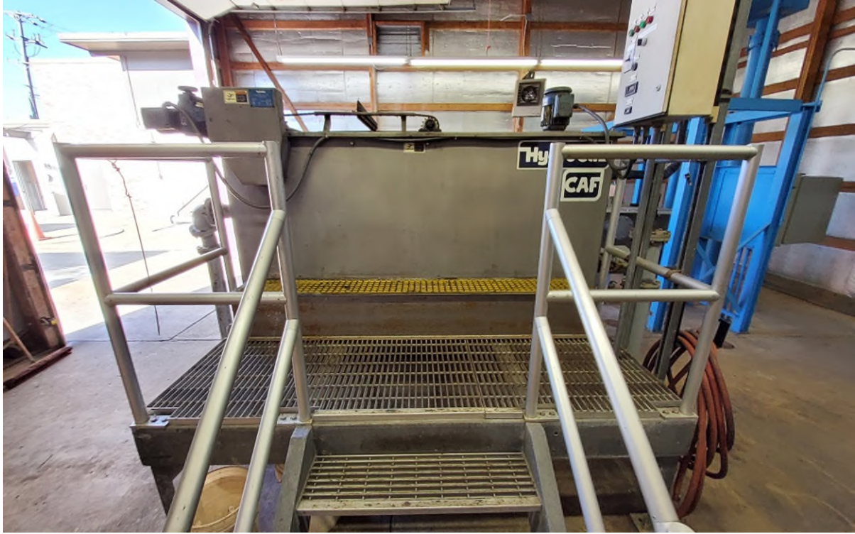
Grease skimmer from North side on concrete floor.
