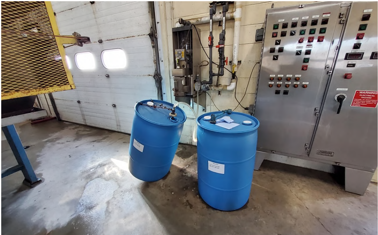
Belt filter press room West wall.
