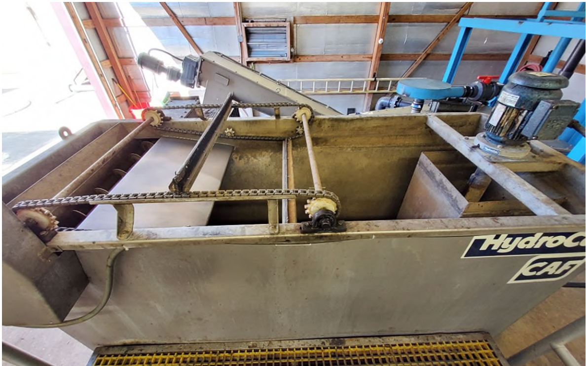
Grease skimmer from platform.
