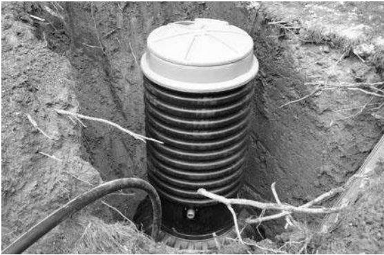
Photo above-Grinder pump station with HDPE tank being installed
