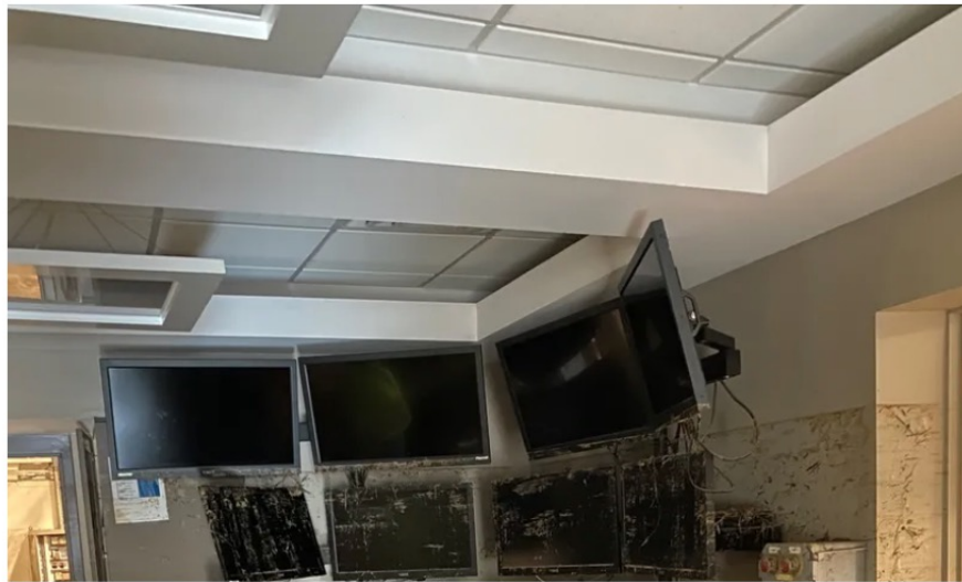
Historic flooding at Aqua's Pickering West water treatment plant damaged the facility's key automated control instrumentation. An Aqua employee points out the high-level water mark. Photo credit Aqua Pennsylvanianormal
