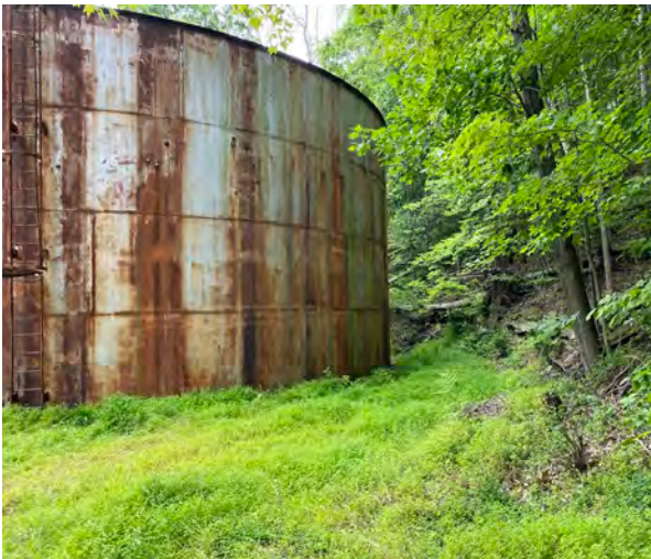
PHOTO #47: View of site.
