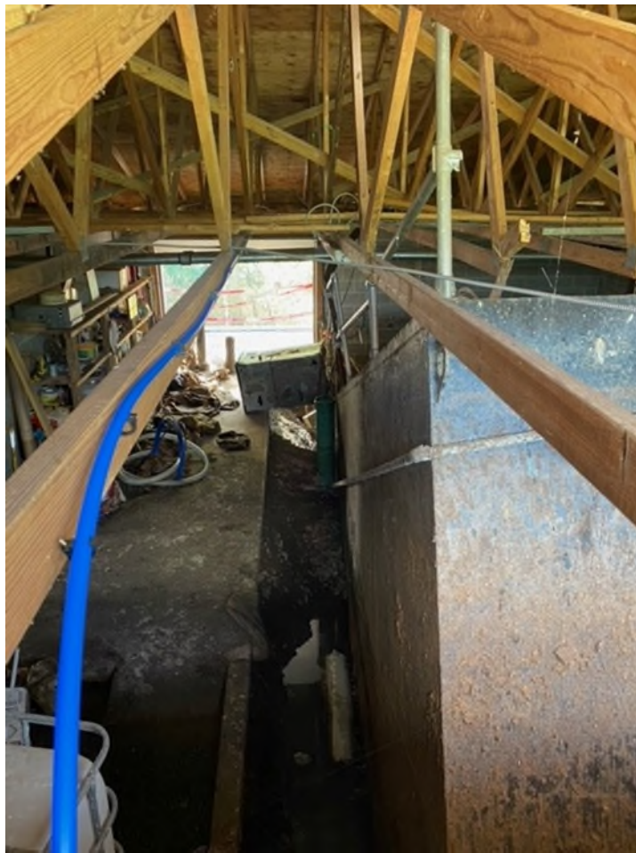
LOOK INSIDE THE CONTROL BLDG. FROM DAMAGED ROOF OPENING. FLOATED TANK IN RIGHT FOREGROUND.
