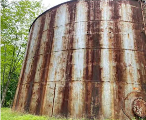
PHOTO #1: Exterior view of the tank.
