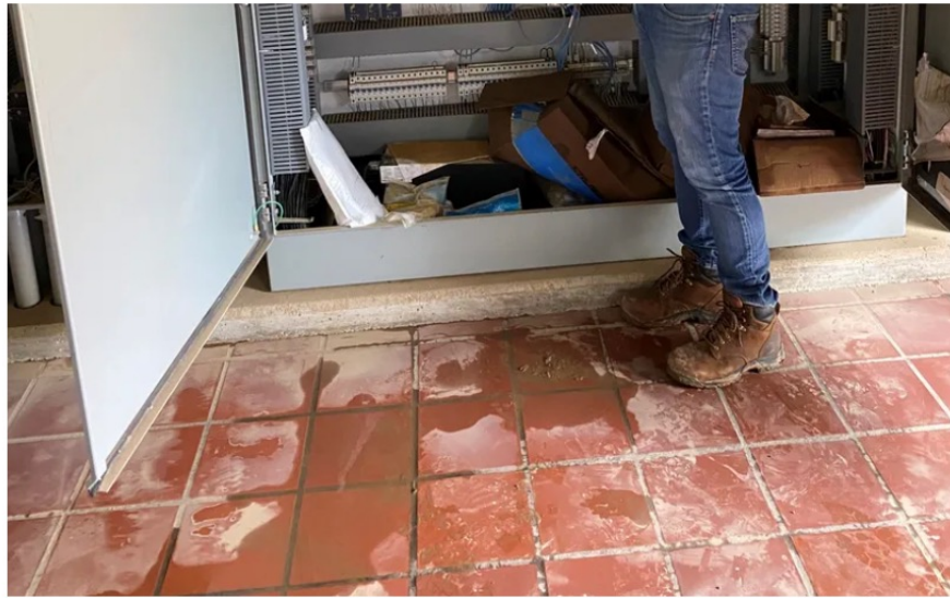
Historic flooding at Aqua's Pickering West water treatment plant damaged the facility's key automated control instrumentation. An Aqua employee points out the high-level water mark. Photo credit Aqua Pennsylvanianormal
