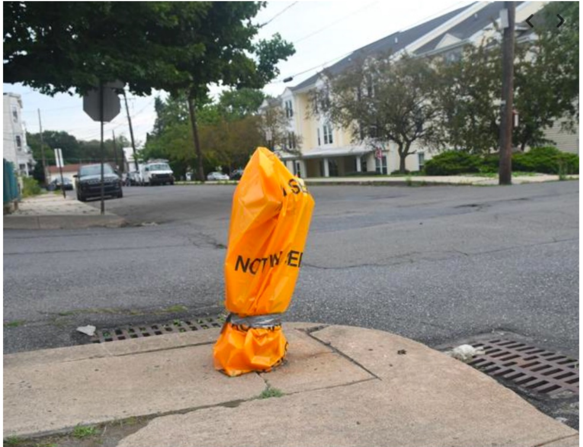
A "Not In Service" bag covers a fire hydrant Monday at East Coal and North Bower streets in Shenandoah.
