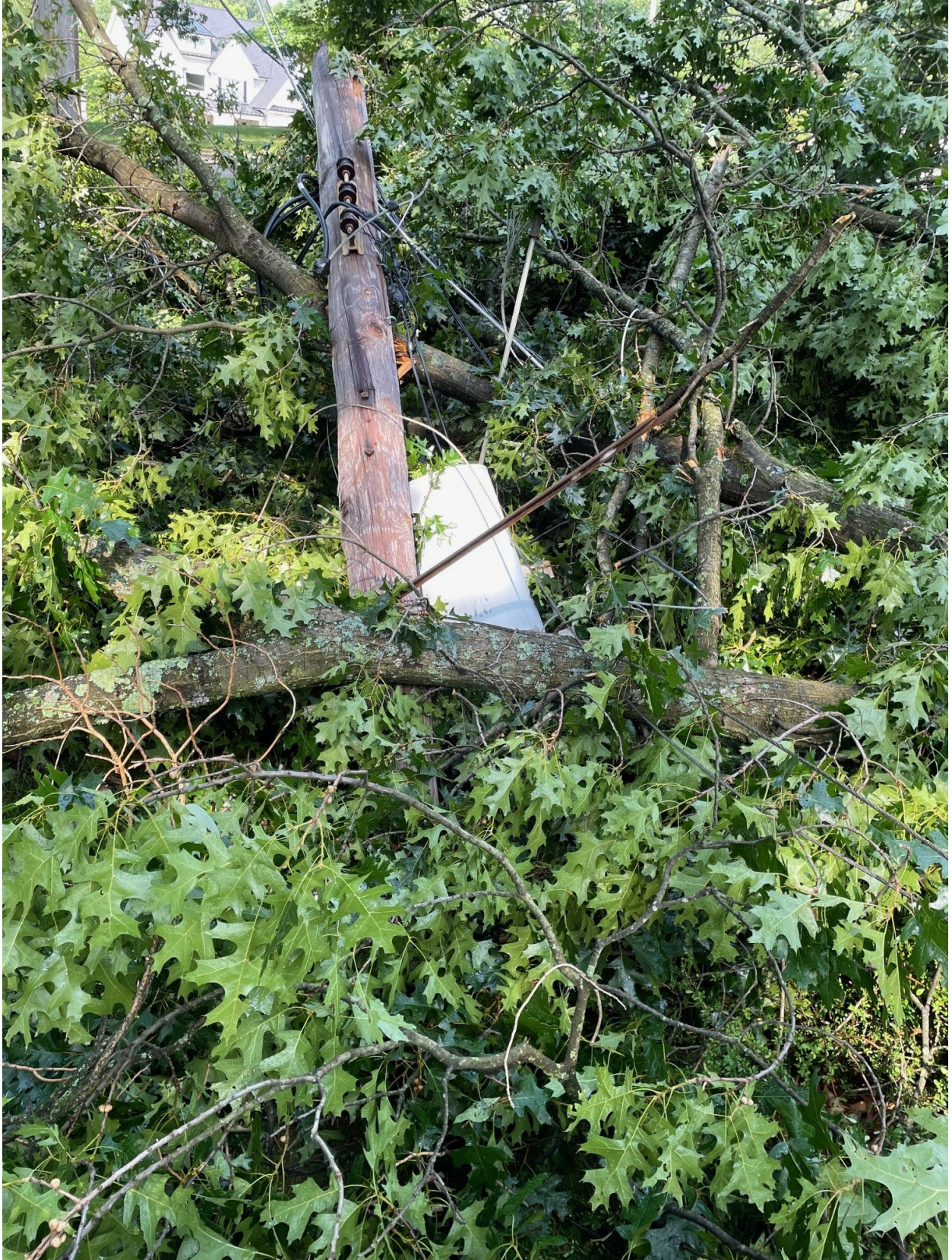
Figure 4: DLC storm photos, Babcock Blvd in McCandless
