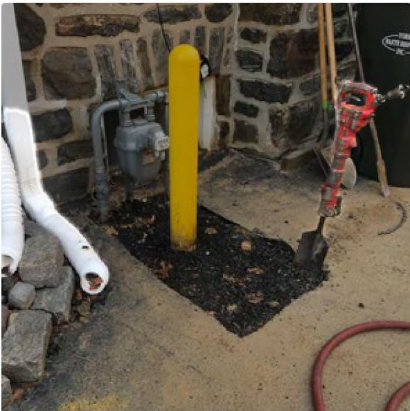
Jackhammer and sinking to replace
