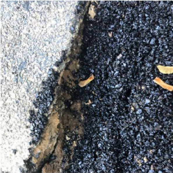
Relocation 1 sinking 3 days
