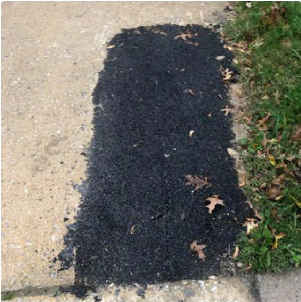
1st pipe access point on driveway
