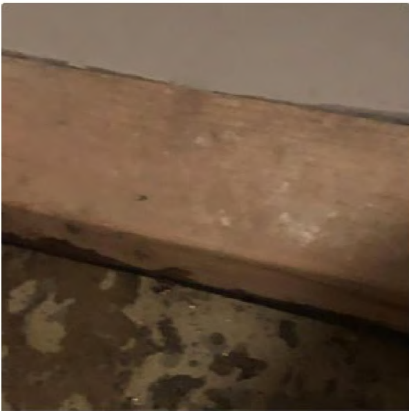
Entry to Sons bedroom louver door from utility room basement
