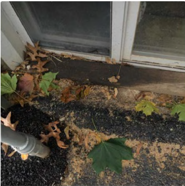
Utility room window
