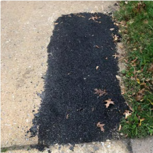
1st pipe access point my property on driveway driveway
