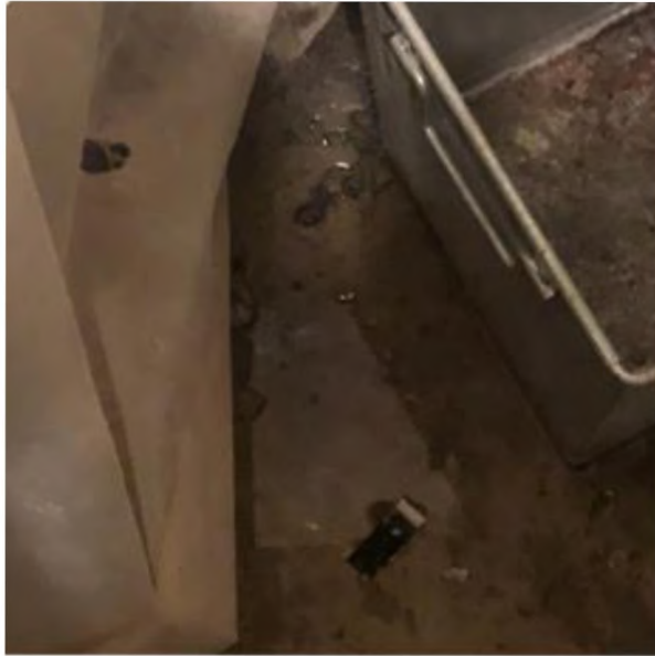
Along chimney floor
