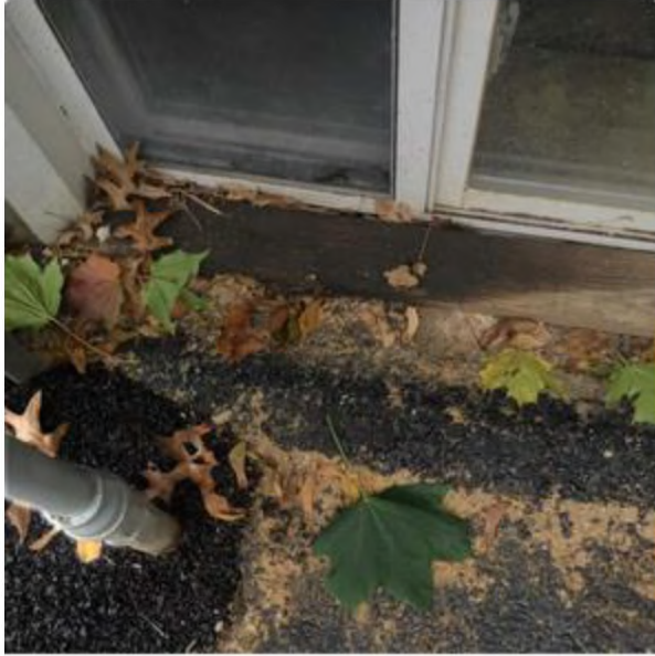
Utility room window
