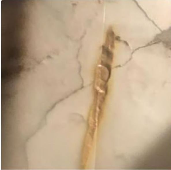
same chimney wall cracking
