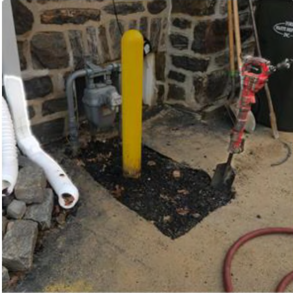
Jackhammer and sinking to replace
