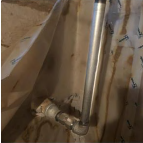
Gas Meter pipe with second sealant applied
