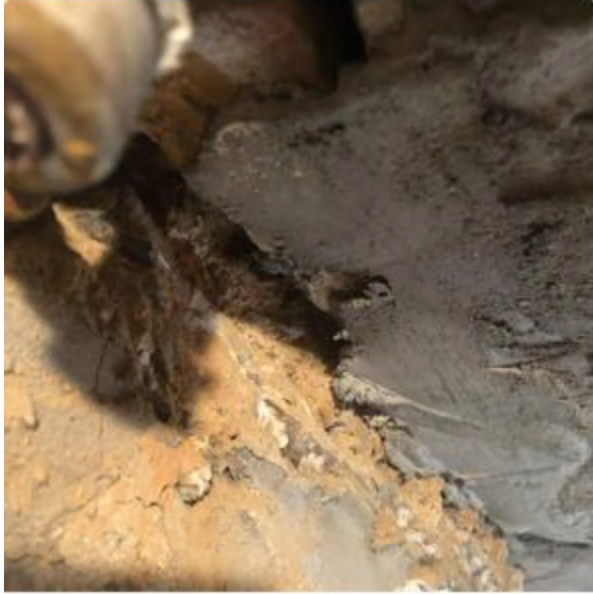
Crack at base of chimney in utility room
