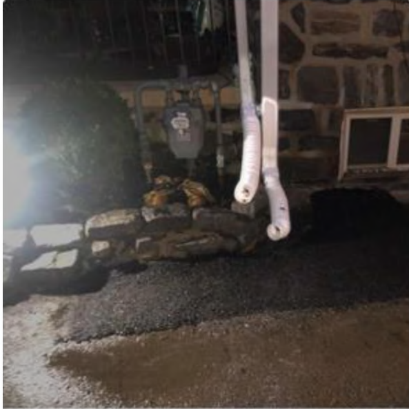
flooding during rain after relocating
