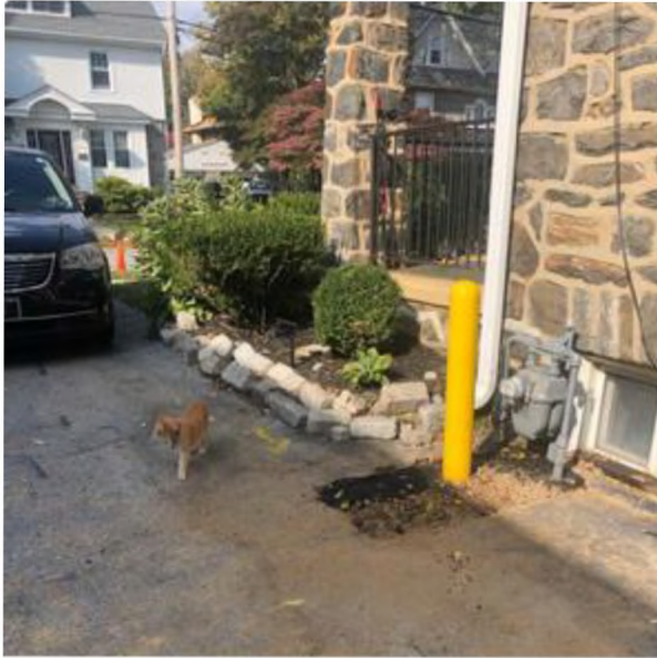
Exhibit 2/70 2nd Access and 1st Relocation of Gas Meter
