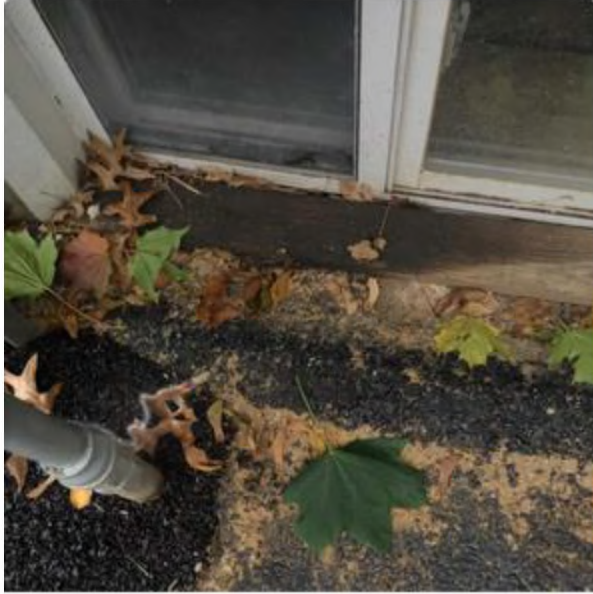
Utility room window
