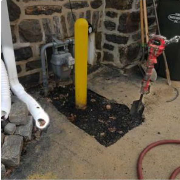
Jackhammer and sinking to refill
