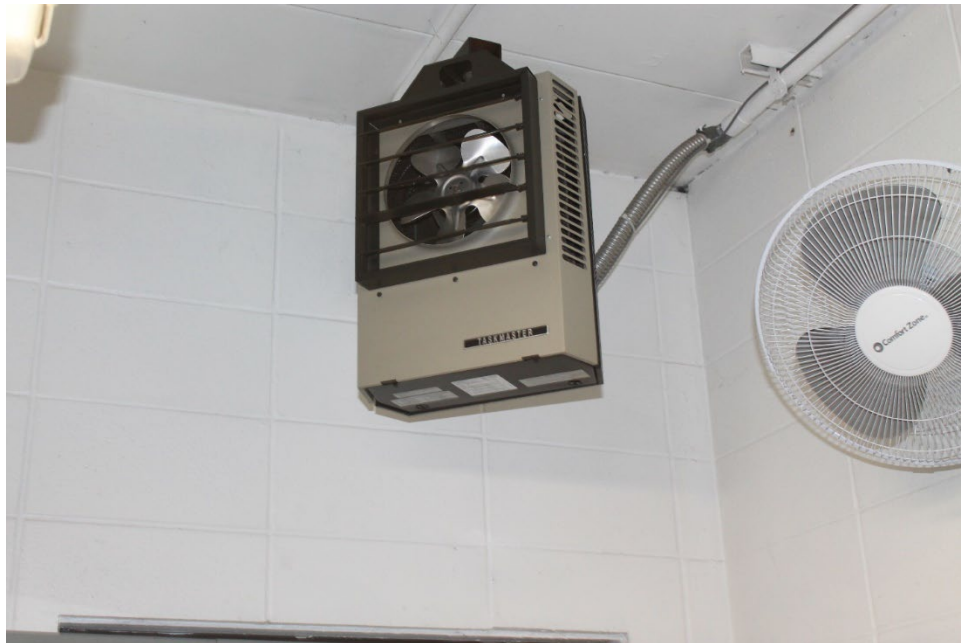
FIGURE 5.3 - 39: ELECTRIC UNIT HEATER-GRIT BUILDING
