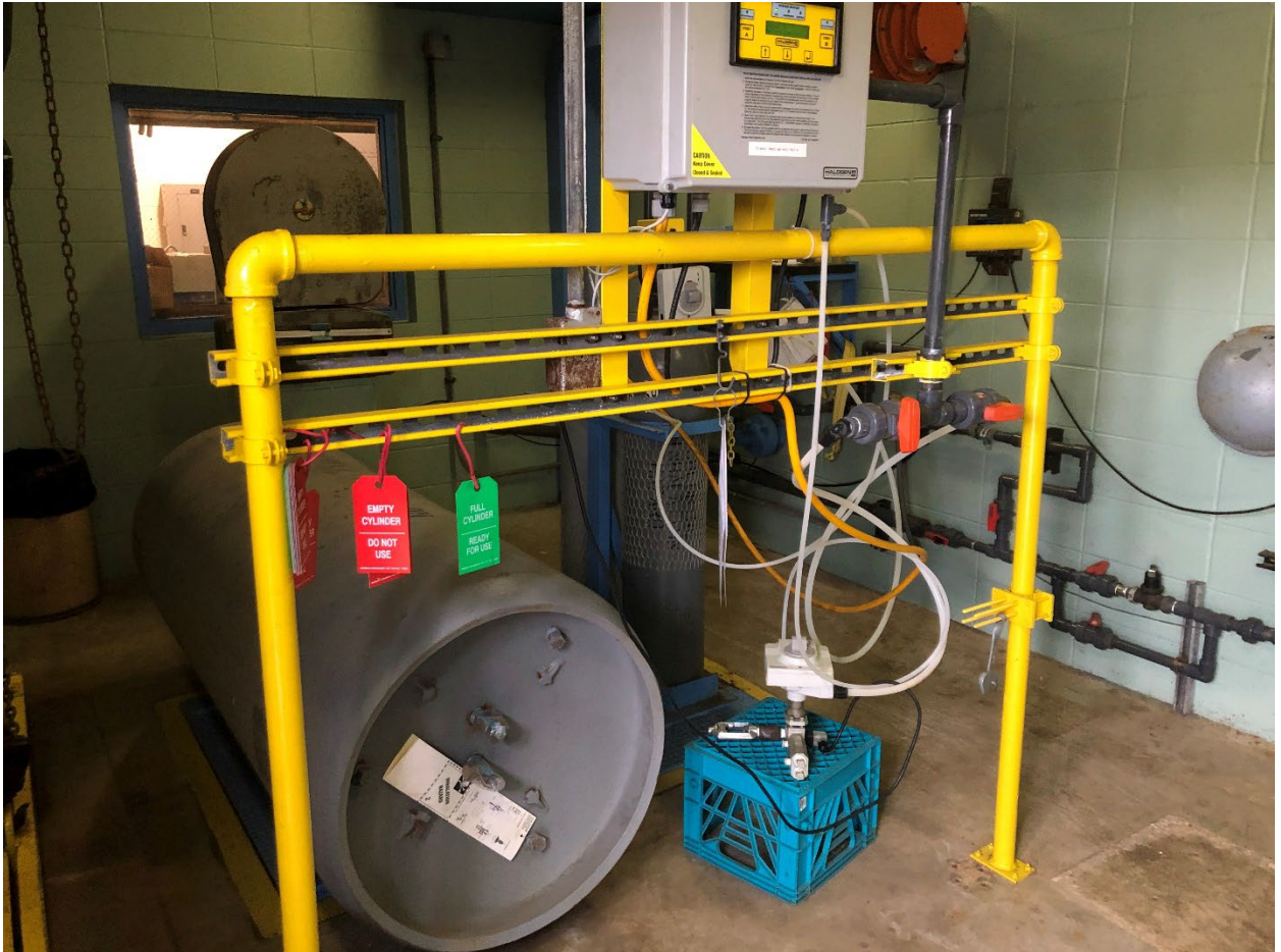
FIGURE 5.3 - 11: CHLORINE SCALES
