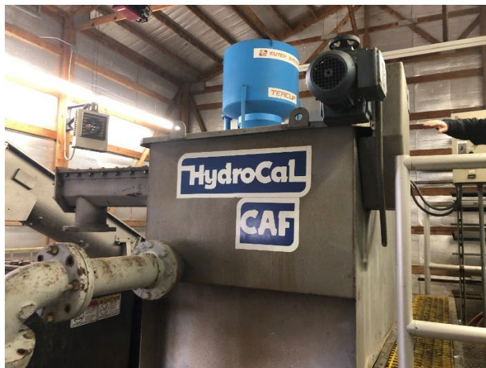
FIGURE 5.3 - 20: GRIT SEPARATOR EQUIPMENT
