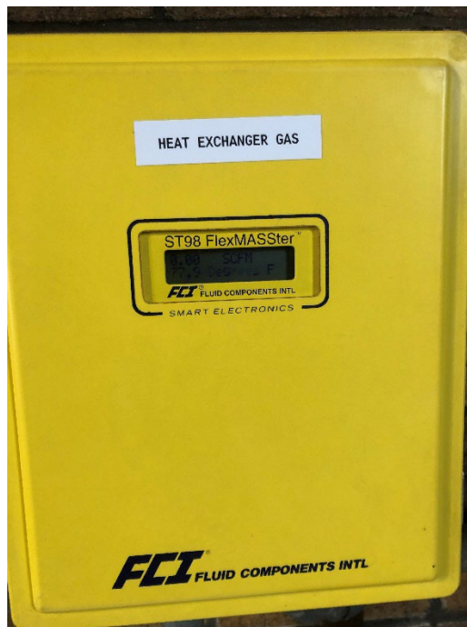
FIGURE 5.3 - 28: ANAEROBIC DIGESTER WASTE GAS METER
