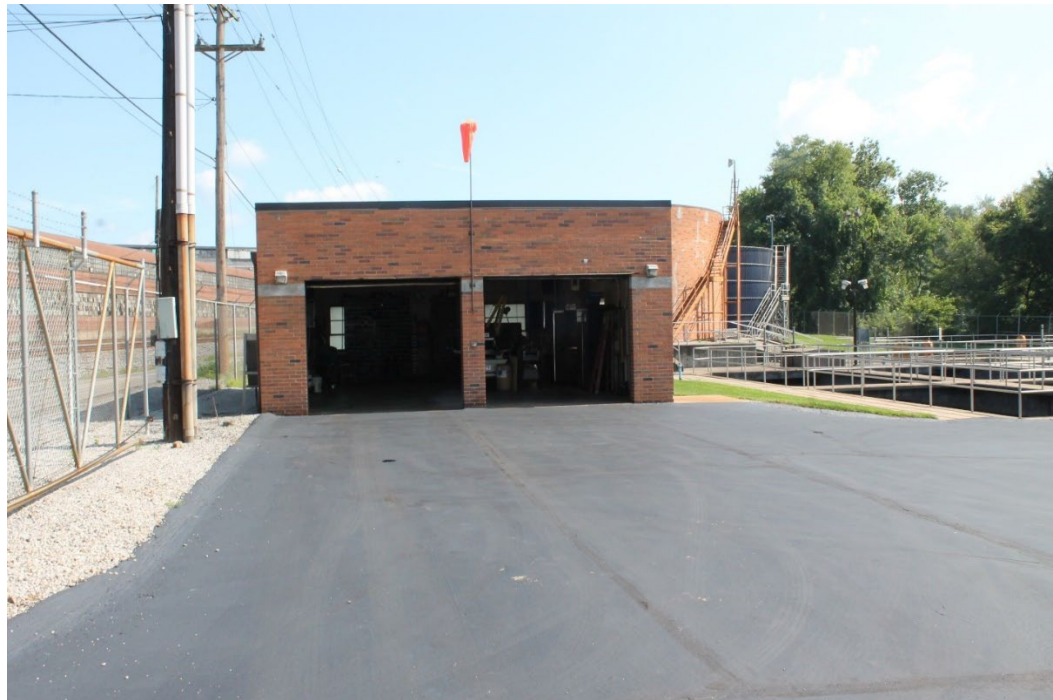
FIGURE 5.3 - 51: MAINTENANCE GARAGE AND TOOL SHOP BUILDING
