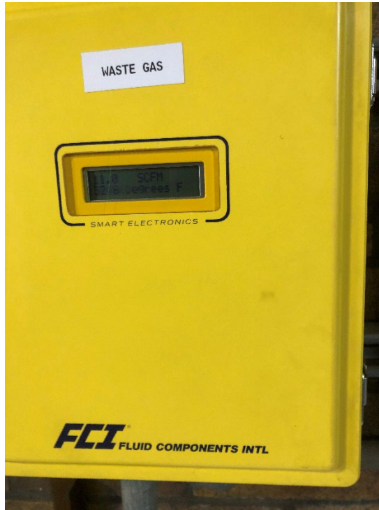
FIGURE 5.3 - 28: ANAEROBIC DIGESTER WASTE GAS METER
