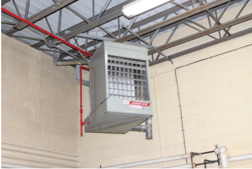
FIGURE 5.3 - 41: GAS FIRED UNIT HEATER GARAGE AREA
