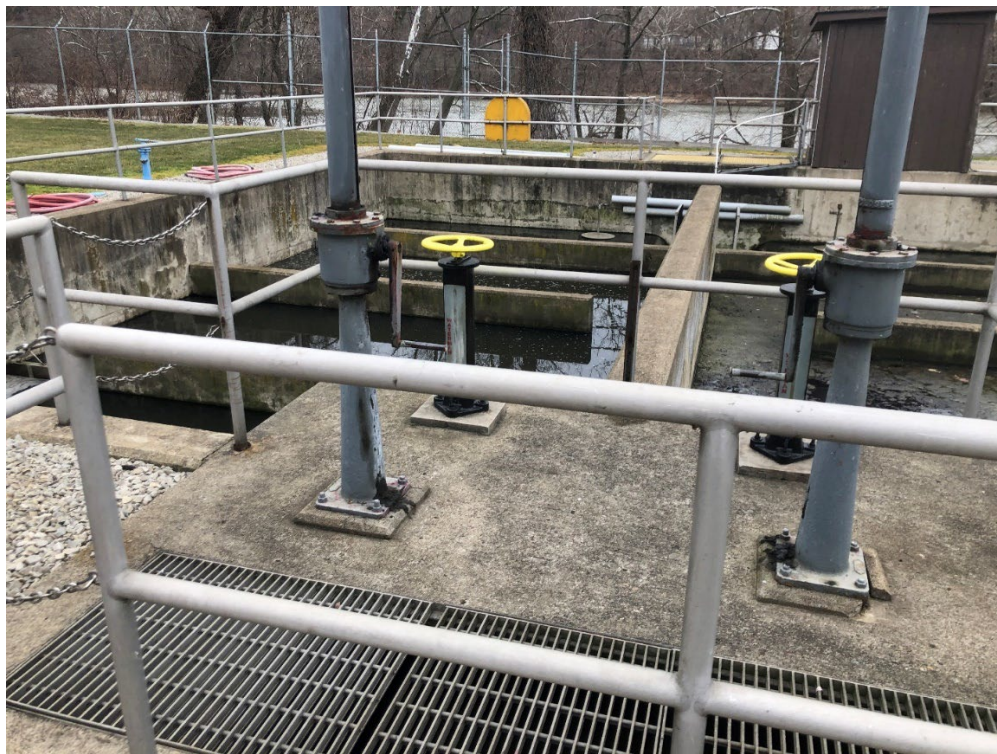
FIGURE 5.3 - 13: CHLORINE CONTACT TANKS-TOP VIEW
