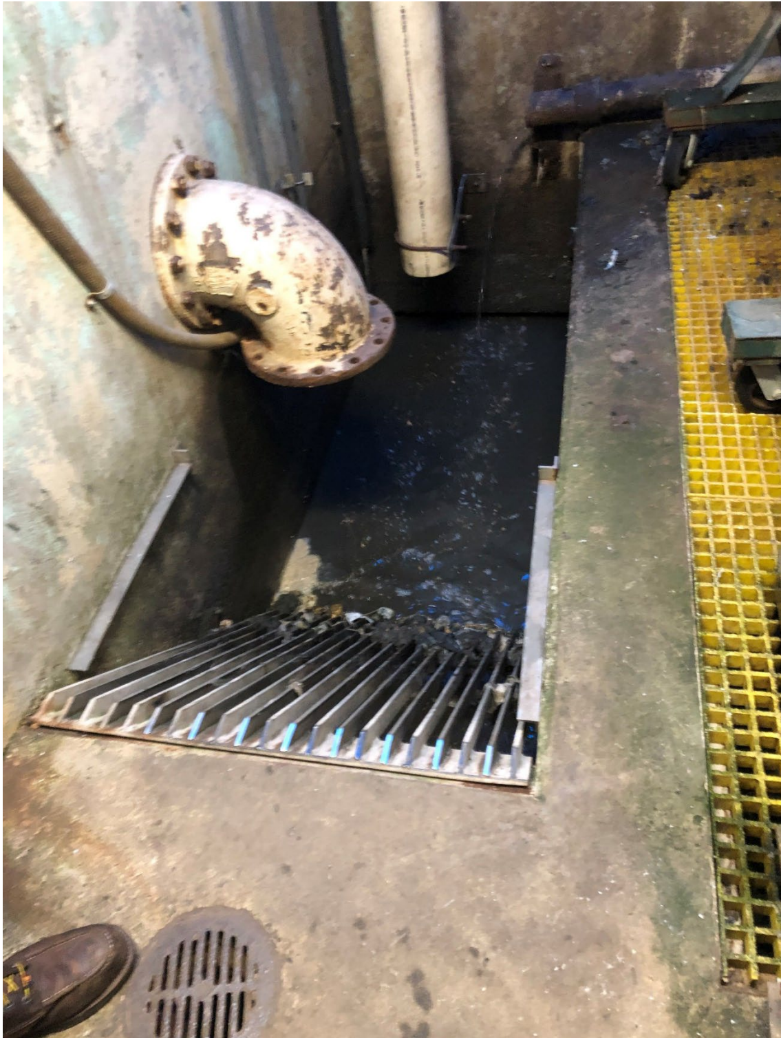
FIGURE 5.3 - 2: MANUAL BAR SCREEN
