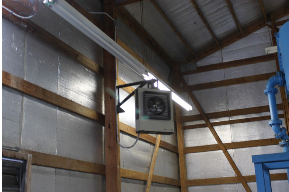
FIGURE 5.3 - 39: ELECTRIC UNIT HEATER-GRIT BUILDING
