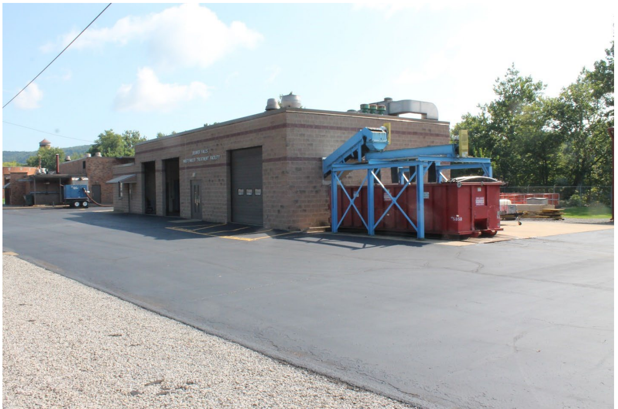
FIGURE 5.3 - 16: SLUDGE DEWATERING BUILDING AND SLUDGE CAKE ROLLOFF BOX
