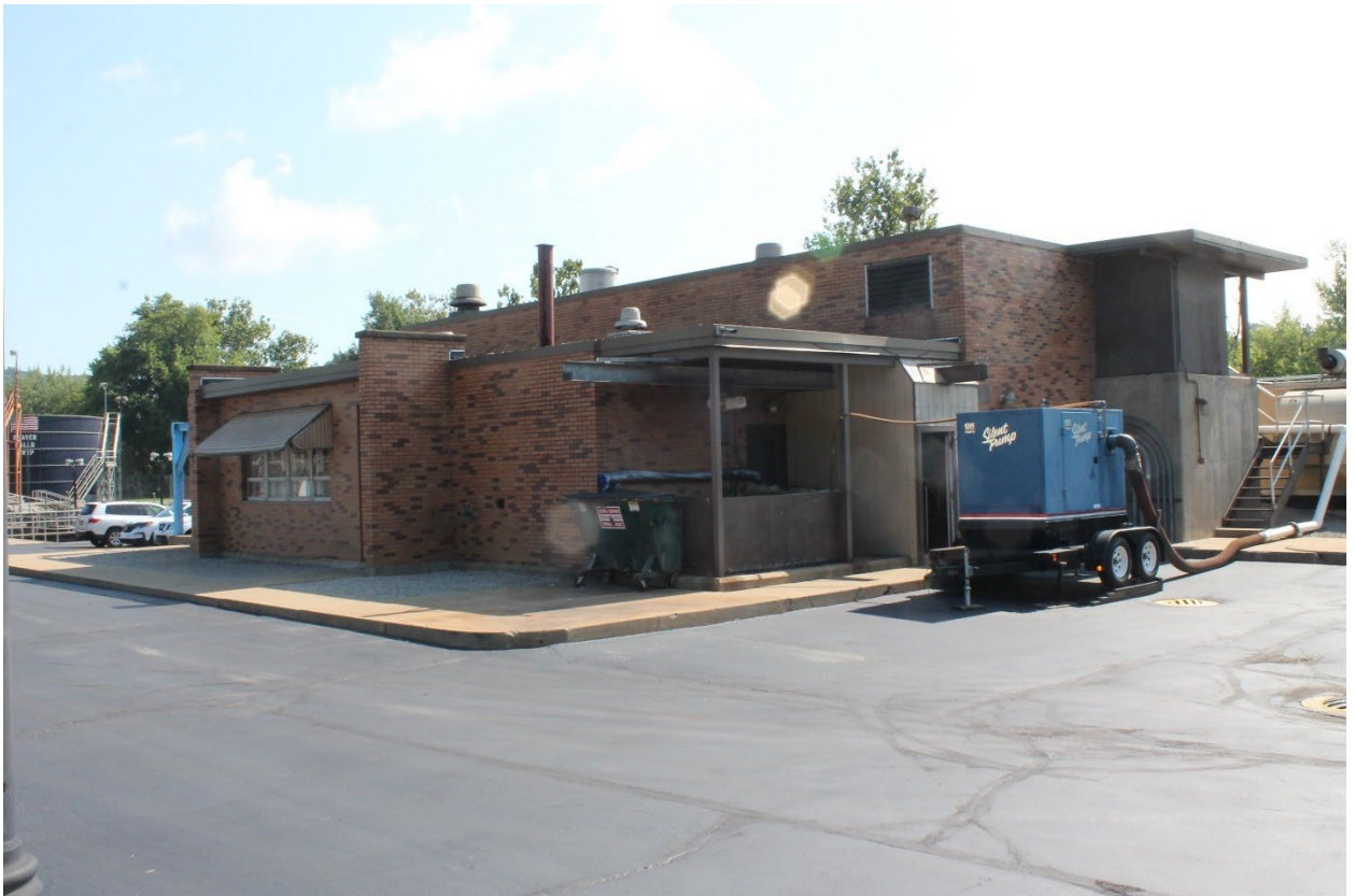
FIGURE 5.3 - 1: HEADWORKS-PRELIMINARY TREATMENT BUILDING
