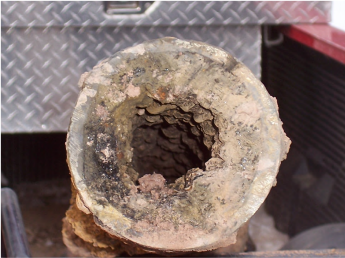
Figure 8 – Replacement of Older Pipes
